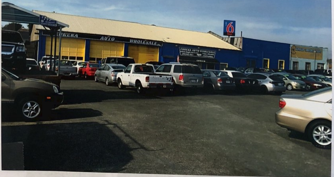
SOUTH WALL (ENDING JUST BELOW MOTEL 6 SIGN)
