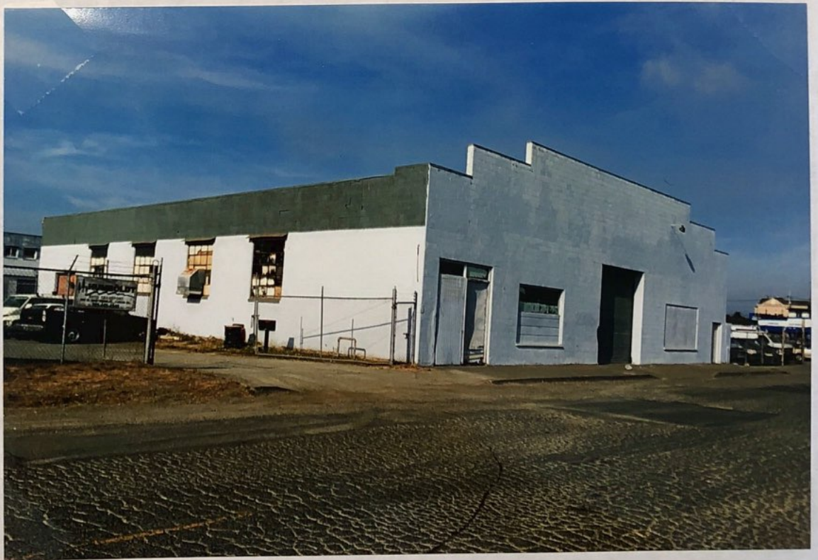
FACADE & WEST WALL
