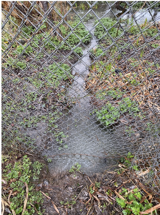
Northern discharge sampling location, D#2. Discharge received from subsurface corrugated pipe receiving runoff from concrete lined ditch and adjacent areas.
