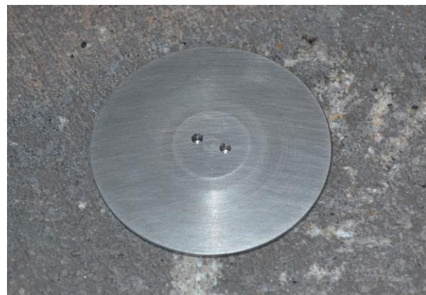
Figure 4. Secure Cover Installed
