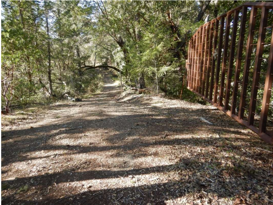
Figure 23: RP 22. Gate. Photo taken facing south-east. (40.0814°, -123.7682°)
