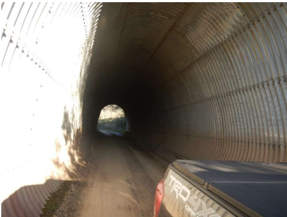
Figure 8: RP 7. Tunnel. Vehicle traveling west. Photo taken facing east. (40.086443°, -123.789988°)
