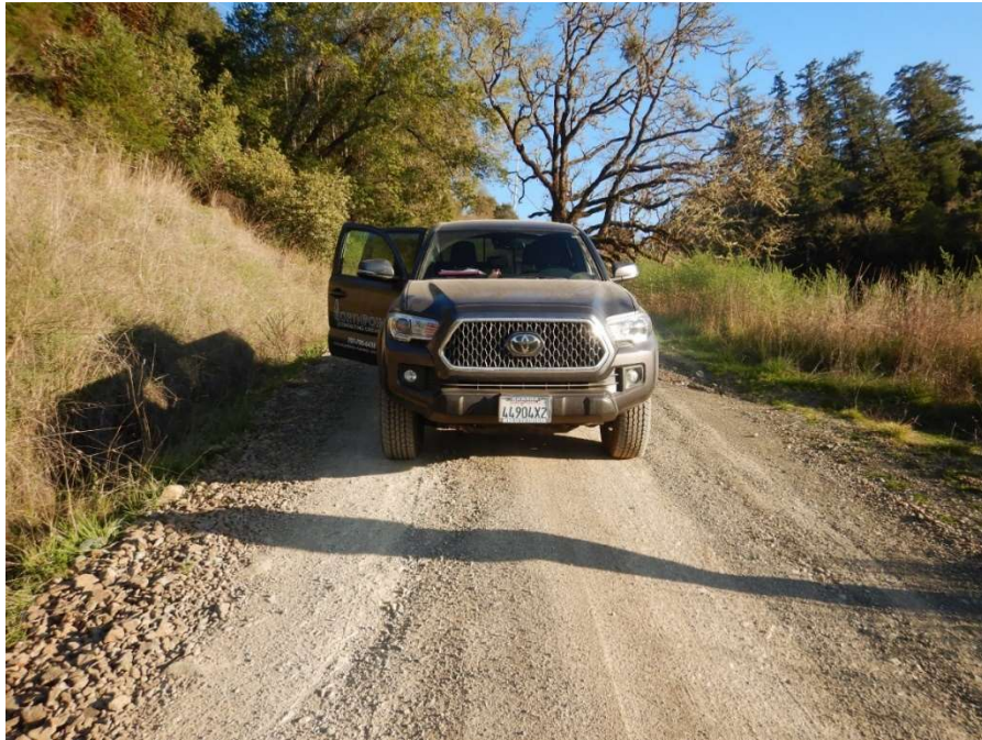
Figure 9: RP 8. Steepest part, 16-ft wide, 22-25% grade for approx. 200' in length. Vehicle traveling north. Photo taken facing south. (40.086675°, -123.788437°)
