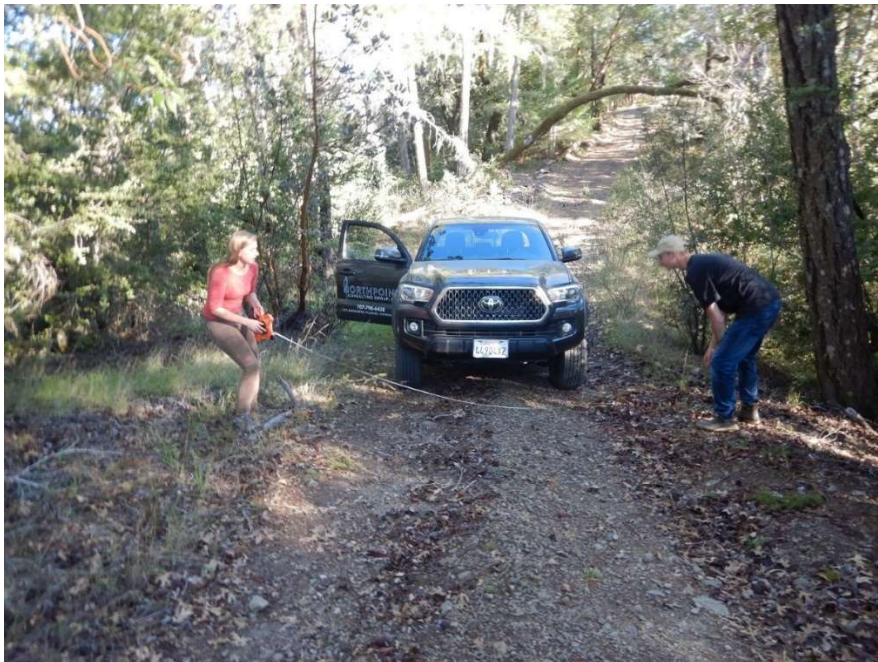
Figure 22: RP 21. Pinch point. Tree in roadway. 11.5-ft wide. No sight distance restrictions. Vehicle traveling north-west. Photo taken facing south-east. (40.082803°, -123.770323°)
