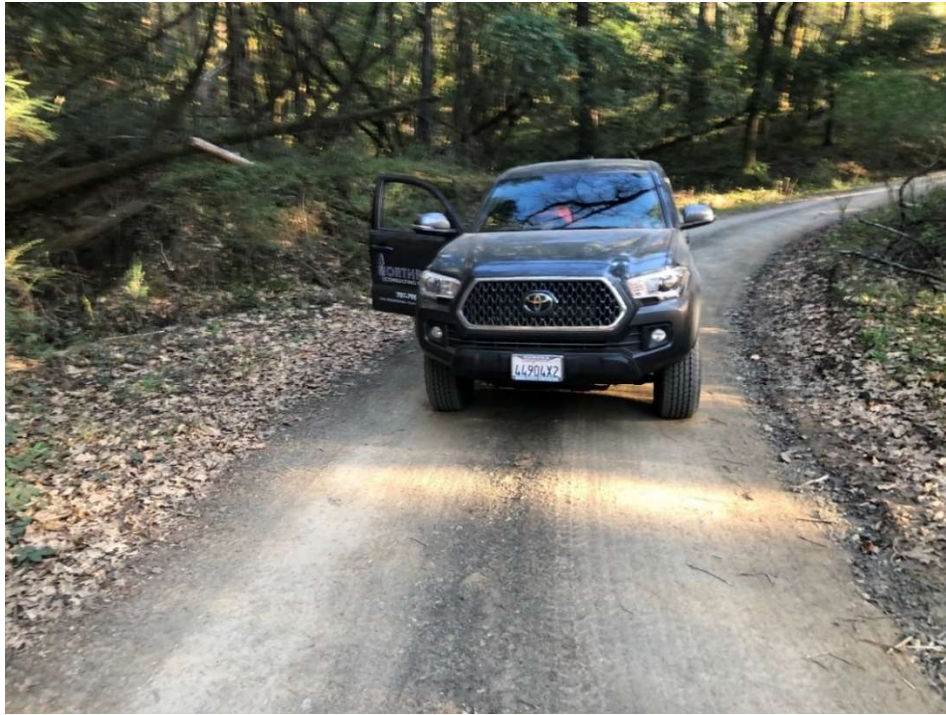
Figure 5: RP 4. Pinch point. Narrow due to STX, 15.5-ft wide. Vehicle traveling north. Photo taken facing south. (40.083967°, -123.793817°)
