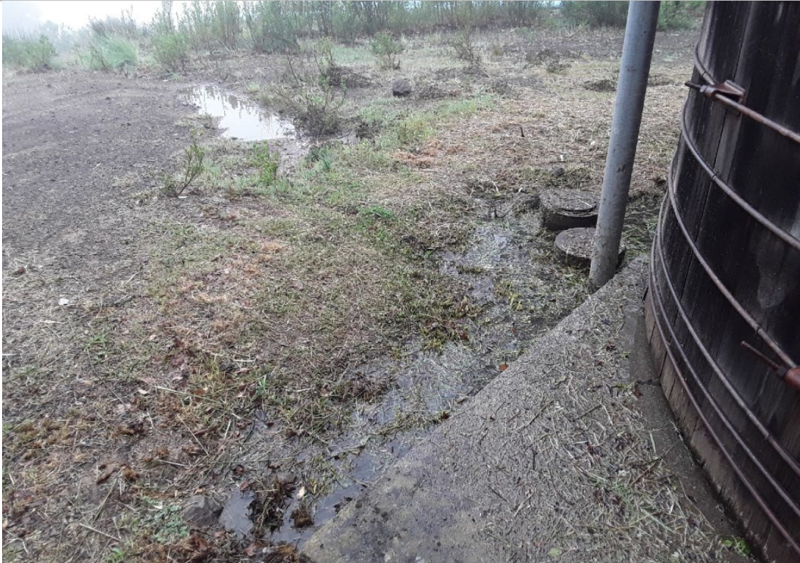
Photo 1: Wallan tank site looking south. Note upland conditions around the tank with pooled water from tank leak. This area was not considered wetland due to the completely artificial conditions and lack of hydrophytes and hydric soils. Photo taken April 19, 2022.
