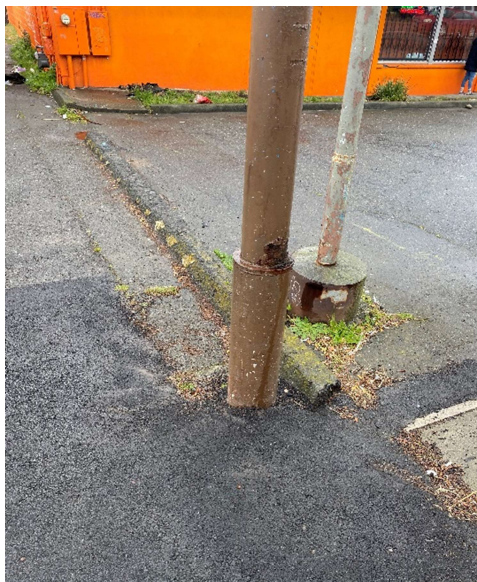
Figure 1. Existing berm between Mr. Fish (on left) and Discount Cigarettes (on right).
