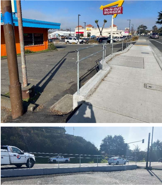
Figure 6: Recently-Constructed Sidewalk Adjacent to the Project Site
