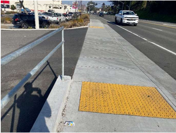
Figure 7: Recently Reconstructed Driveway Access for the Project Site
