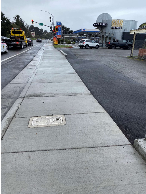
Figure 2. New sidewalk in front of 2740 Broadway (Mr. Fish).
