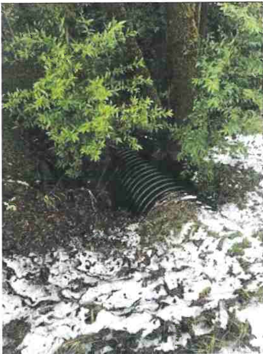
Stream Crossing Culvert near decommissioned greenhouses
