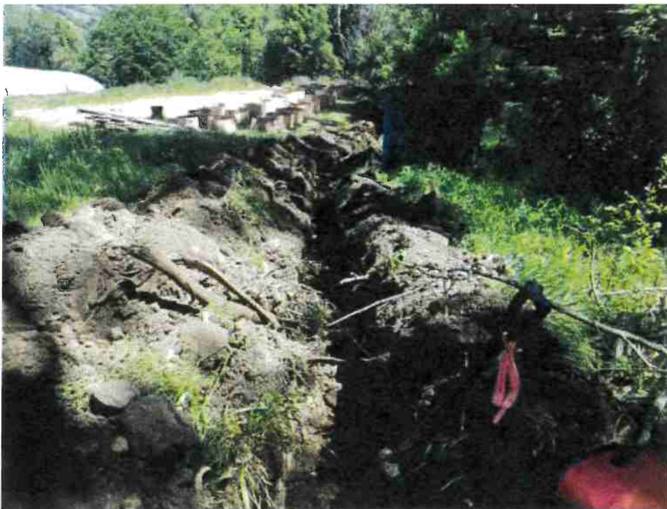
Photo 14. Looking east at Plot 8 in trench, at shovel. April 2021
