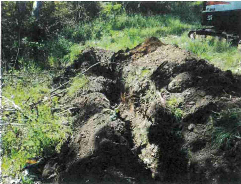
Photo 13. Looking west towards Plot 8, which is in trench. April 2021
