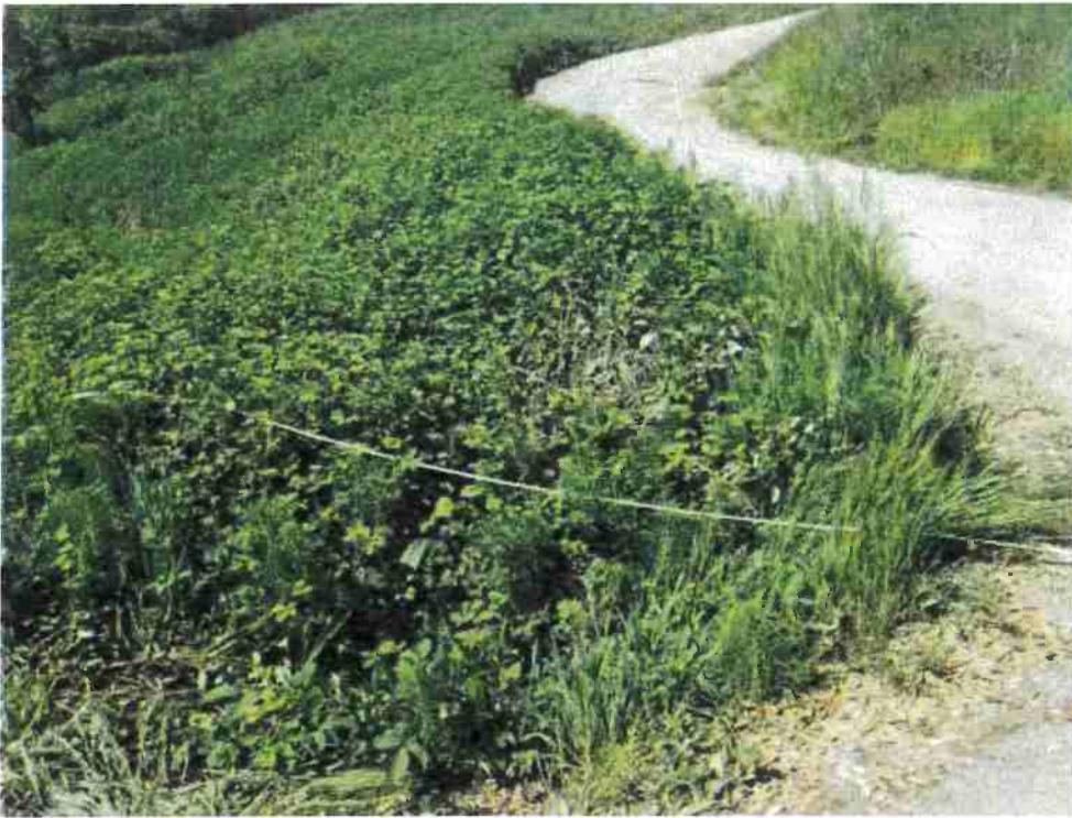
Photo 9. Looking West towards Plot 6. April 2021
