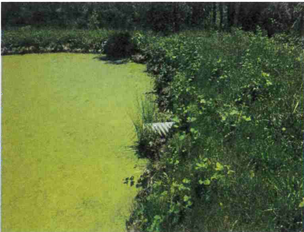
Photo 4. Looking east across pond outlet culvert. April 2021
