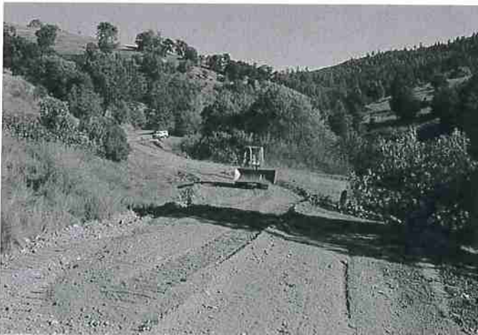
Figure 31. Bulldozer reshaping road surface to out-sloped condition to improve drainage. Photo: Jared Gerstein.
