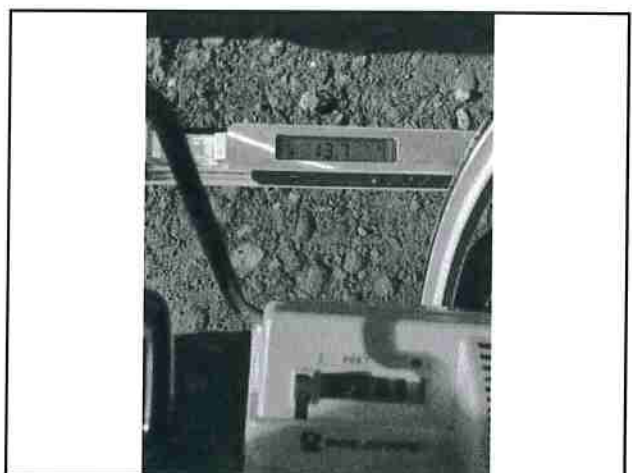
Photo #36 Cobb Rd Slope 13.7' Width 15'11"
