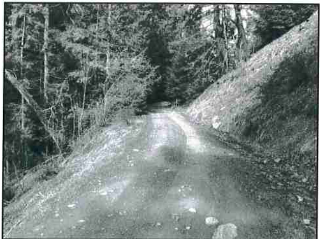
Photo #12 Cobb Rd @ Pullout Looking NW
