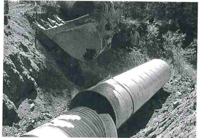
Figure 30. Installation of a new culvert after the old one was excavated. Photo: Jared Gerstein.
