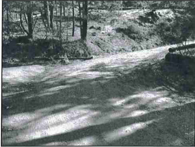
Photo #37 Cobb Rd @ Curve w/ Pullout Looking NE
