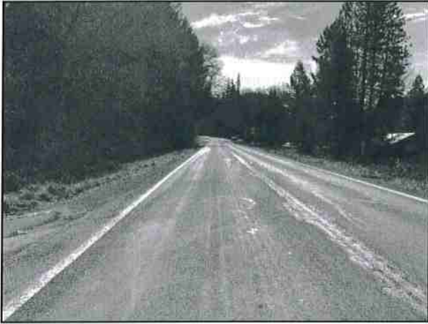
Photo #43 Cobb Rd & Highway 36 Looking East
