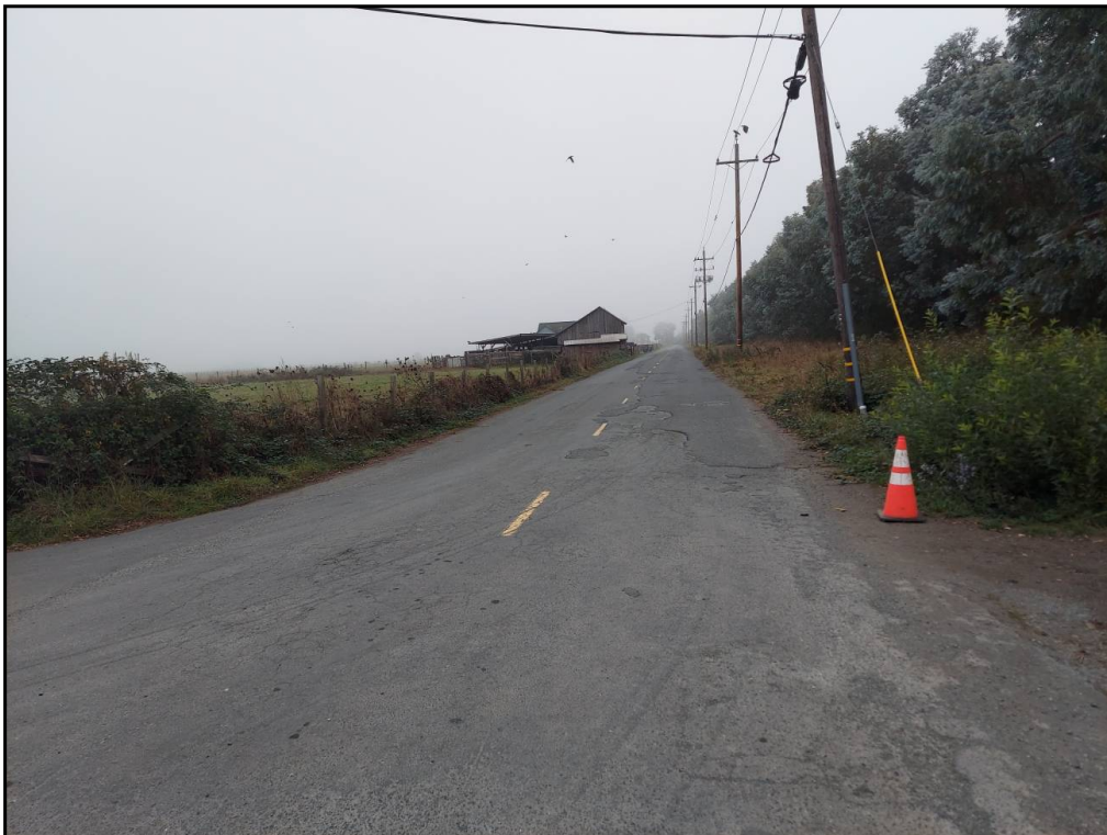
10 : View down Foster Avenue, facing northwest.
