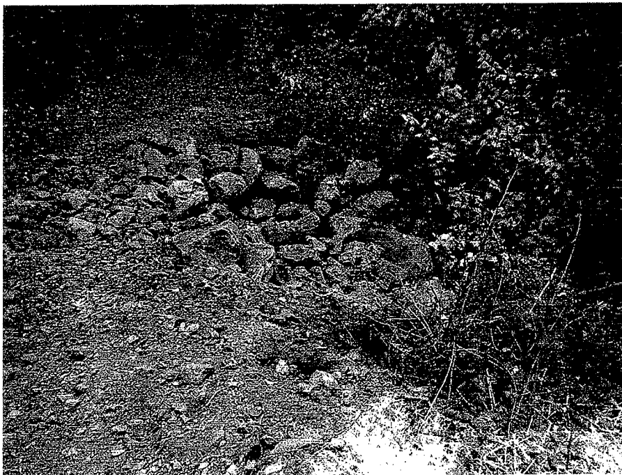
Photo 1D - SC #1: View looking at the armored fillslope crossing from the right outboard edge of the road (Photo 11/5/2020).
