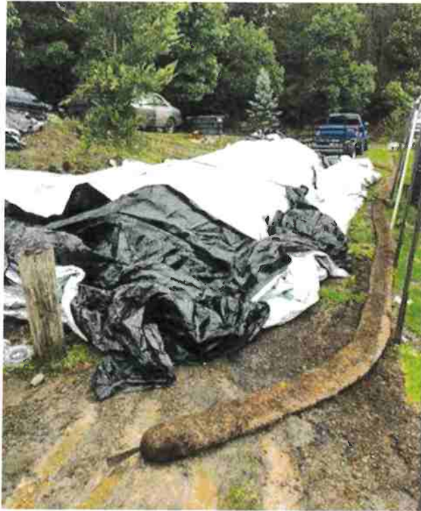
Photo 5. Spoils pile next to nursery – 1/14/19
