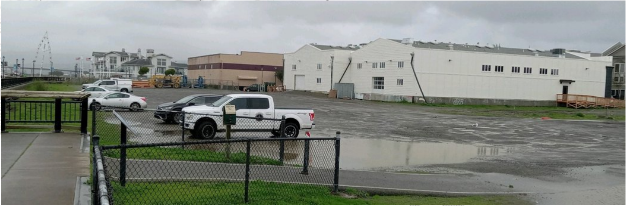
Site City-13: #1 E Street (Street view from Boardwalk looking southeast)
