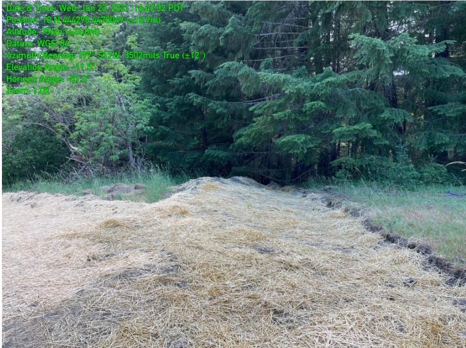
9.0 Mulched Area of Disturbed Soils
