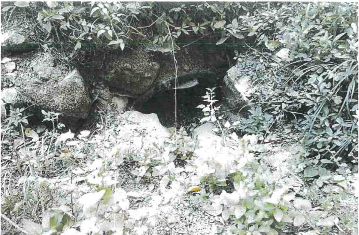
Photo looking at the inlet of the culvert at Site 07.
