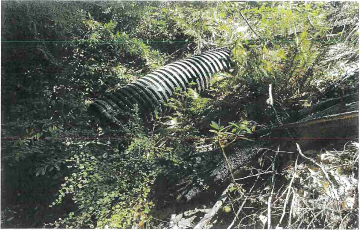
Photo looking at the outlet of the culvert at Site 05.
