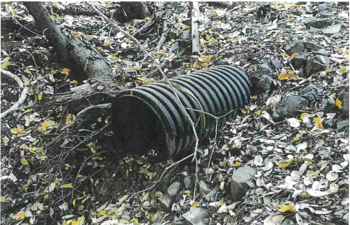
Photo looking at the outlet of the culvert at Site 07.
