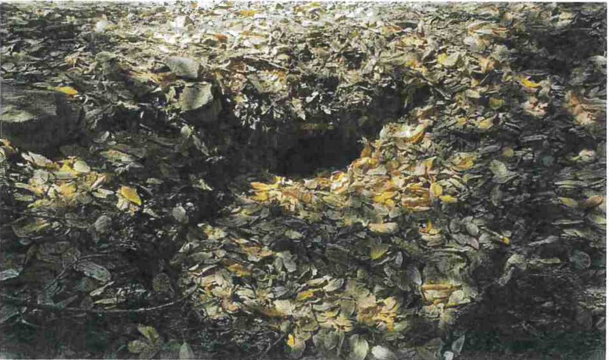
Photo looking at the inlet of the culvert at Site 04.
