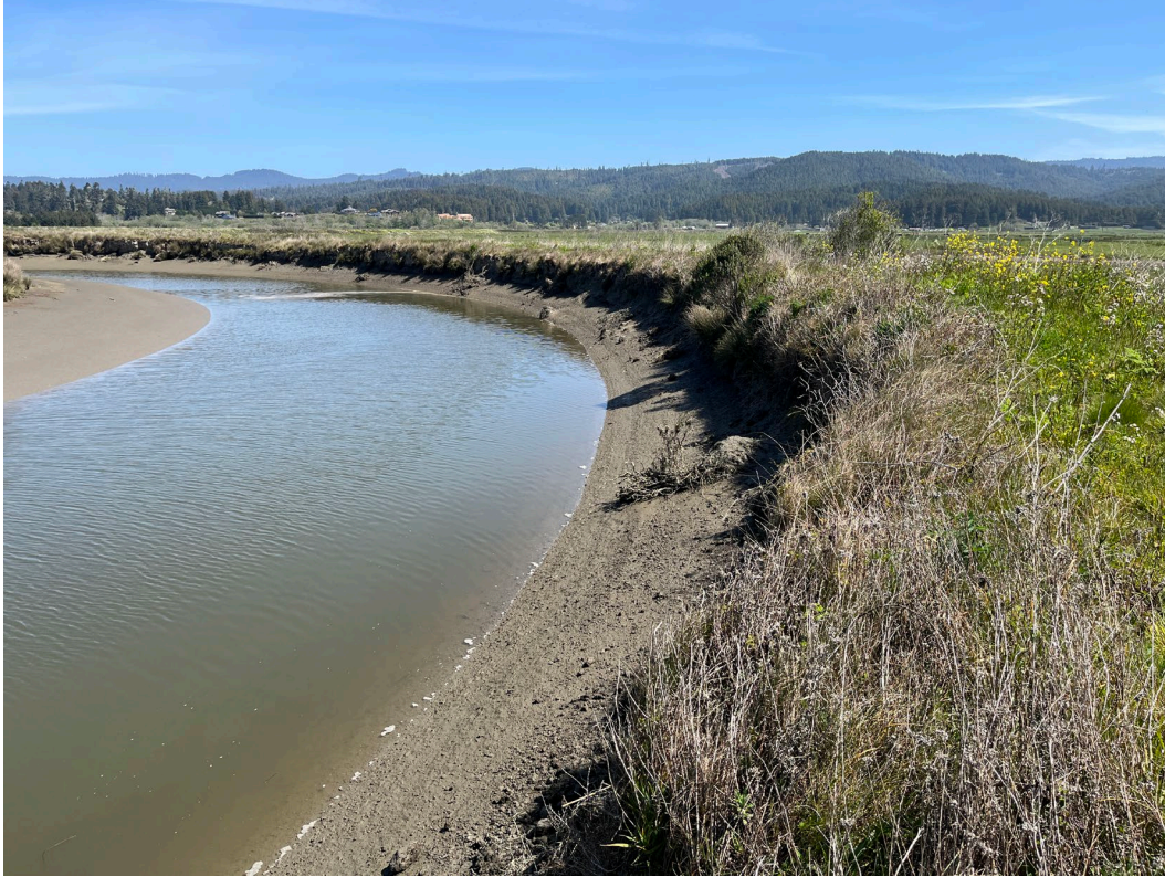
Photo 3. Example of levee edge where erosions is slowly occurring.
