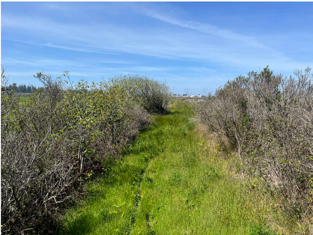
Photo 4. Example of access road along top of levee and vegetation colonizing the levee. The access road is mowed once a year.
