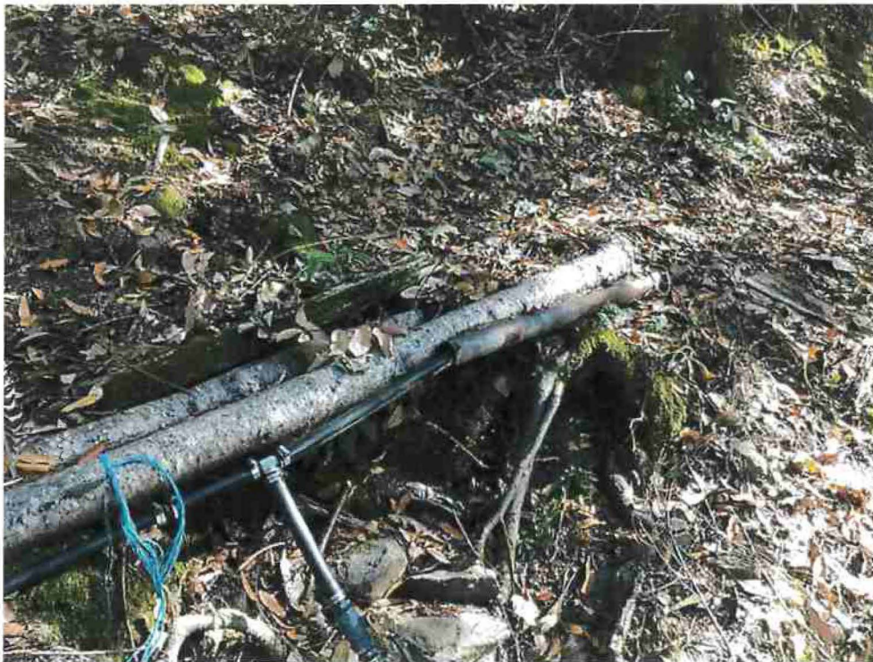
Photo 4. Well infrastructure collecting sub-surface water.
