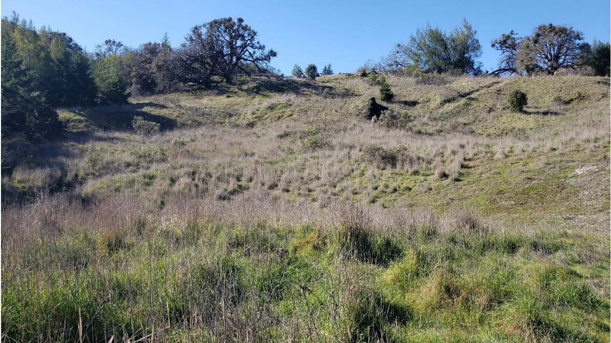
Looking up slope at the southern edge of the graded area and the cutbank above the graded area. The streambed will be restored through this area from center right to lower left of the photo. In this photo, you can see the drainage ditch from the center of the photo going left to the center edge of the photo. This drainage ditch conveys flows that otherwise would have been flows in the native watercourse. During restoration activities this ditch will be breached with the restored watercourse to return flows. The channel that these diverted flows have created will be left alone.
