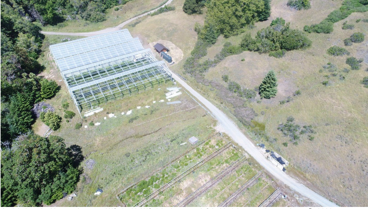
Aerial photo looking northwest at WQ-1 with WQ-2 in the upper left behind the greenhouse. June 4 th , 2020
