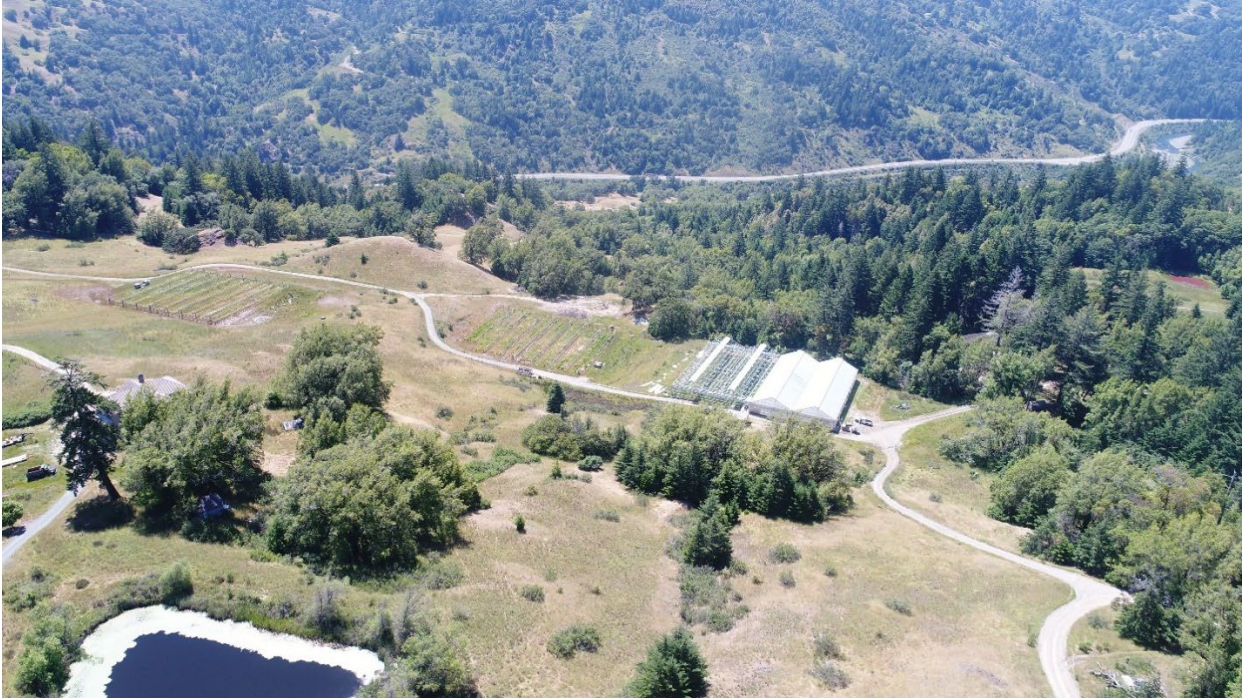
Aerial photo looking southeast at WQ-1 & WQ-2 with the pond at WQ-8 in the lower left. June 4 th , 2020
