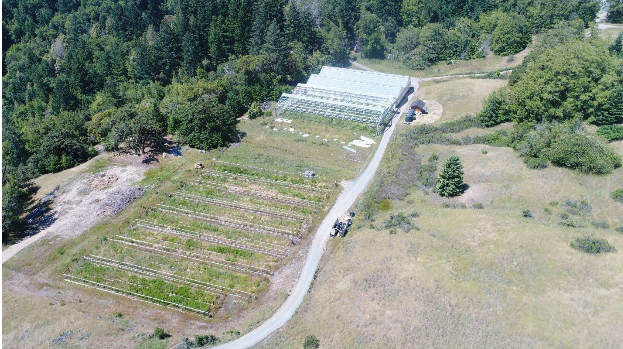
Aerial photo looking southwest at WQ-1 with WQ-2 in the middle-upper right behind the greenhouse. June 4 th , 2020
