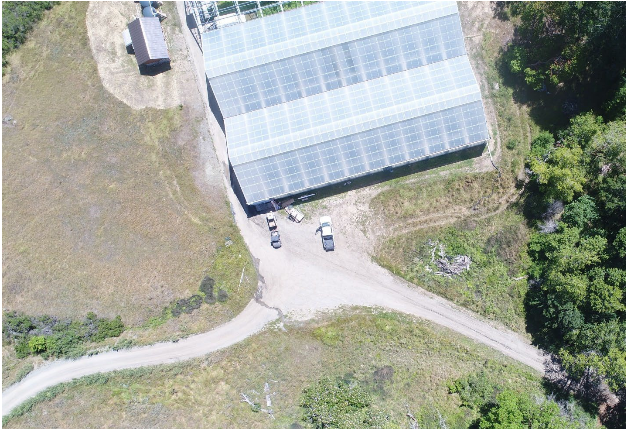
Aerial photo looking down on WQ-2. June 4 th , 2020
