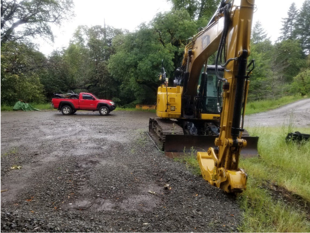
Photo looking south at WQ-4 from just downslope from PM 6. May 5 th , 2020
