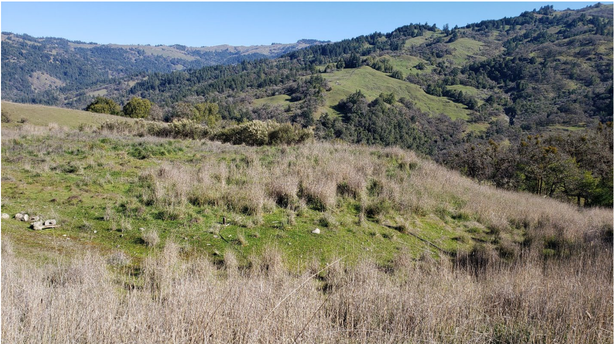
Looking east at the southern edge of the graded area at Site E. This southern edge will be removed (fill pulled back and contoured into the graded area) and the watercourse restored that is underneath it.
