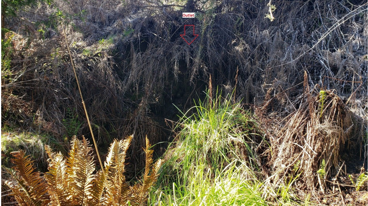
Photo looking southwest directly at the impoundment overflow structure outlet and downhill fillslope toe of the impoundment at WQ-5 from PM 11. March 2 nd , 2021
