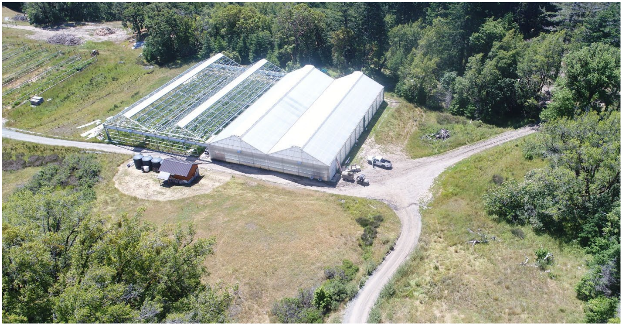
Aerial photo looking southeast at WQ-2. June 4 th , 2020
