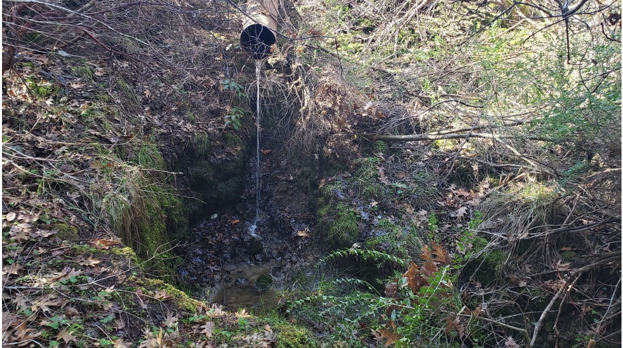
Photo looking west at the impoundment overflow structure outlet at WQ-9. March 2 nd , 2021
