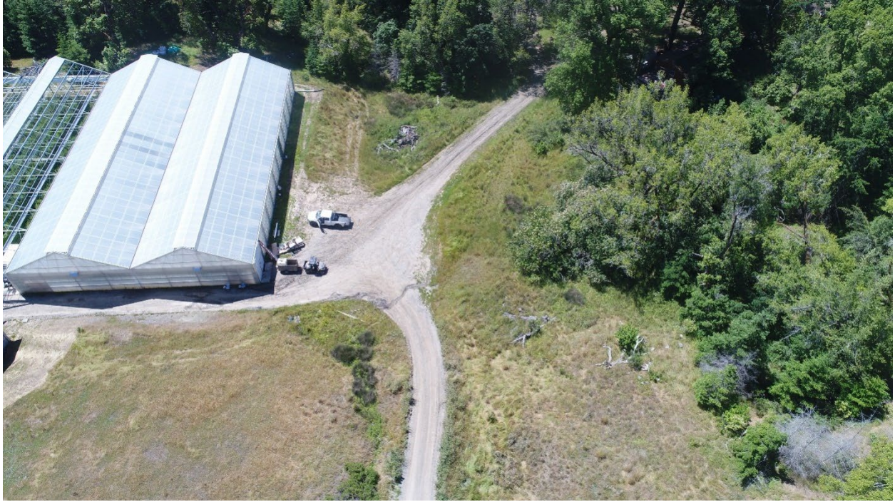
Aerial photo looking south at WQ-2. June 4 th , 2020
