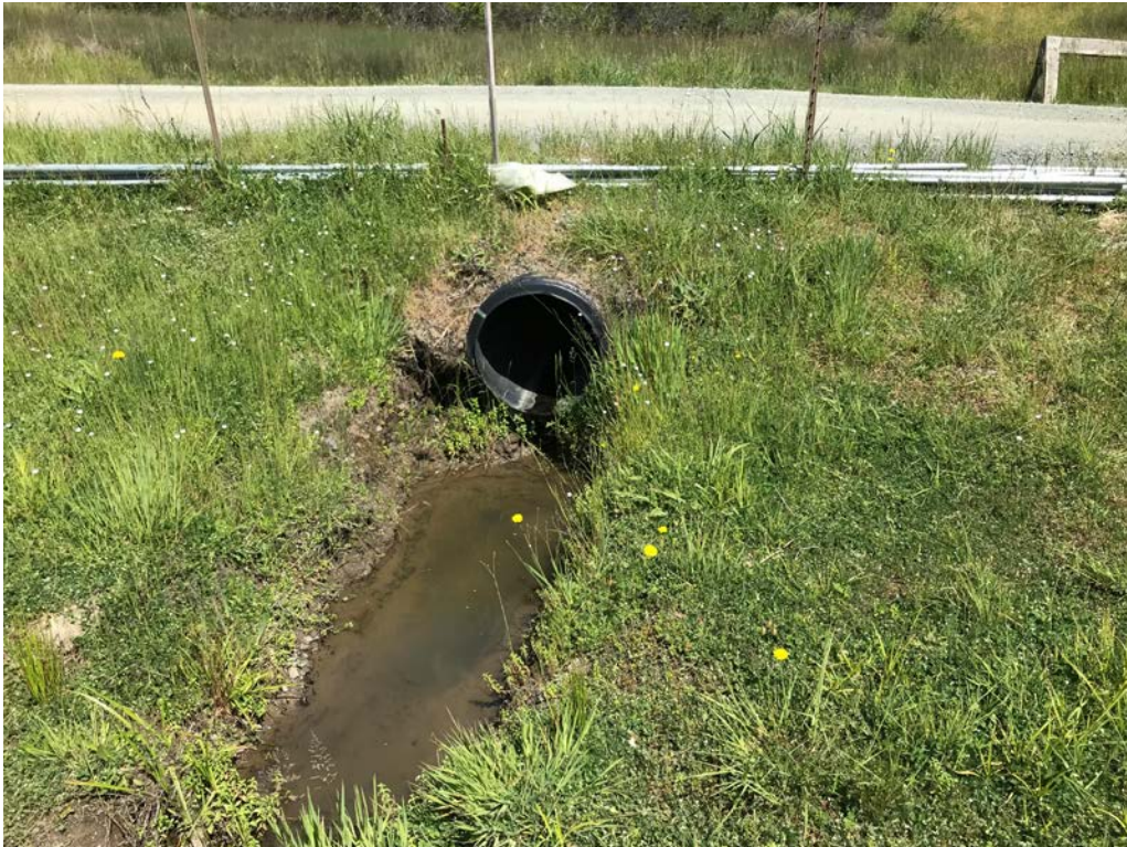
Photo 10. Intermittent stream through disturbed portion of Wetland 1, looking north.
