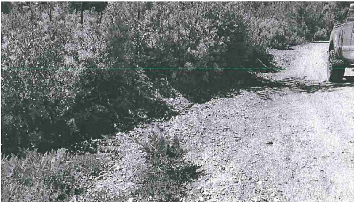
Road Point 3(top) & Road Point 4(bottom): A water bar has been installed in these two locations to direct road runoff. Owner will monitor and maintain the water bars so that road runoff is adequately diverted. 7/12/2016
