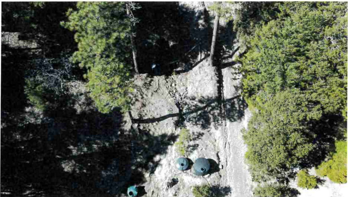
36.0 Cultivation Site E – Erosion Along Road, Storage Tank Within Watercourse
