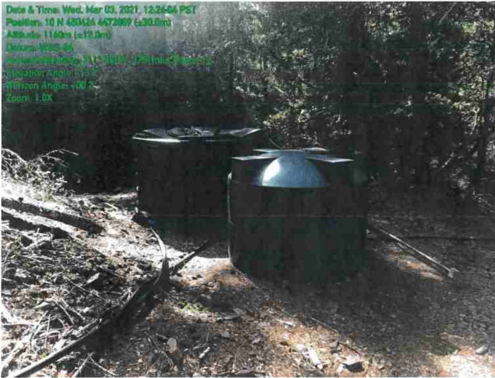
21.0 Water Storage at Cultivation Site B
