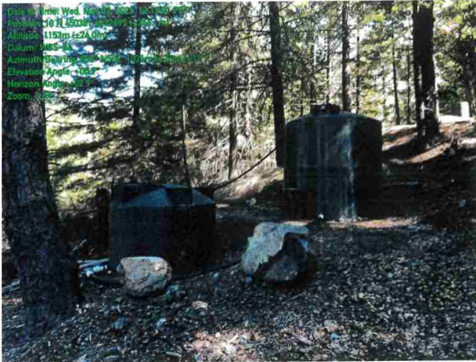
19.0 Water Storage at Cultivation Site E
