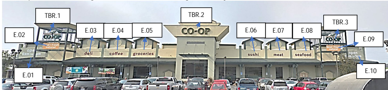
Figure 3: Current storefront with existing signs marked E.01 through E.10 which will remain. Signs marked TBR are to be replaced with new signs. See Table 1 below for sign inventory.
