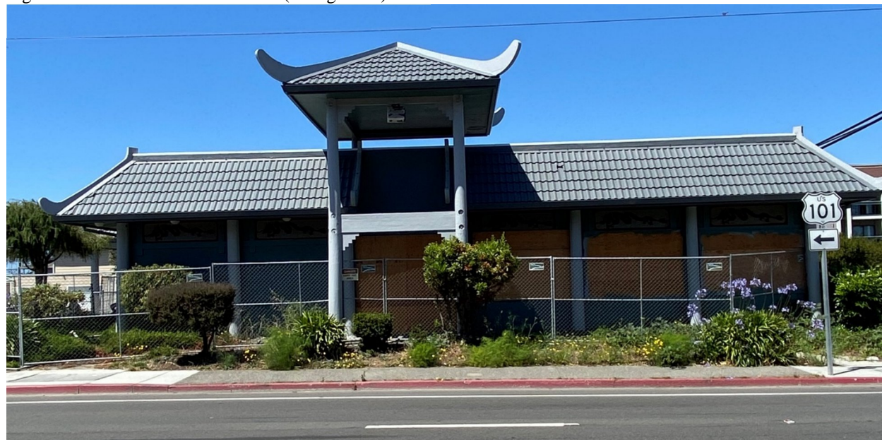
Figure 3: Street view from 4 th Street (facing north)
