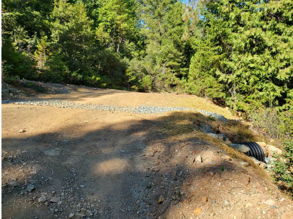
Figure 31: MP10 replaced culvert and rocked road surface.
