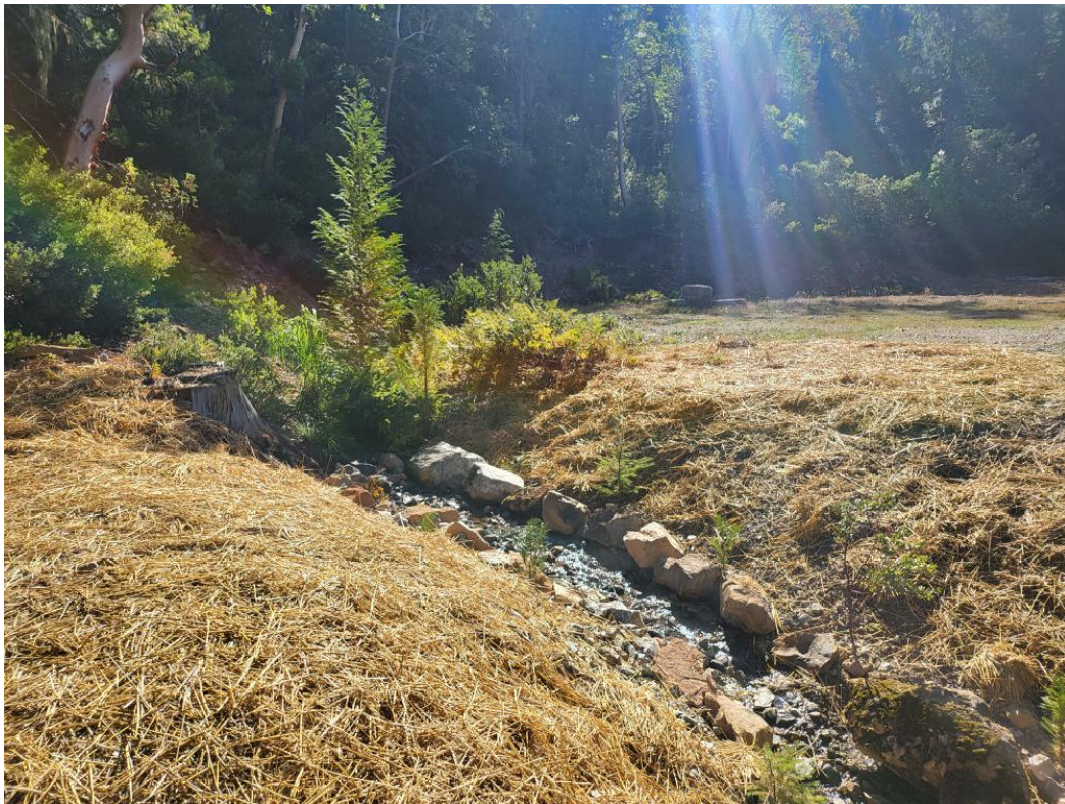
Figure 20: MP8 culvert remove and stream restored.
