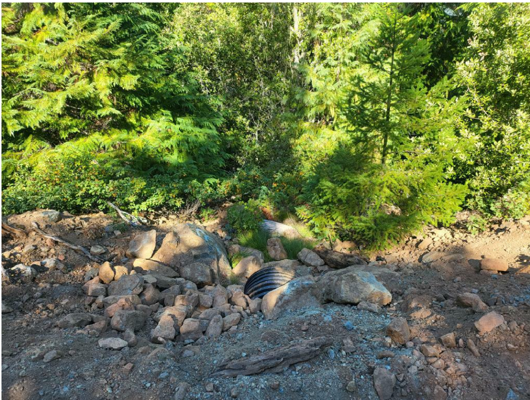
Figure 6: MP3 24" culvert outlet.
