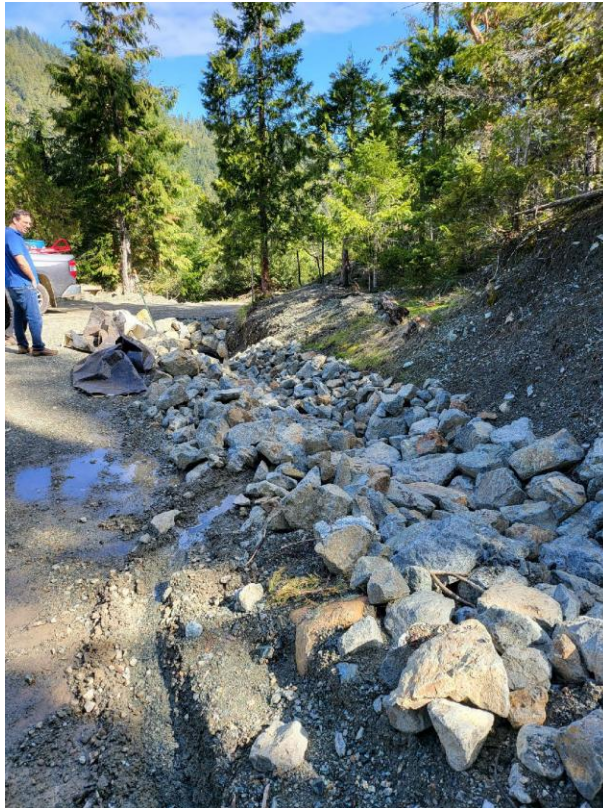
Figure 48: MP19 reestablished channel with rock armor.
