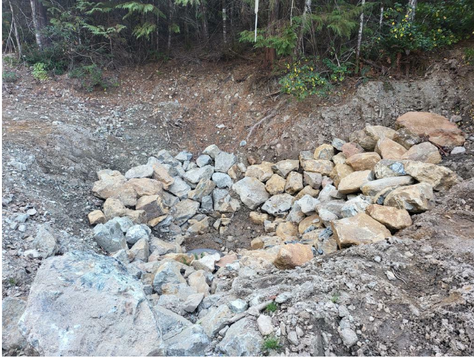
Figure 51: MP20 culvert inlet.
