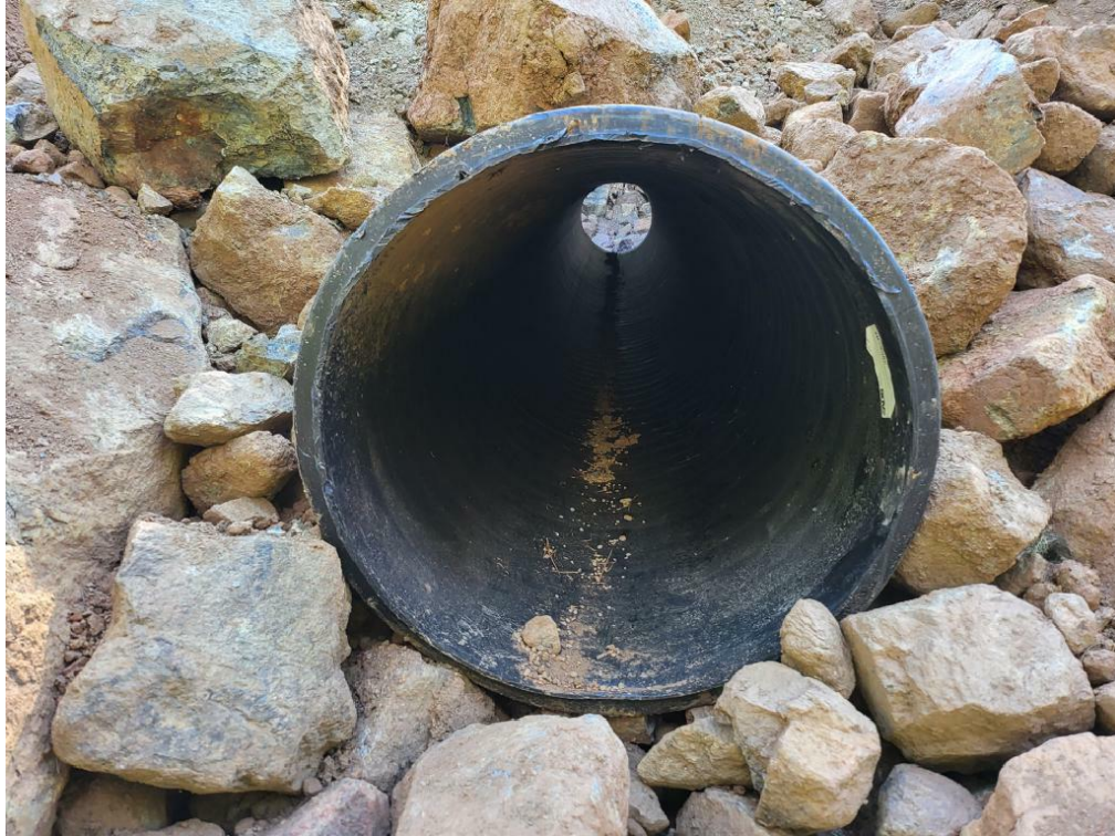
Figure 7: MP3 24" culvert cleared.
