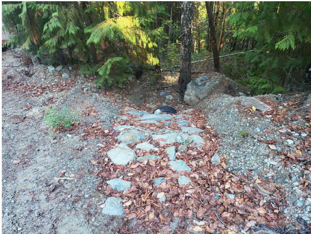
Figure 52: MP20 culvert outlet.
