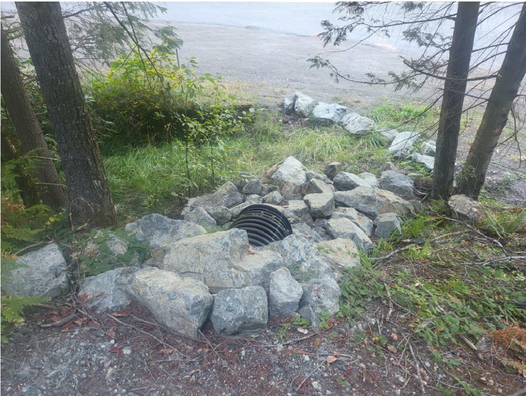
Figure 54: MP21 culvert outlet.
