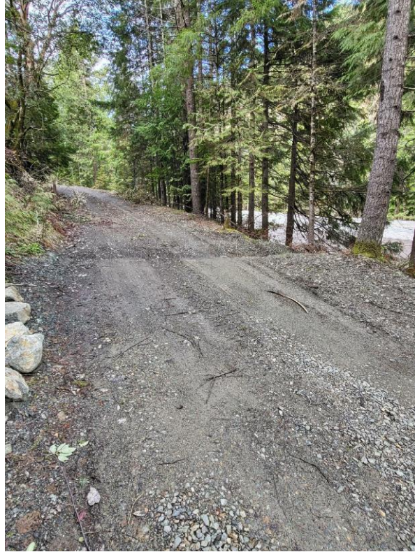
Figure 55: Water bar on roadway above MP21.
