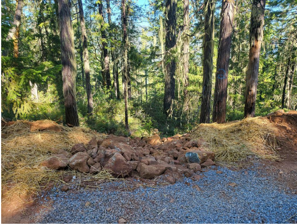
Figure 3: Rock armor placed downstream of MP2.
