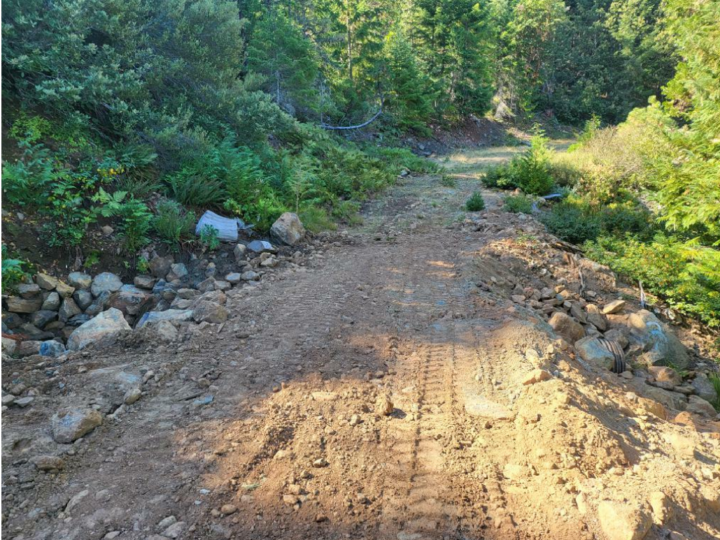
Figure 4: MP3 replaced 24" culvert.
