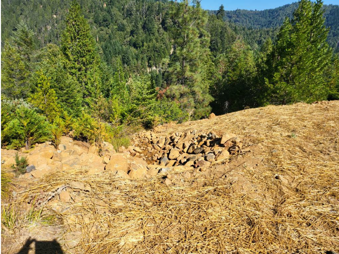
Figure 41: MP13 culvert downstream view.
