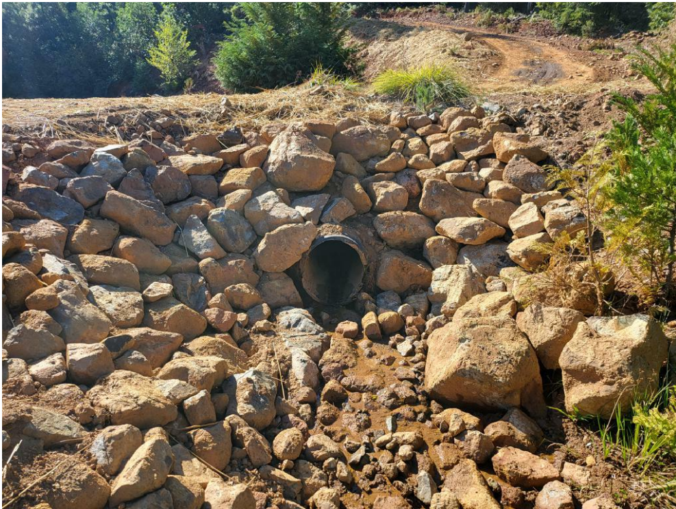
Figure 42: MP13 culvert outlet.
