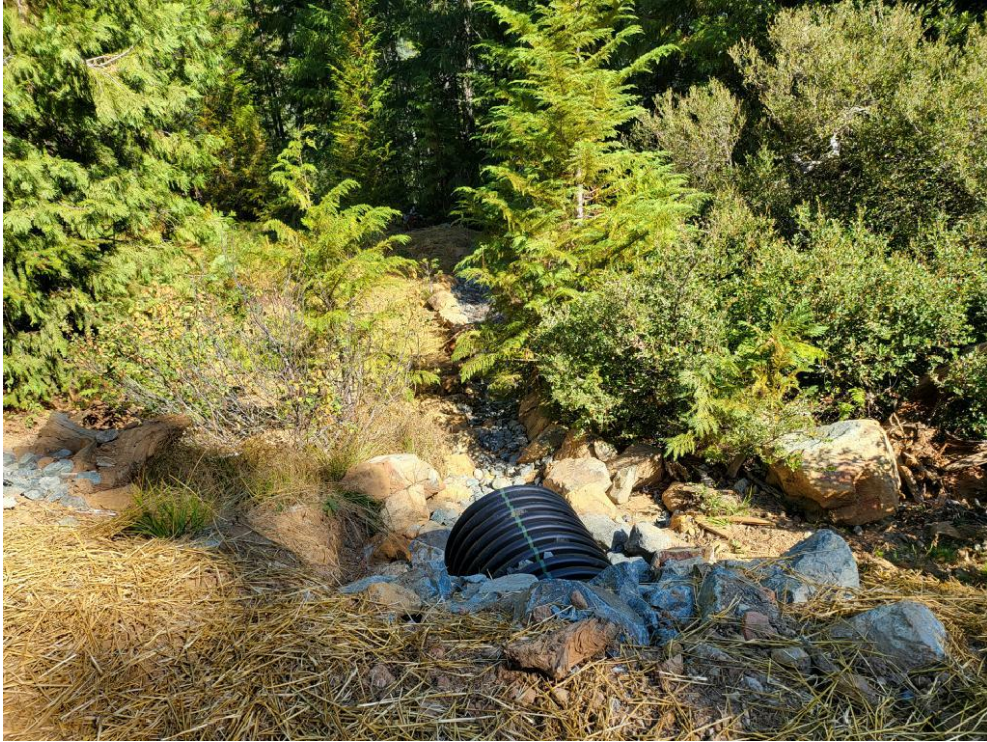
Figure 33: MP10 outlet with reconstructed channel.
