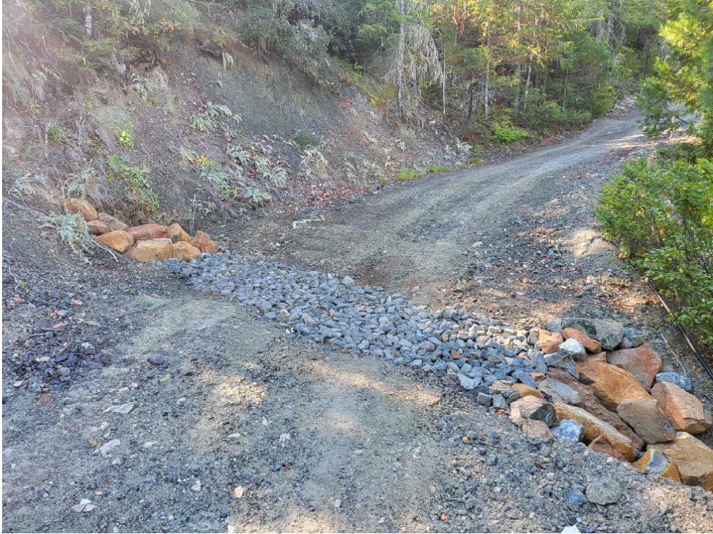
Figure 27: MP9 installed rock armor.
