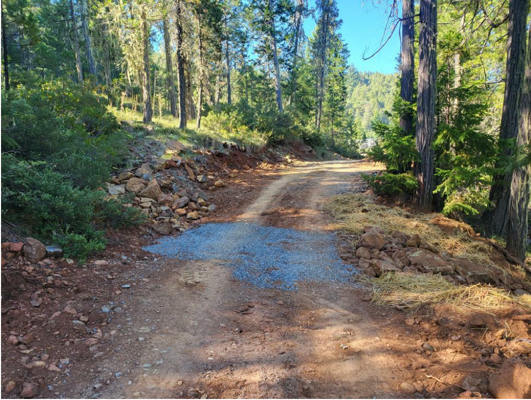
Figure 1: MP2 Installed Rocked Ford.
