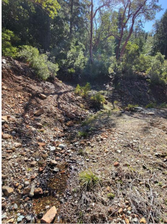
Figure 23: MP8 stream restoration.
