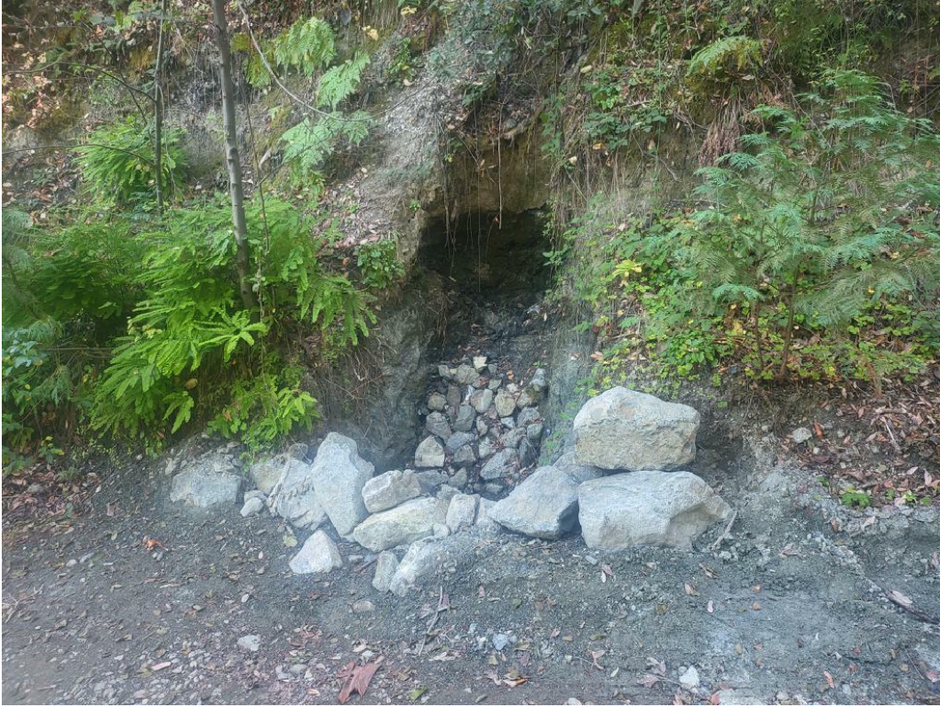
Figure 53: MP21 culvert inlet.
