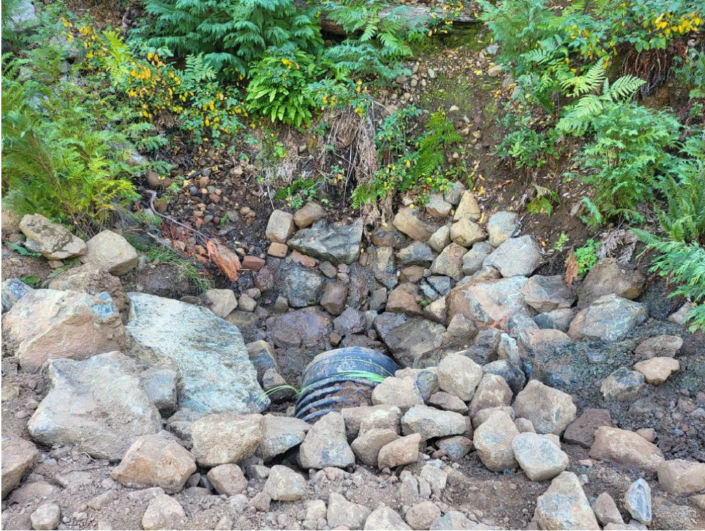
Figure 5: MP3 24" culvert inlet.
