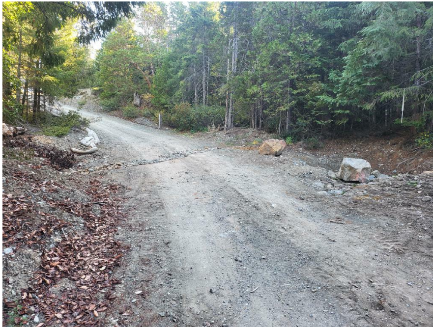
Figure 50: MP20 culvert and water bar.
