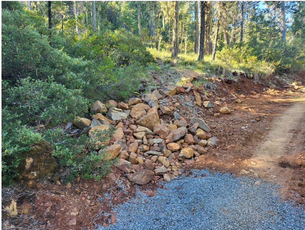
Figure 2: Rock placed upstream of rocked ford crossing.
