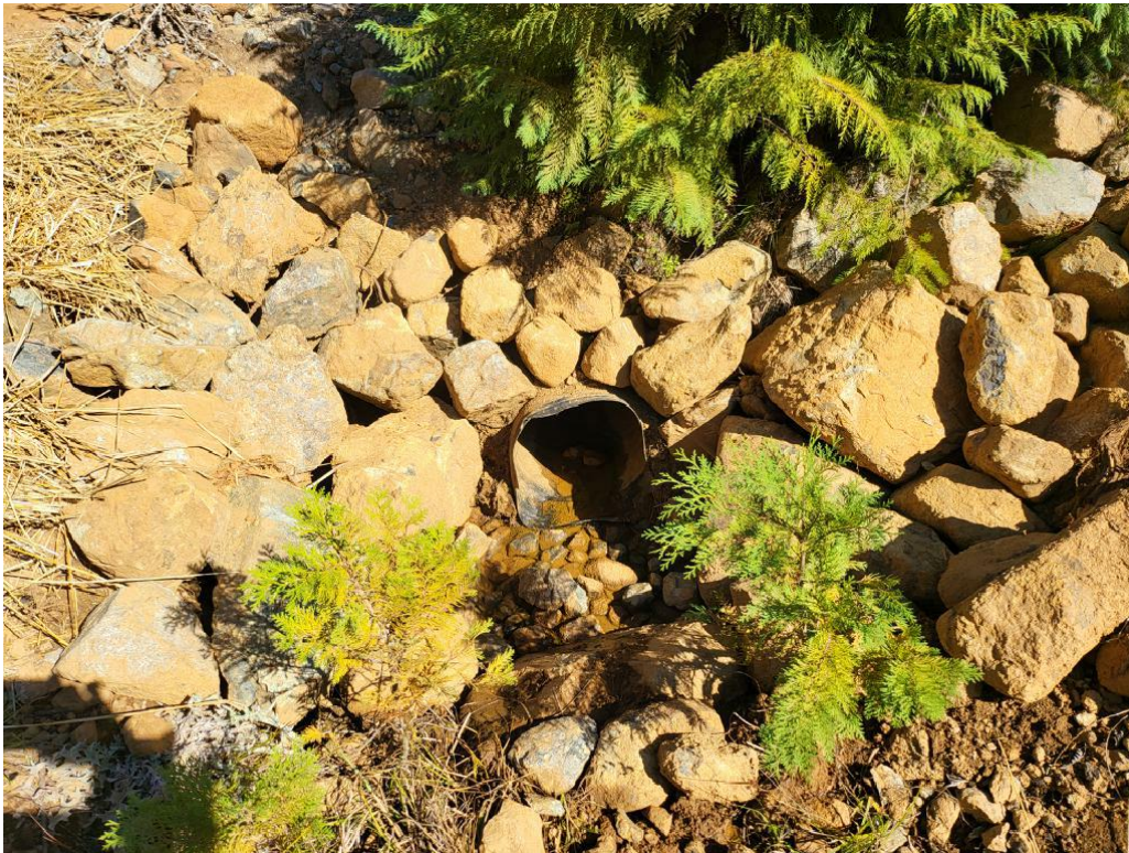
Figure 44: MP13 cleared culvert inlet.
