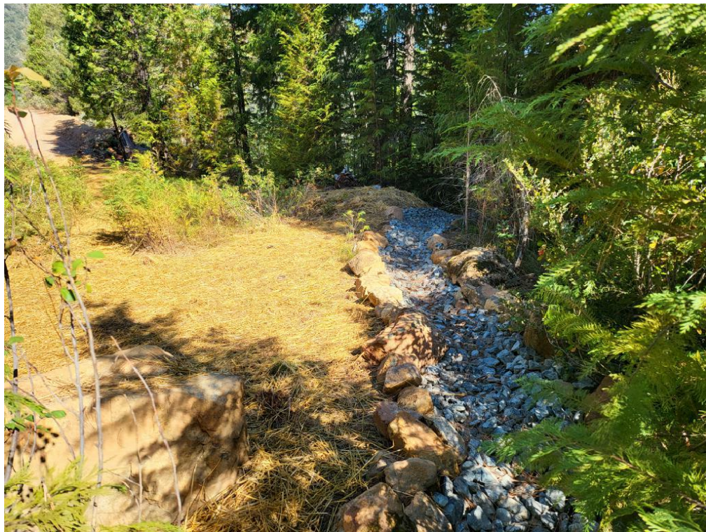
Figure 36: MP10 reconstructed channel, revegetation, and removal of boat.
