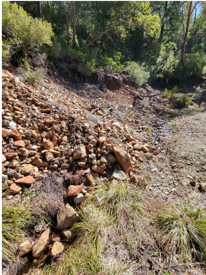
Figure 22: MP8 perched unstable fill removed.
