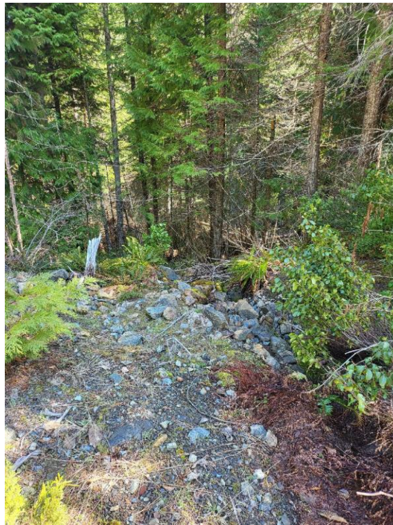
Figure 46: MP14 rock armor.
