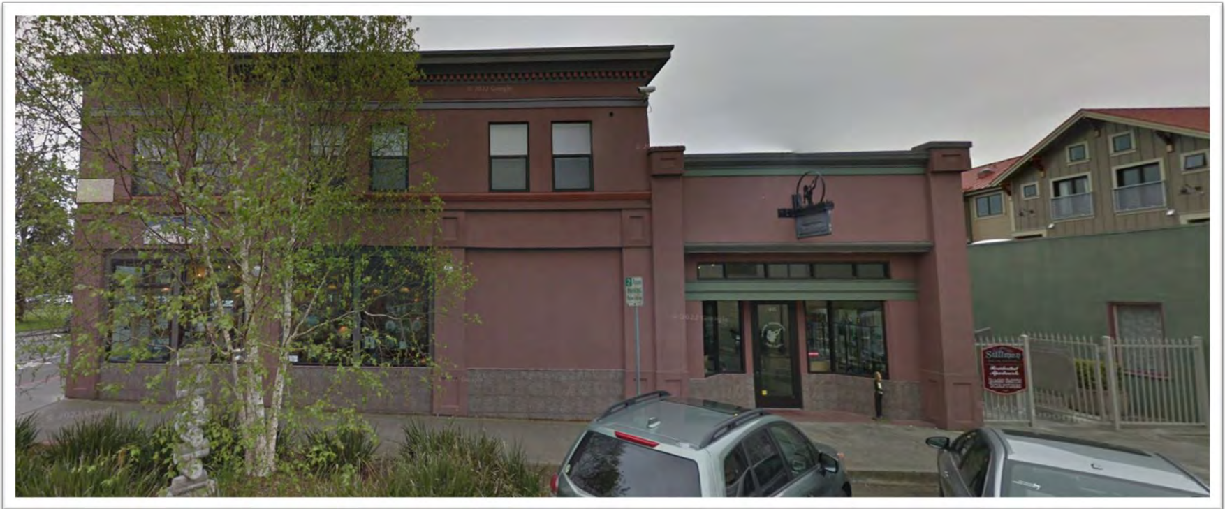
893 H Street and 815 9 th Street – Google Maps image (May 2018) North Building elevation
