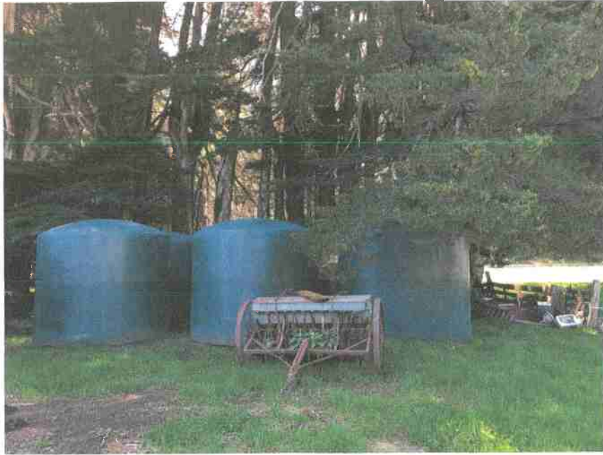
Photo 3: Existing water storage tanks
