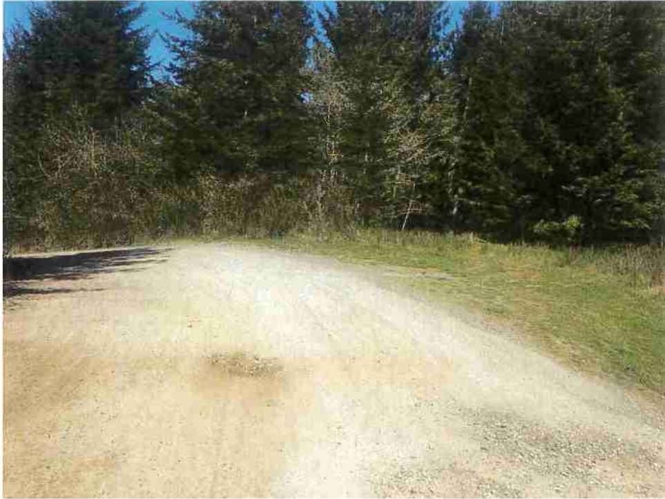
Figure 11: RP 6. 20' road width; unpaved road. 24' wide turnout at bend in road. Image shown facing northwest.
