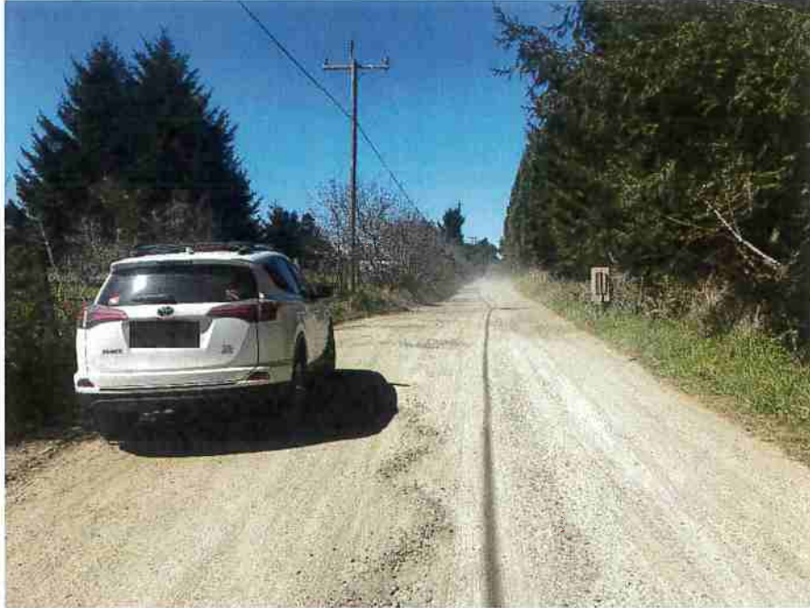
Figure 3: RP 2. Graveled Road Width 16' with 7' wide and 90' long righthand turnout. Image shown facing west.
