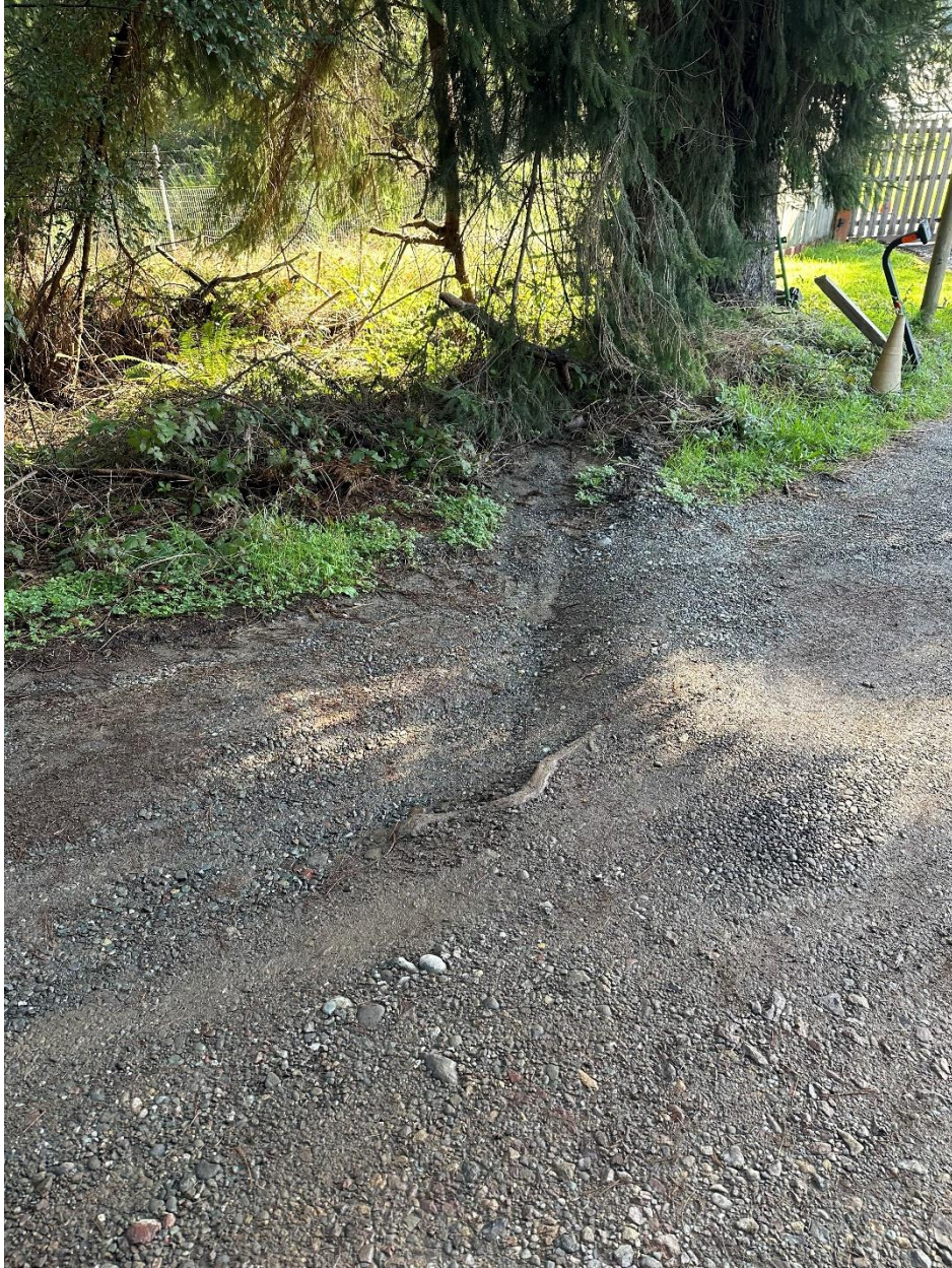
Figure 29: RP 12. Lead-out ditch.
