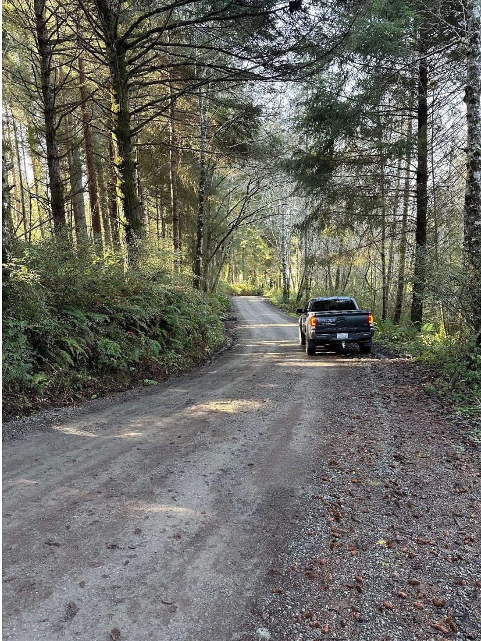
Figure 15: RP 6, typical section of Hooven Road. Photo Taken facing west, vehicle traveling west.
