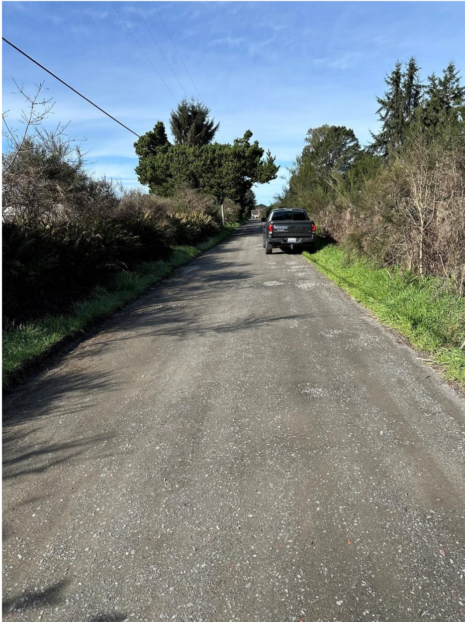
Figure 4: RP 2, typical section of Hooven Road. RP 2, typical section of Hooven Road. Photo Taken facing west, vehicle traveling west.
