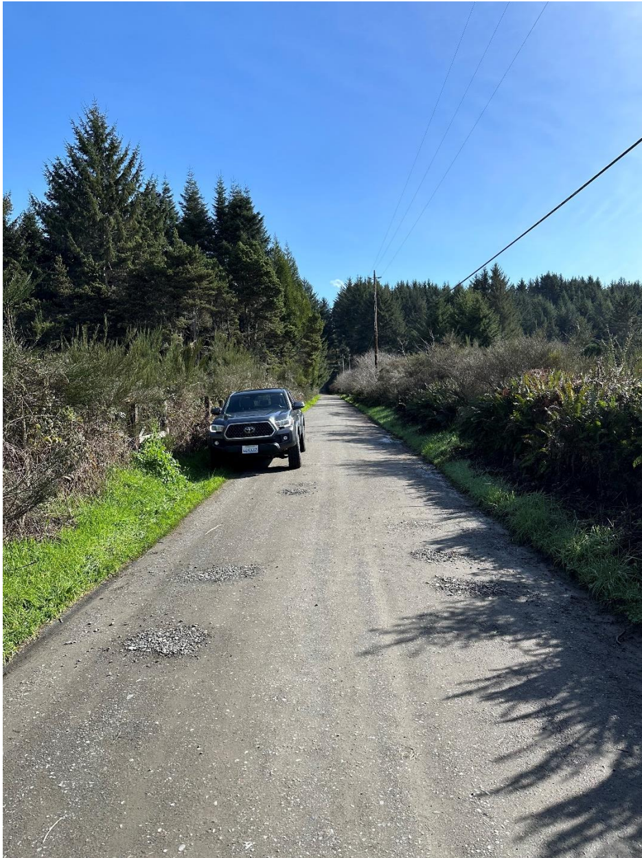
Figure 3: RP 2, typical section of Hooven Road. RP 2, typical section of Hooven Road. Photo Taken facing east, vehicle traveling west.
