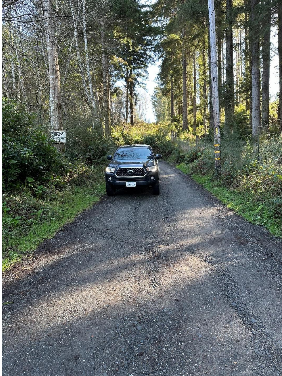
Figure 11: RP 5. Bottom of approaching mild grade. 10% grade for approximately 200 feet in length. Photo Taken facing east, vehicle traveling west.
