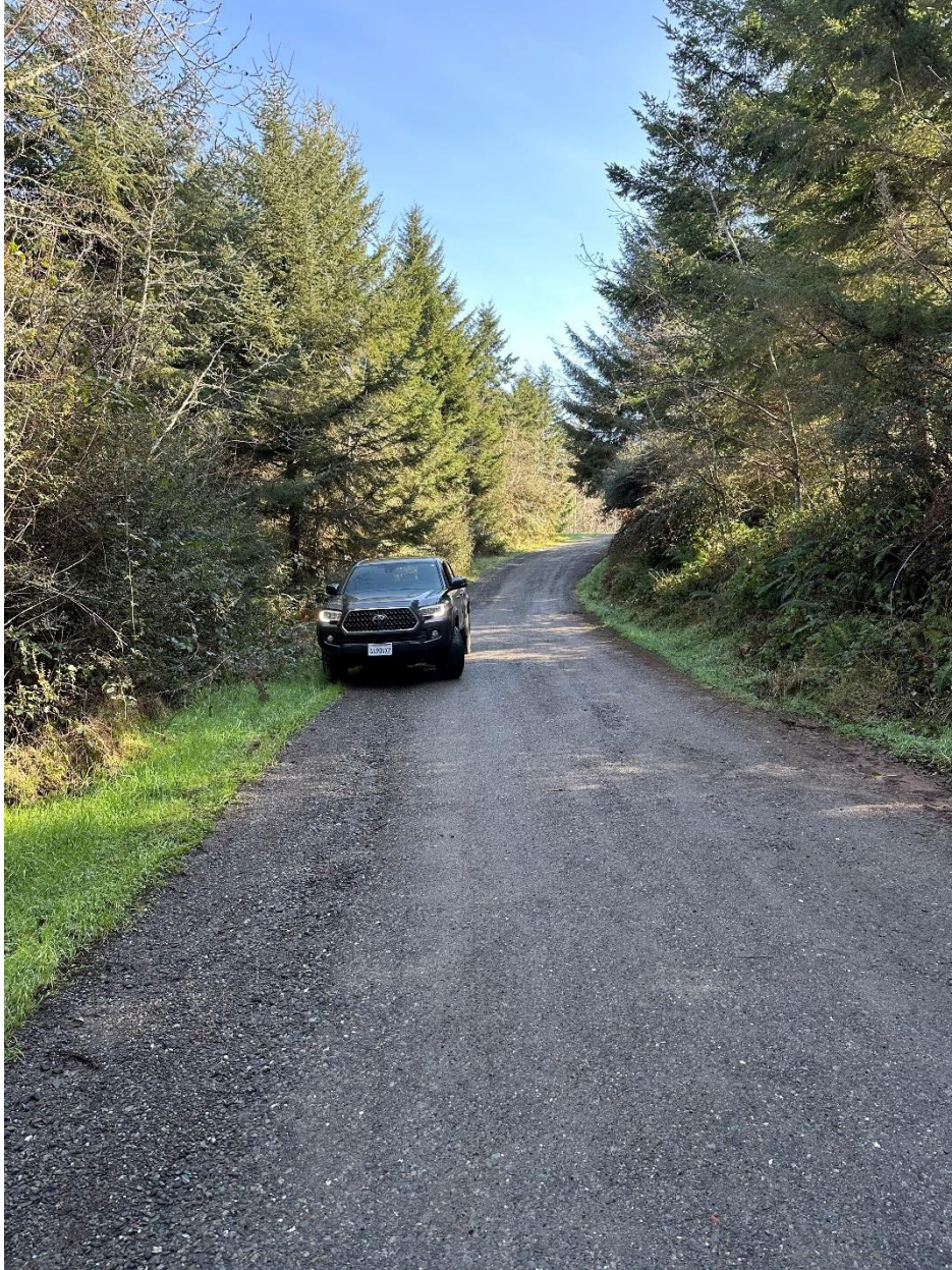
Figure 17: RP 7, typical section of Hooven Road. Photo Taken facing east, vehicle traveling west.
