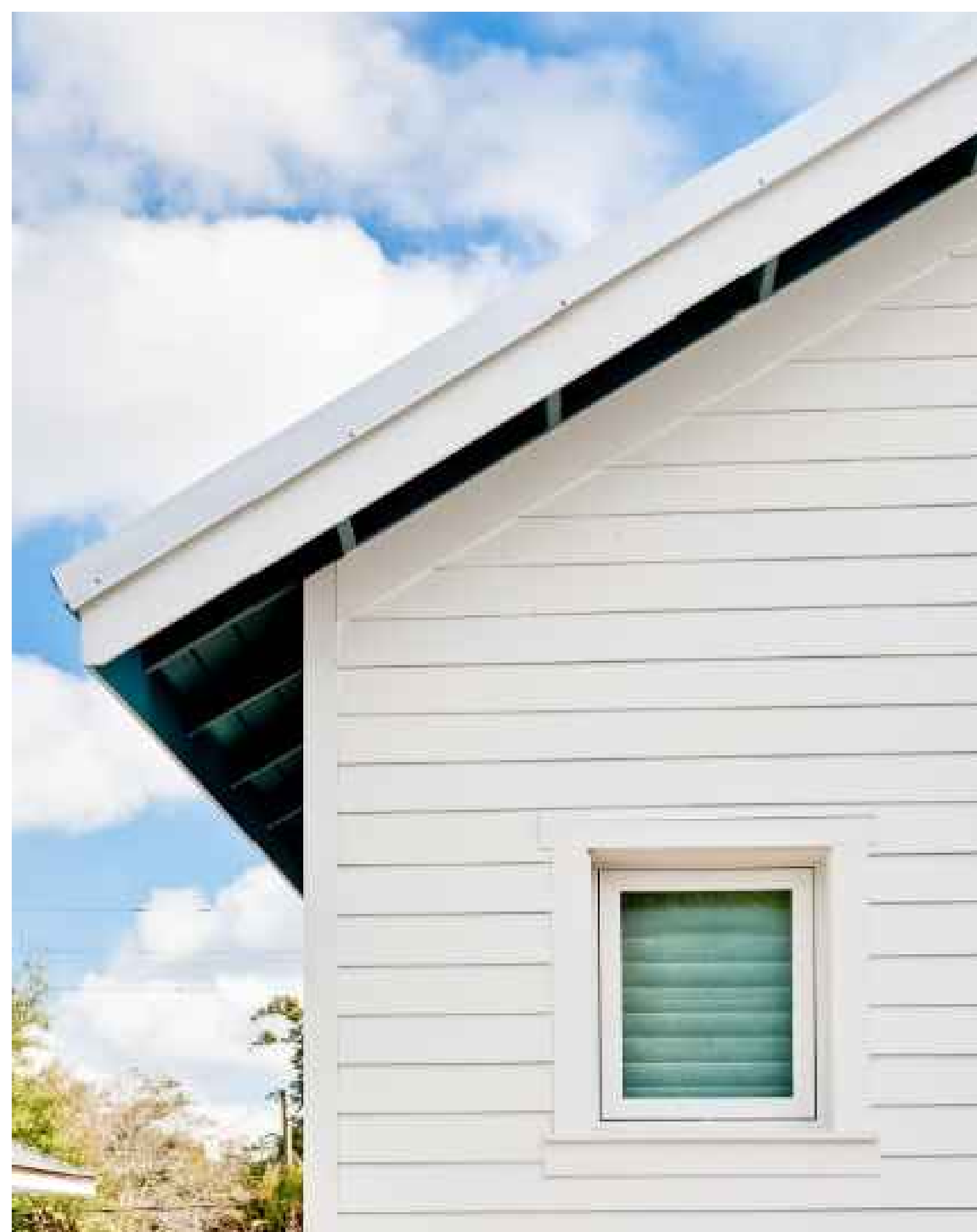
FIBER CEMENT SIDING
