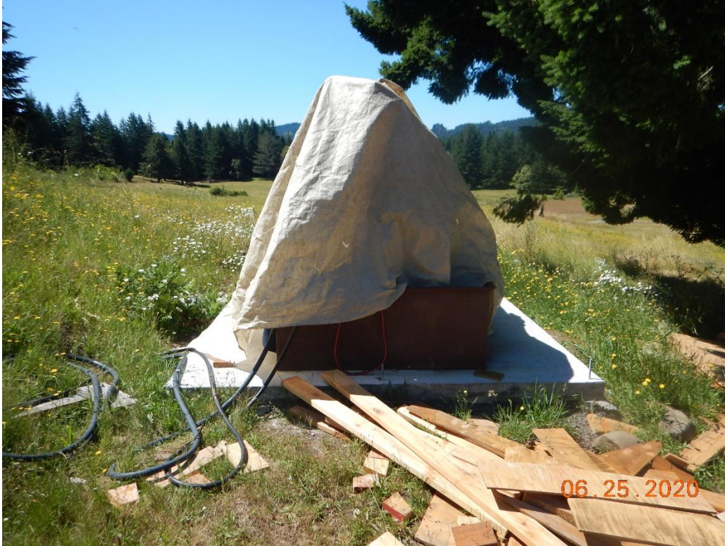
Photo 21. Diesel tank in Containment Post-Pad installation
