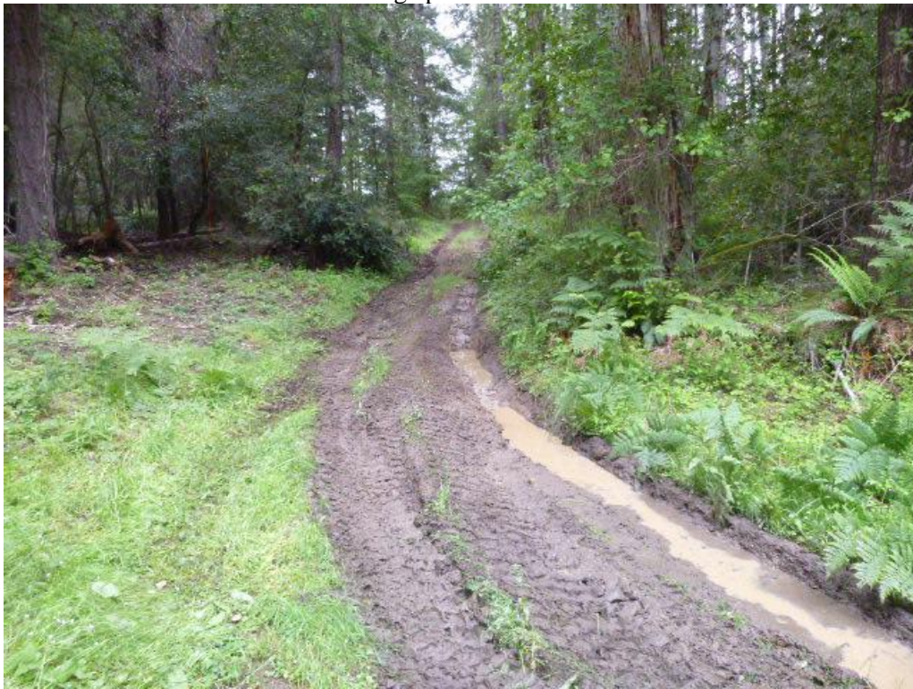
Photo 5. Additional Point 2 (Non-project). Rutted, entrenched road draining to head of Class III below.
