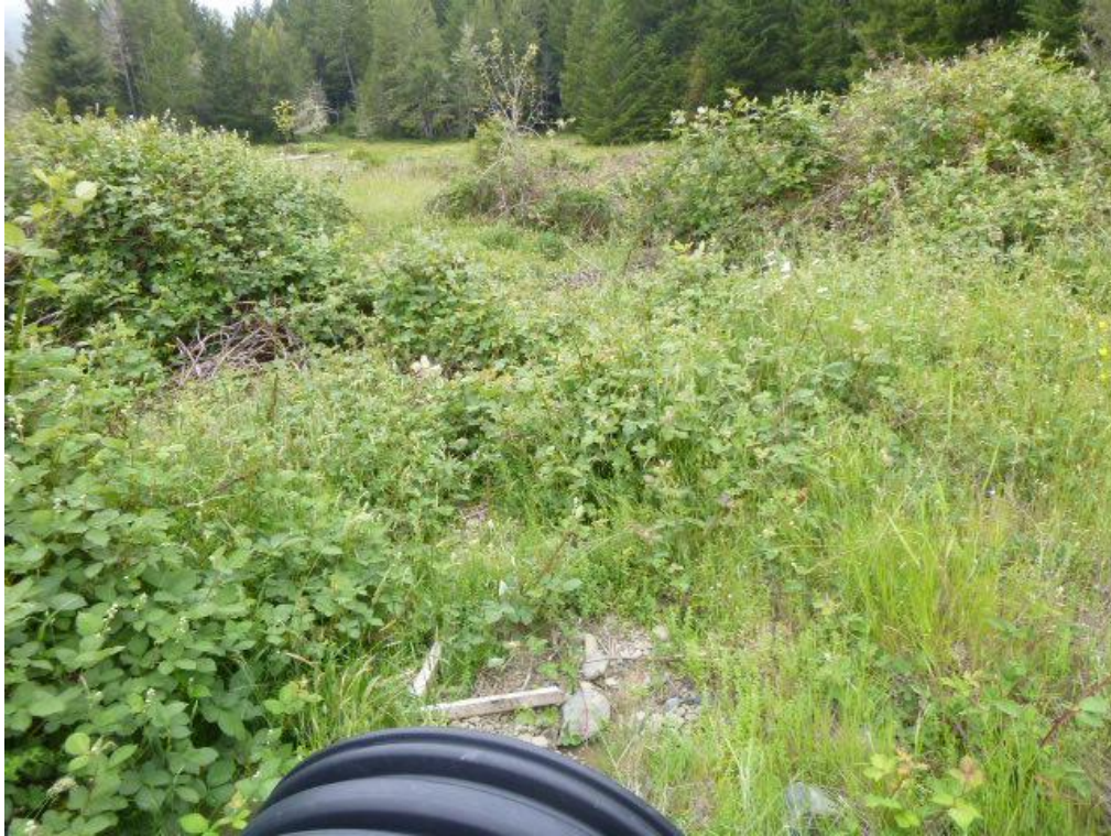
Photo 2. Project 1- Large pond, At the outlet of the overflow culvert on the large pond, with an ephemeral Class III watercourse channel that dissipates approximately 225 feet downslope.
