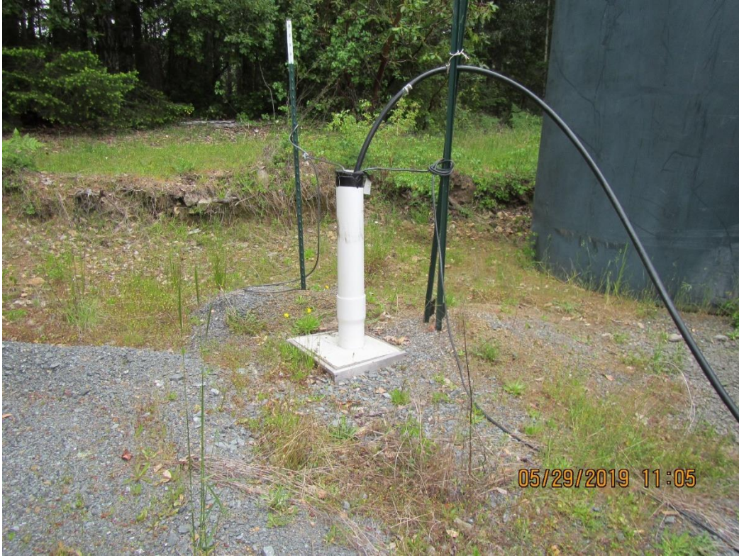
Photo 10. Additional Point 6. Well #1
