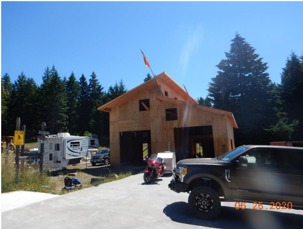
Photo 27. New shop/outbuilding under construction
