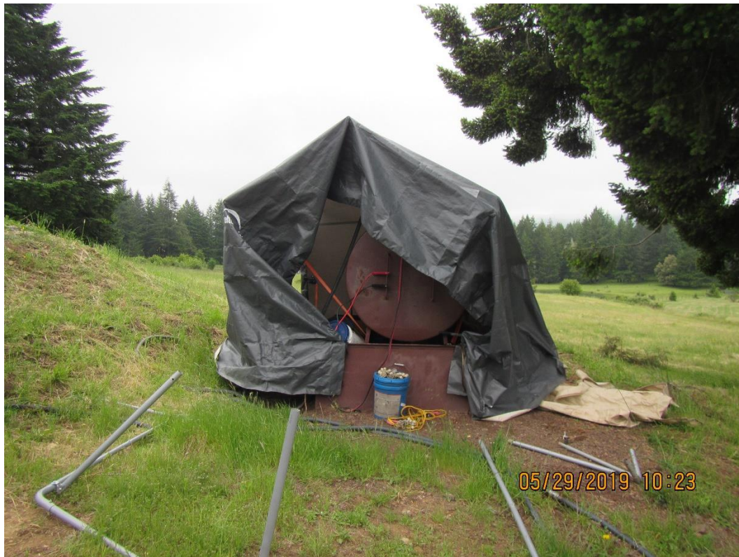
Photo 21. Diesel tank in Containment Pre-Pad installation
