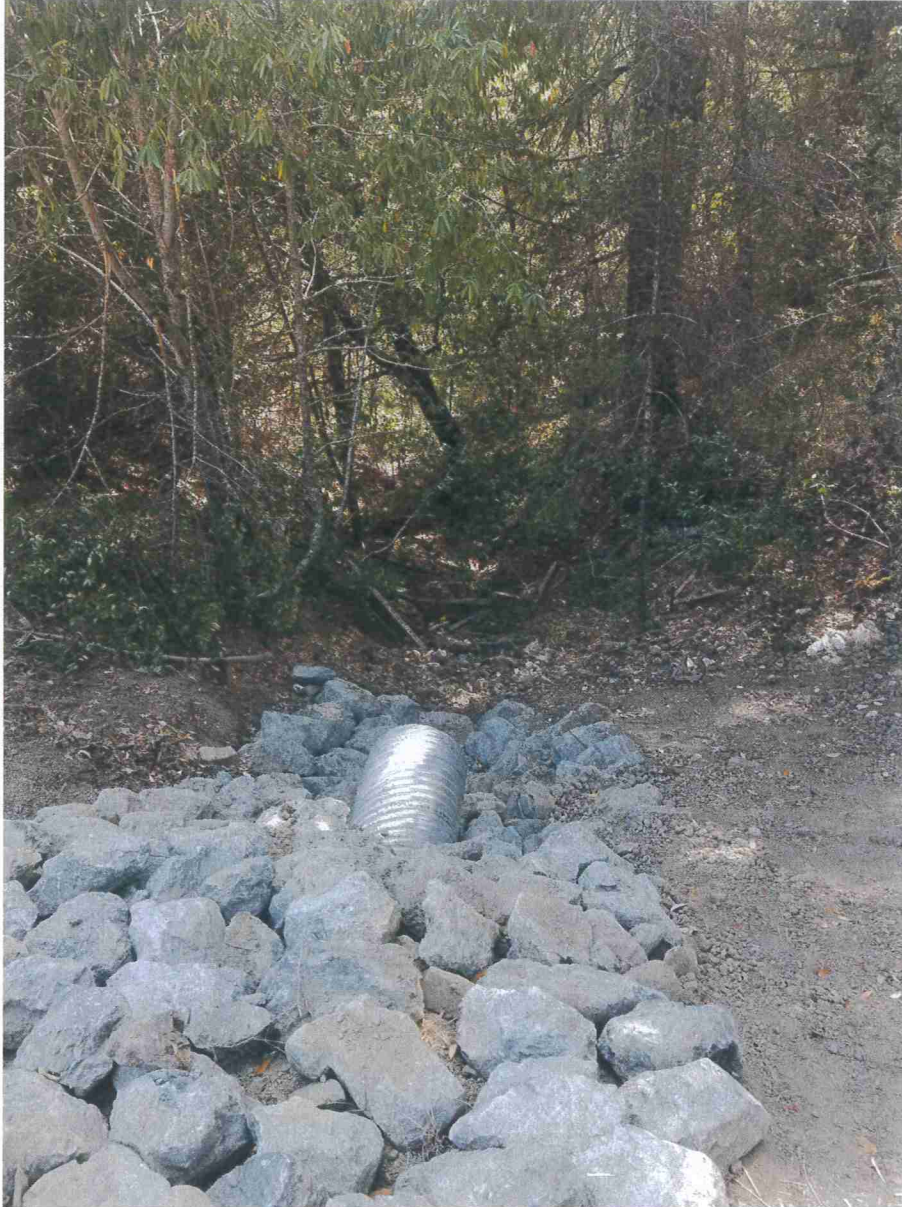
Picture 3: Crossing #1's outlet.
