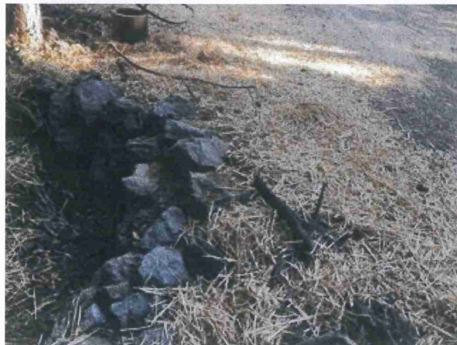
Picture 8 & 9: Crossing #3's inlet (top). Crossing #1's inlet in the process of Erosion Control being applied. (bottom photo was provided by the Applicant on 11-12-2020.)
