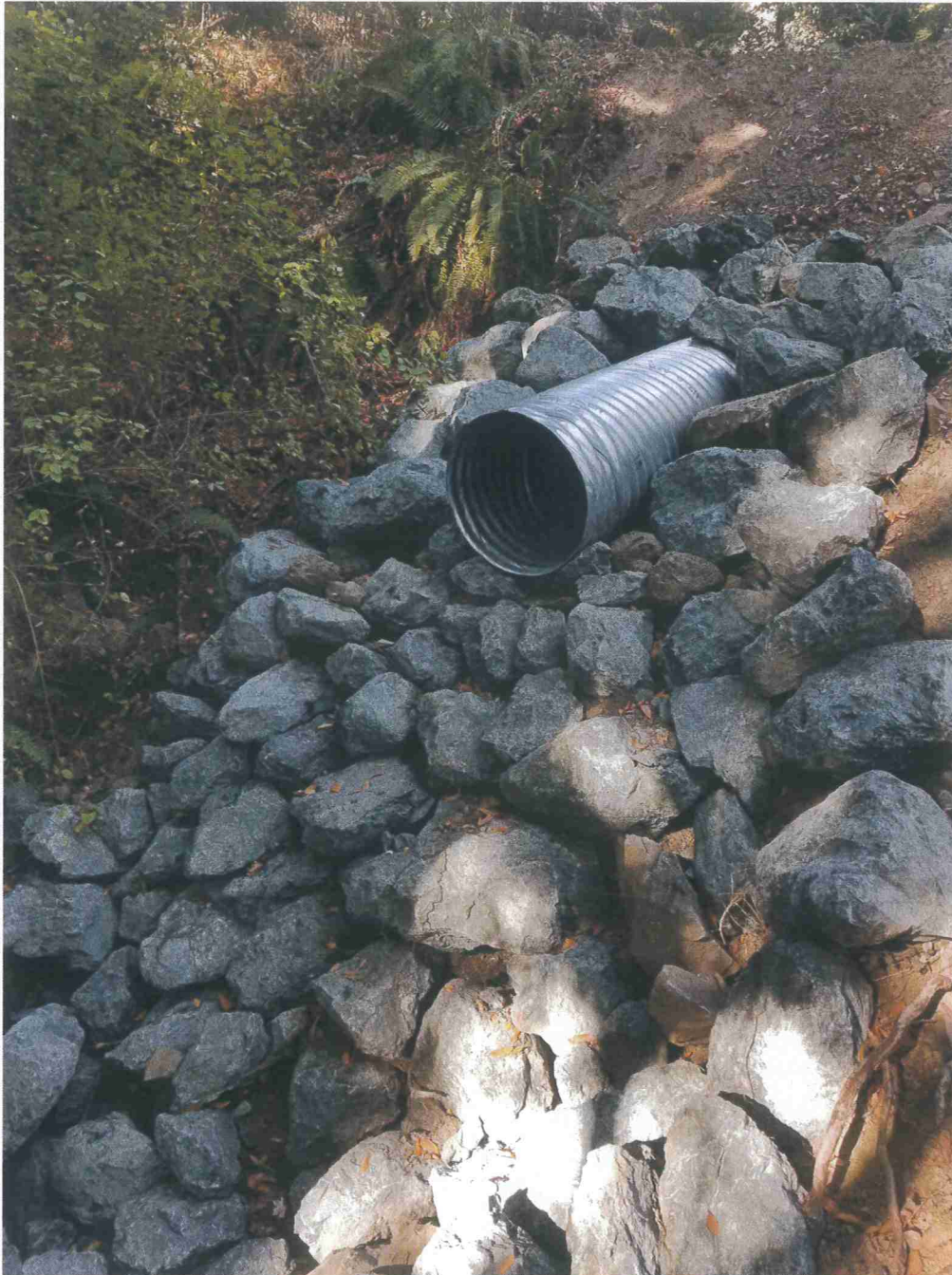
Picture 10: Crossing #3's outlet.
