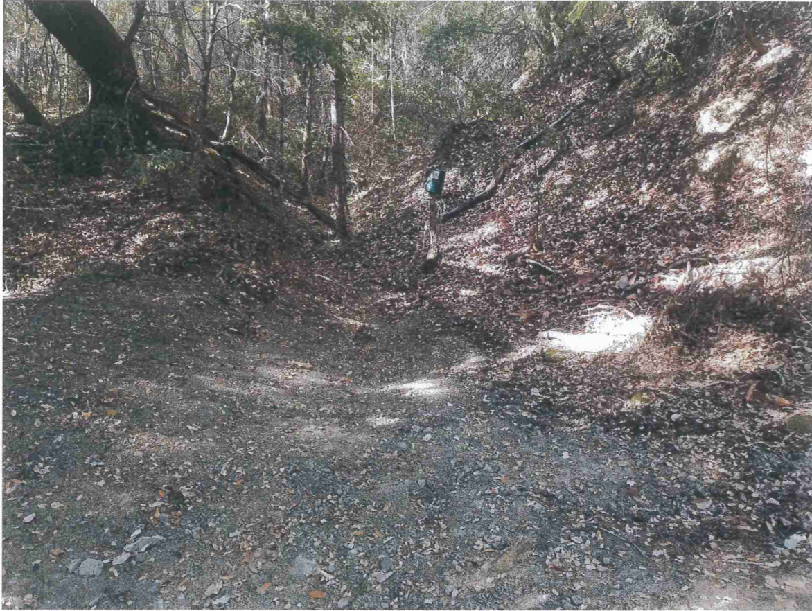
Picture 5: Crossing #2's inlet.
