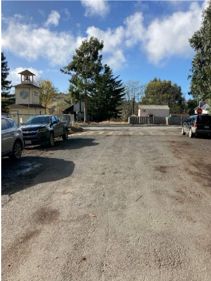
Image 7. Representative of RS2 conditions (looking west) at intersection of Chambers Road and Mattole Road. Details asphalt surface, 25'+ average road width, shoulders, turnouts, crowned geometry with fair drainage, average slopes <5%.
