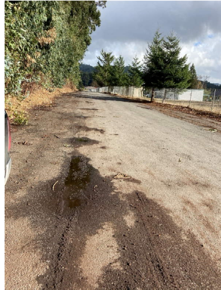
Image 8. Representative of RS2 conditions (looking east) near intersection of Chambers Road and Mattole Road. Details asphalt surface, 25'+ average road width, shoulders, turnouts, crowned geometry with fair drainage, average slopes <5%.
