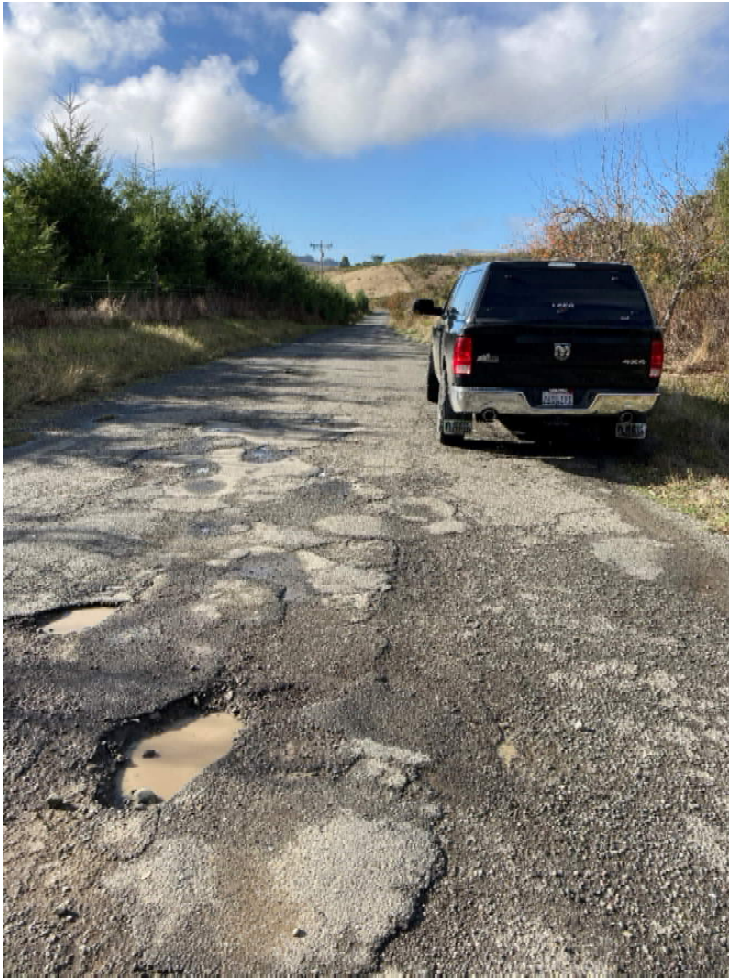
Image 5. Representative of RS2 conditions (looking west). Details asphalt surface, 20'+ average road width, shoulders, turnouts, crowned geometry with fair drainage, average slopes <5%.
