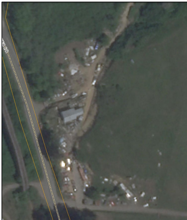
Eel River Drive before abatement
