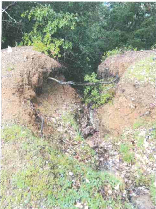
Unprotected discharge point.
