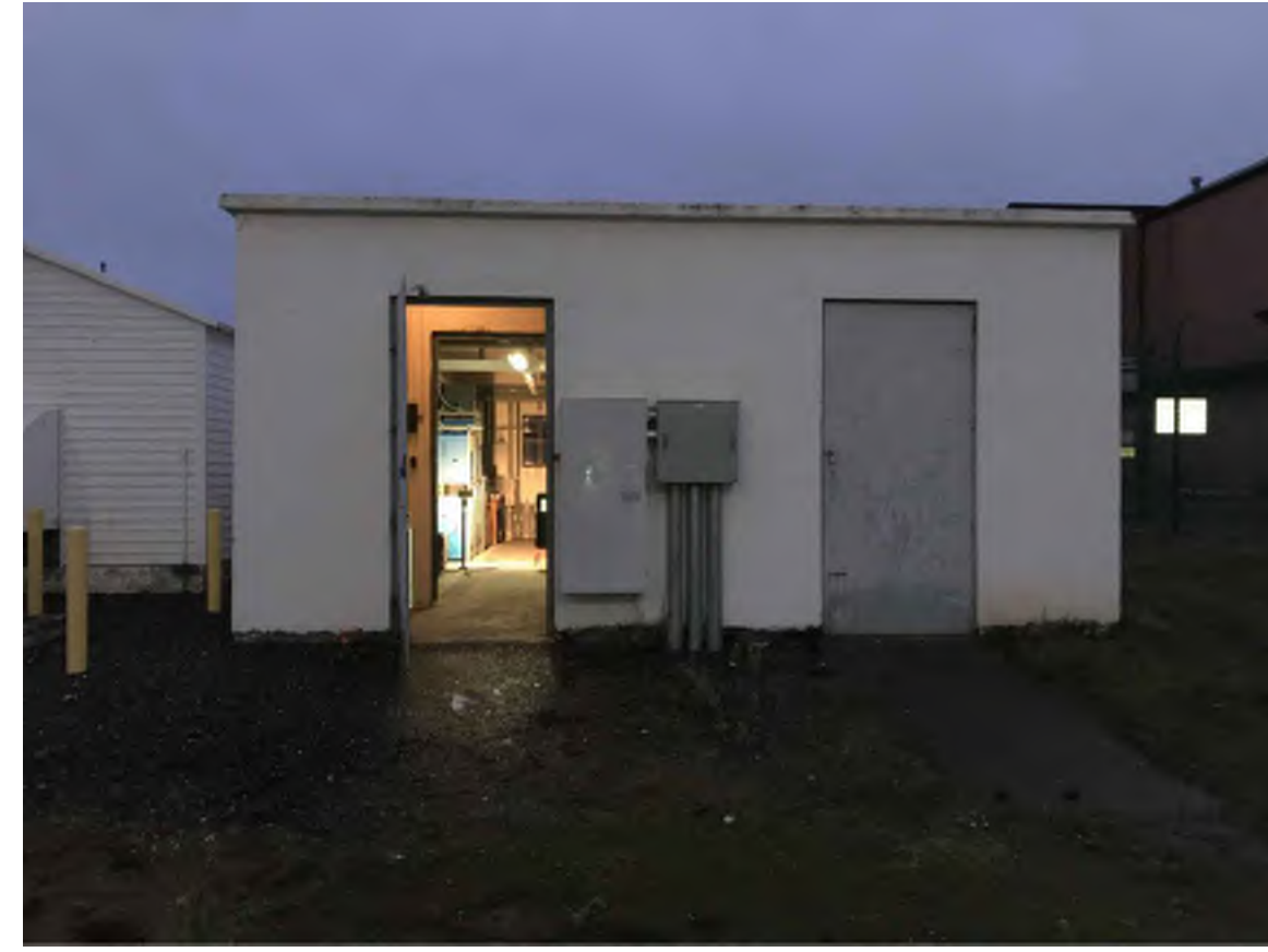
2 EXISTING VAULT ENTRANCE SCALE: NTS
