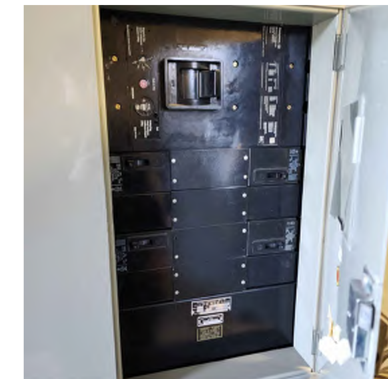
3 MAIN BREAKER PANEL SECTION 1 SCALE: NTS
