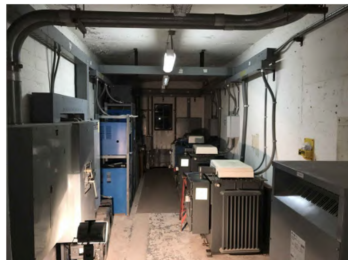
7 EXISTING VAULT INTERIOR SCALE: NTS
