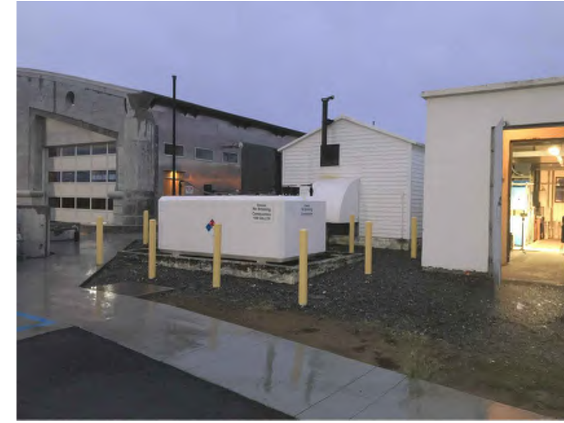
3 EXISTING VAULT ENTRANCE SCALE: NTS
