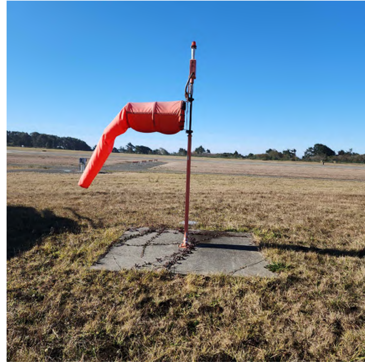
4 14-32 NORTH WINDCONE SCALE: NTS
