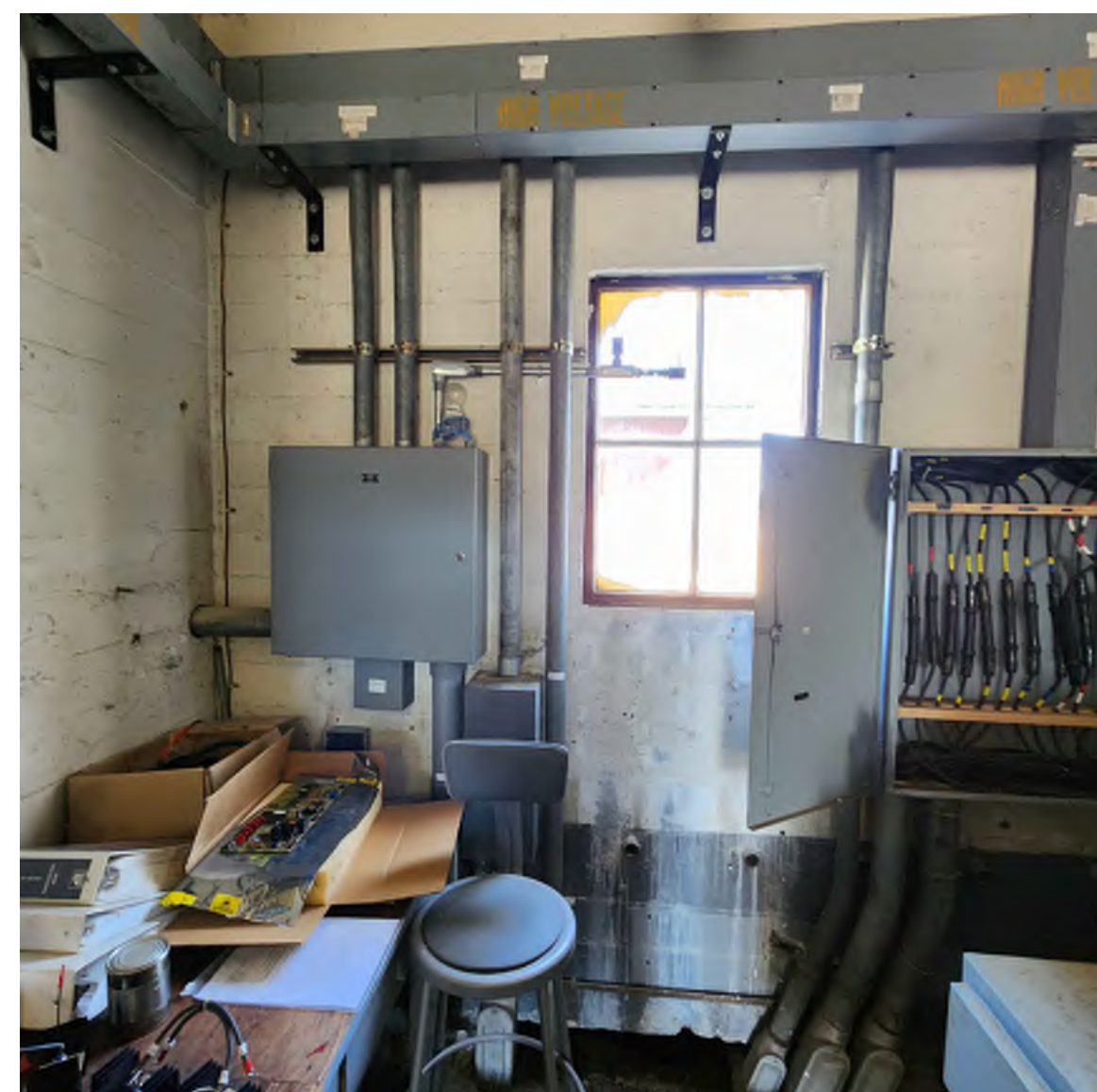
7 EXISTING VAULT INTERIOR SCALE: NTS
