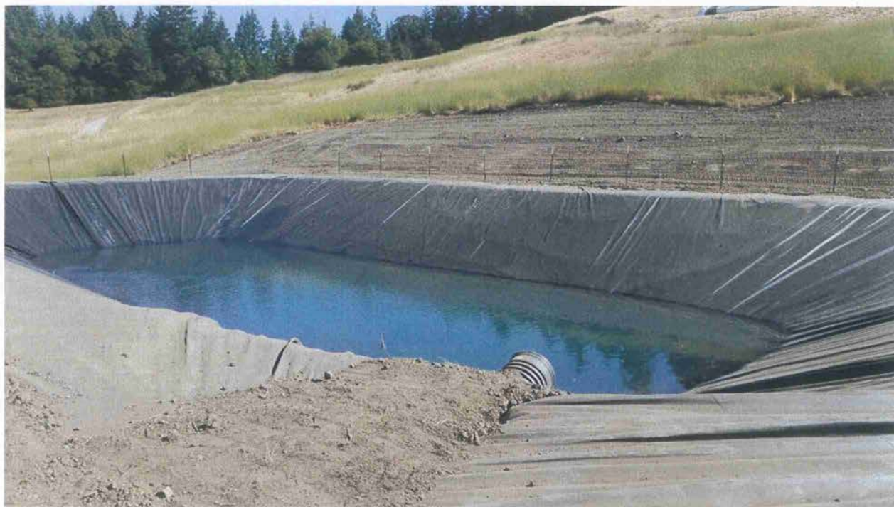
Picture 7: 350,000-gallon rain catchment pond. Photo date 7-06-2017.
