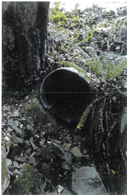
Photo looking at the outlet of the watercourser crossing at Site 22. Photo date 6-11-2016
