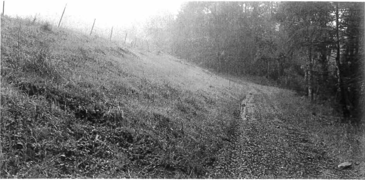
Photo looking southeast the the southern pond embankment.
