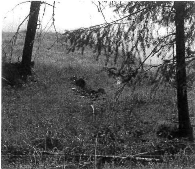
Photo looking at the outlet of the pond overflow.
