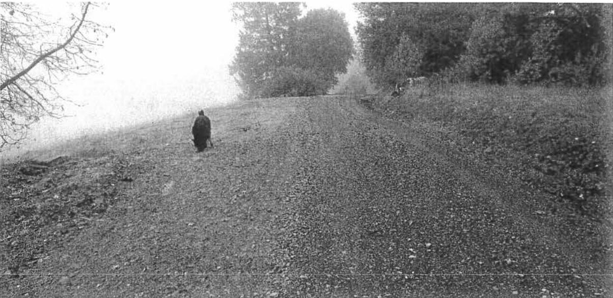
Photo looking down grade at Site 18. Note road rock surfacing and the stable road base. The majority of roads on the property are in similar condition.
