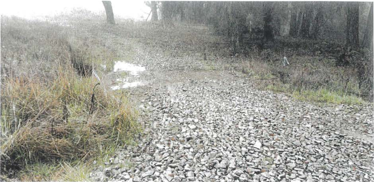
Photo looking southeast at the rocky ford watercourse crossing at Site 12. An 18" D x 20' culvert is being proposed as an upgrade to this crossing, per request by CDFW and North Coast Regional Water Quality Board personnel.
