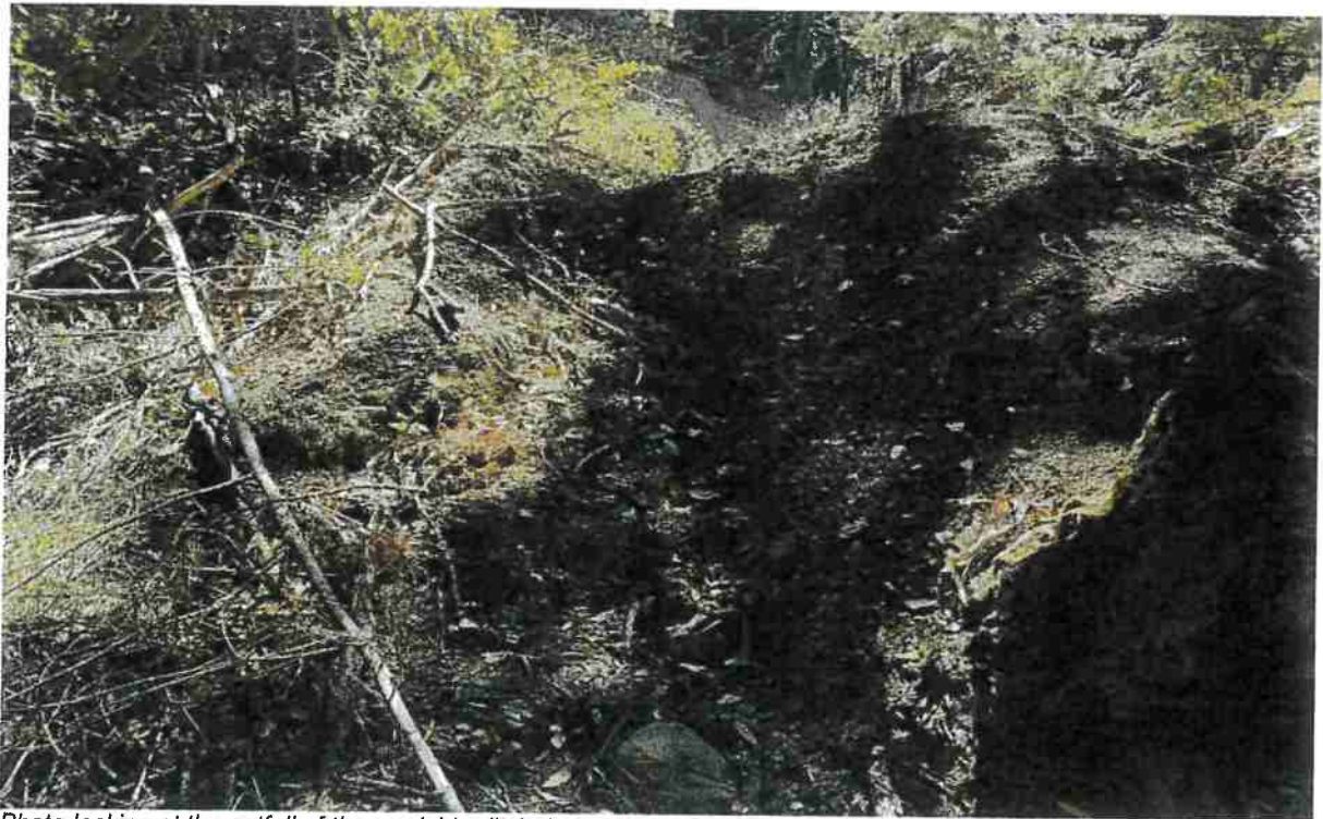
Photo looking at the outfall of the roadside ditch that starts at Site 14 and extends down to Site 13.
