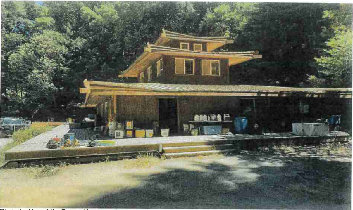
Photo looking at the Drying House on the property.
