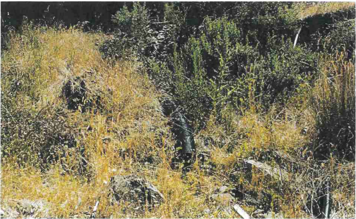
Photo looking at the outlet of the French drain at Site 16.
