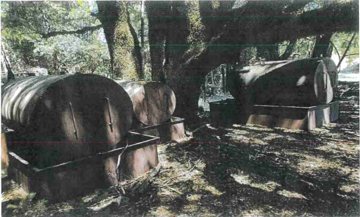
Photos looking at the petroleum tanks that don't have proper cover at Site 21.
