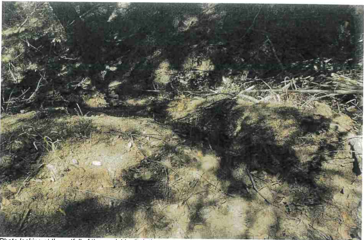
Photo looking at the outfall of the roadside ditch that starts at Site 14 and extends down to Site 13.
