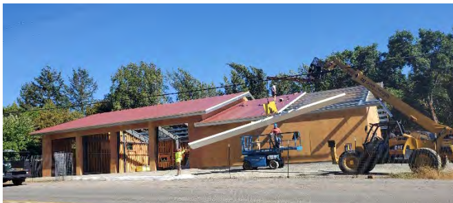
New Briceland Fire Station Under Construction
