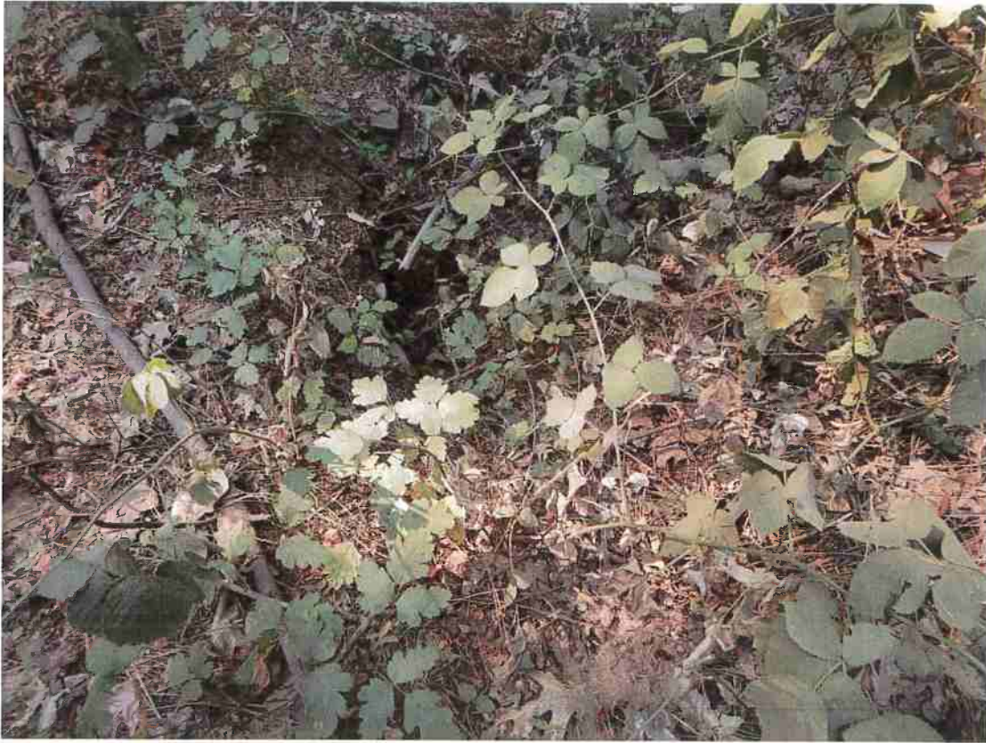
Photo 16: RP 8. Inlet to drainage relieve culvert.
