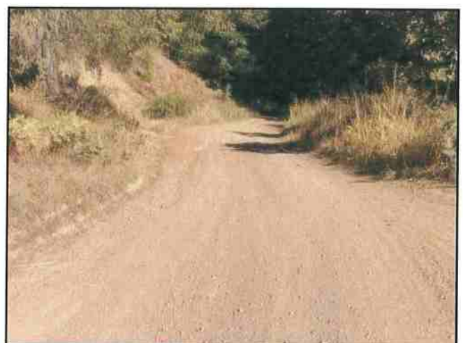
Photo #450 River Rd @ Curve w/ Turnout Looking NW
