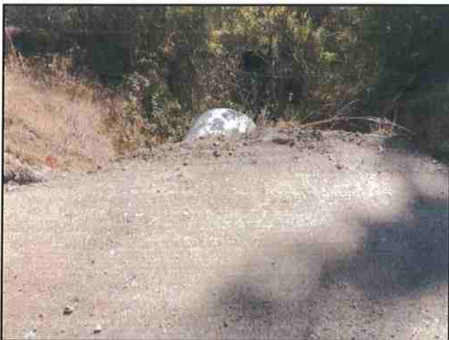
Photo #125 River Rd Looking @ 36" Culvert Out
