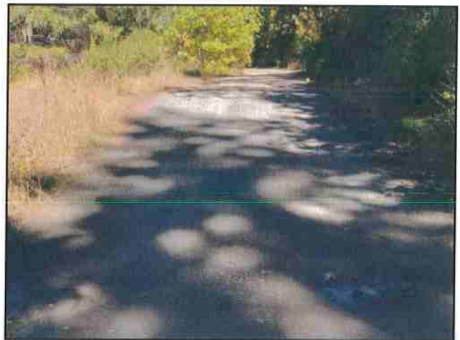
Photo #266 River Rd Looking North @ Turnout Location
