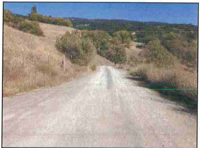
Photo #38 River Rd Looking East
