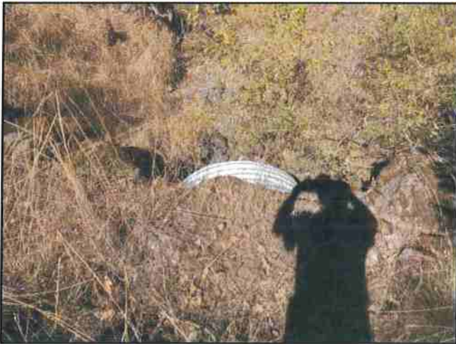
Photo #63 River Rd Looking @ 36" Culvert Out (Dual?)
