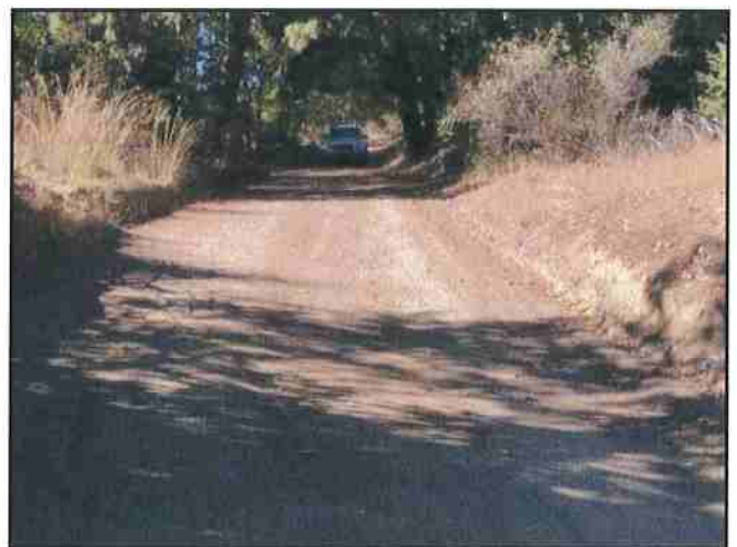
Photo #402 River Rd Looking NE
