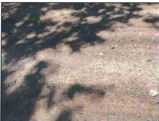
Photo #143 River Rd Looking @ Drainage Path Over Road
