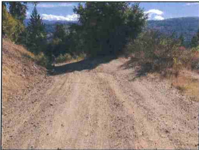
Photo #387 River Rd @ Turnout Location Looking SW @ Curve
