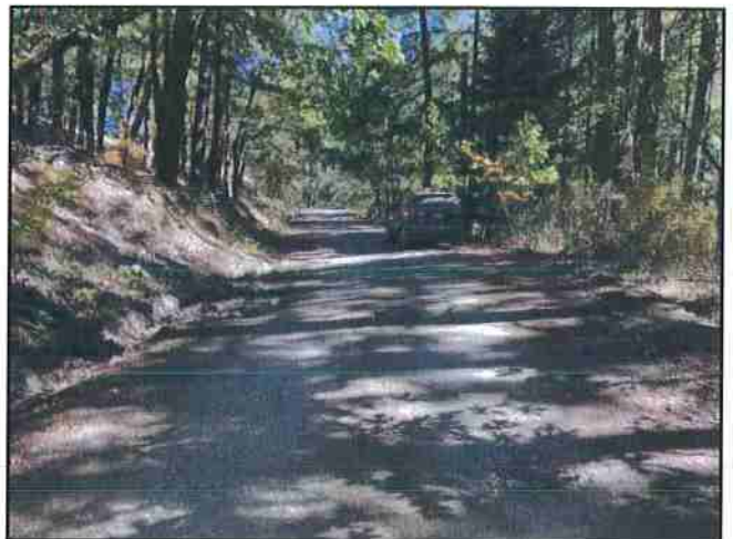
Photo #100 River Rd @ Curve w/ Turnout Looking SE
