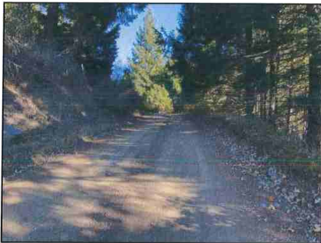
Photo #201 River Rd Looking SE @ Curve w/ Turnout
