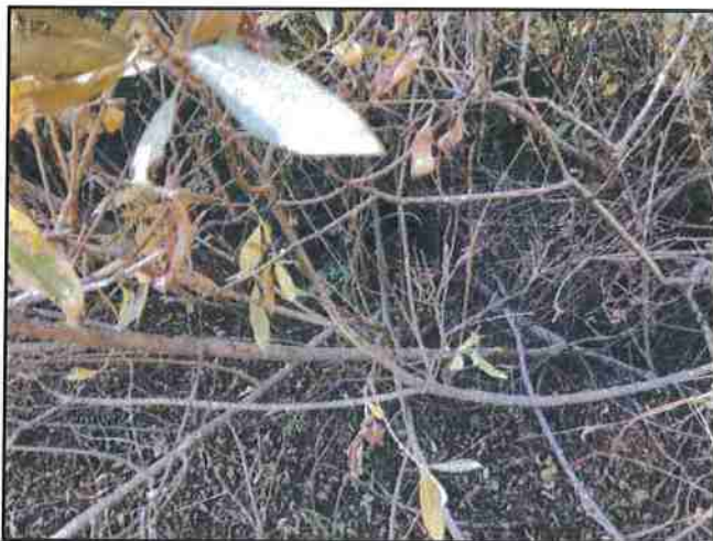
Photo #203 River Rd Looking @ 12" Culvert In
