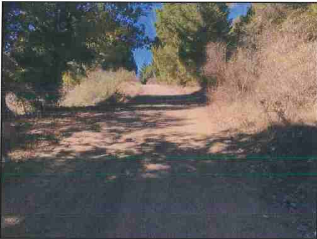
Photo #189 River Rd @ Turnout Looking @ Curve w/ Turnout
