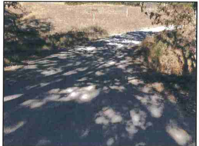
Photo #70 River Rd @ Turnout Looking @ Curve
