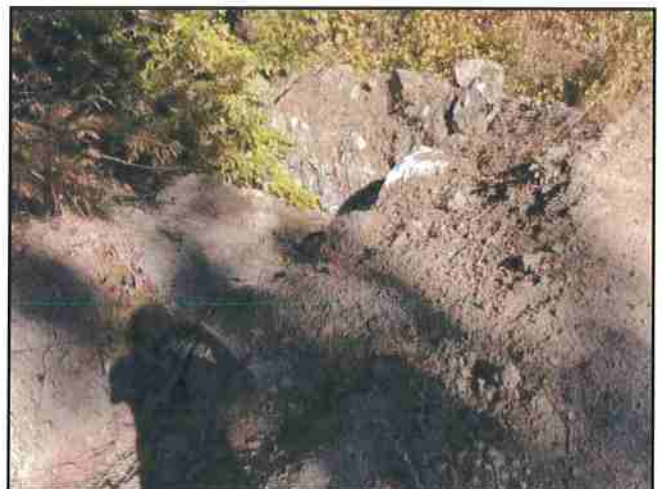
Photo #126 River Rd Looking @ 36" Culvert In
