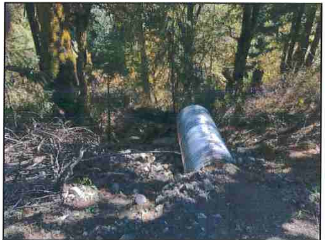
Photo #178 River Rd Looking @ 36" Culvert Out
