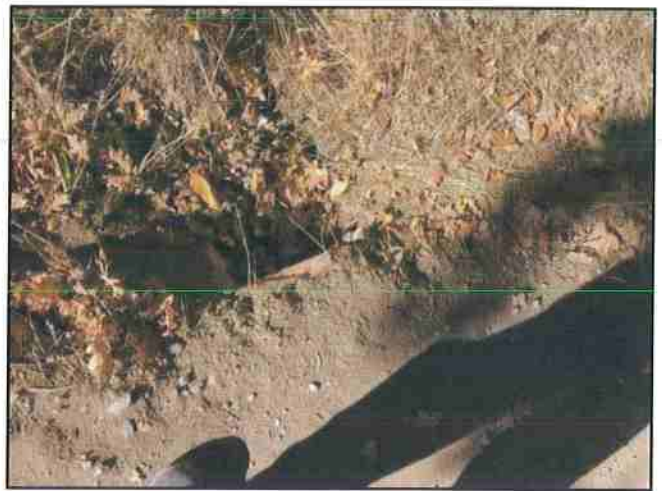
Photo #50 River Rd 12" Culvert In
