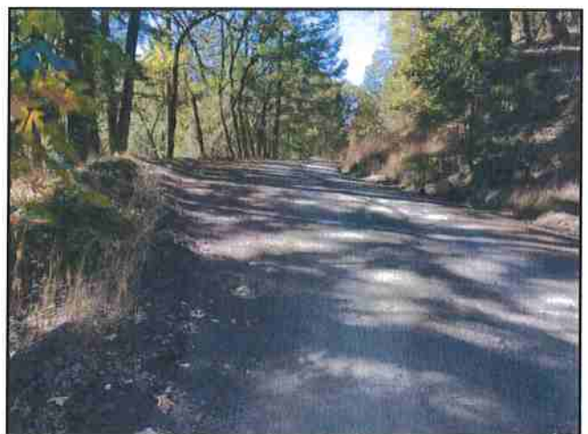
Photo #102 River Rd Looking SE @ Curve w/ Turnout
