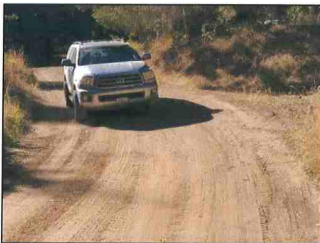
Photo #449 River Rd @ Curve w/ Turnout Looking SW
