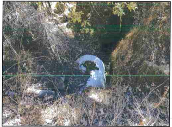
Photo #62 River Rd Looking @ 36" Culvert Out (Dual?)
