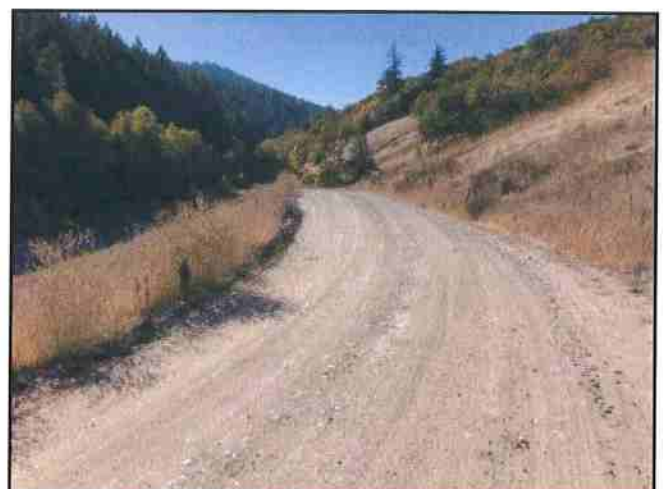
Photo #42 River Rd Looking West @ Curve w/ Pullout
