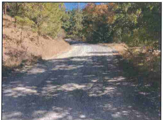
Photo #66 River Rd Looking SE @ Curve w/ Turnout
