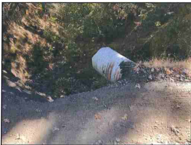
Photo #89 River Rd Looking @ 24" Culvert Out
