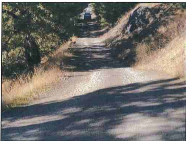
Photo #341 River Rd @ Turnout Location Looking North
