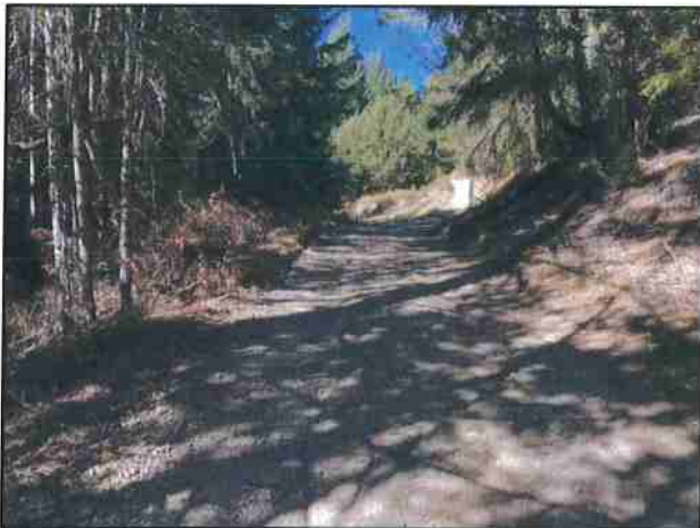
Photo #638 Mad River Trail @ Turnout Location Looking NE @ Curve
