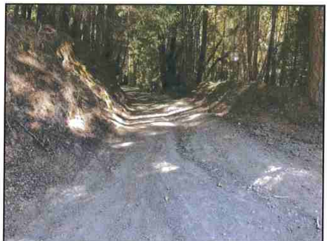
Photo #615 Mad River Trail @ Turnout Location Looking SE @ Curve w/ Rutting (Poor Drainage)
