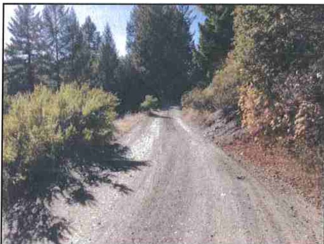
Photo #359 River Rd Looking SW
