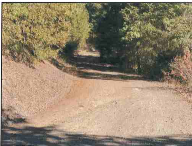
Photo #317 River Rd Looking South @ Curve w/ Turnout
