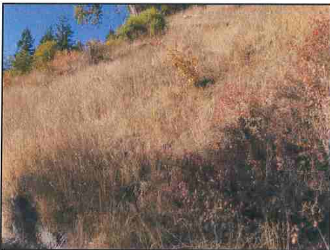
Photo #221 River Rd Looking North @ Hillside Slip
