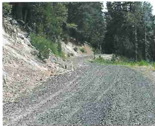
Figure 39. Pinchard Creek road two years after project construction, 2004. Note that the road surface remains in good shape without additional maintenance. Photo: Joe Hoffman, Plumas National Forest.
