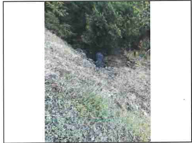
Photo #64 Private Access Rd Looking @ 18" Culvert Out
