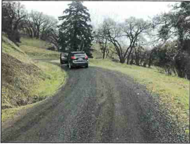
Photo #55 Private Access Rd Looking @ Curve w/ Pullout Looking NE
