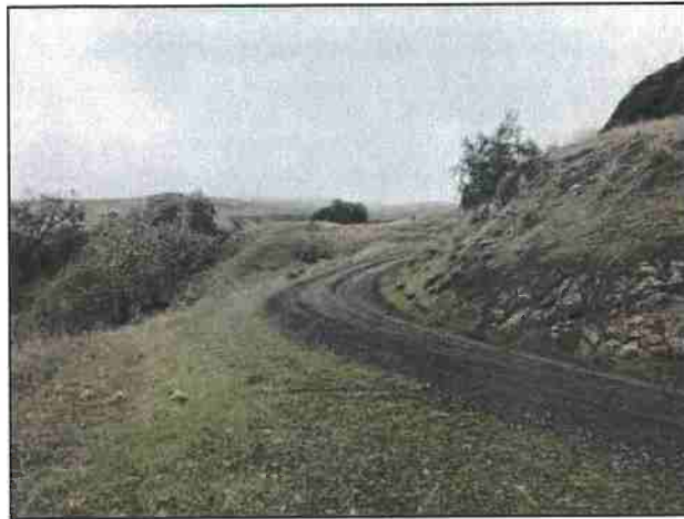
Photo #15 Private Access Rd @ Curve w/ Pullout Looking NW
