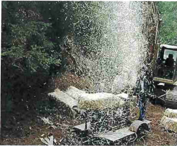
Figure 40. Using a portable blower to spread straw mulch on a disturbed road site. Photo: Julie Bawcom, California Geological Survey.
