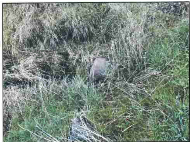
Photo #30 Private Access Rd Looking @ 24" Culvert In
