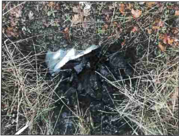
Photo #19 Private Access Rd Looking @ 18" Culvert In
