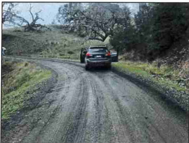
Photo #11 Private Access Rd @ Curve w/ Pullout Looking NW
