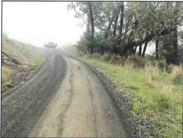
Photo #81 Private Access Rd @ Curve w/ Pullout Looking NE
