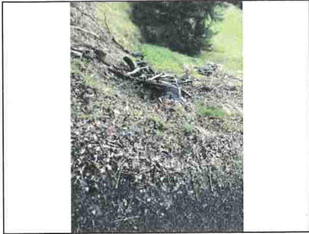
Photo #49 Private Access Rd Looking @ 12" Culvert Out
