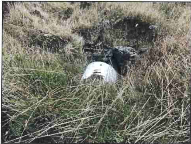
Photo #21 Private Access Rd Looking @ 18" Culvert Out
