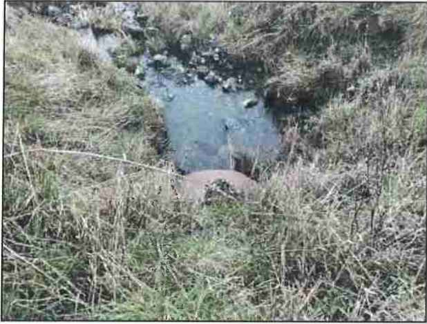
Photo #31 Private Access Rd Looking @ 24" Culvert Out
