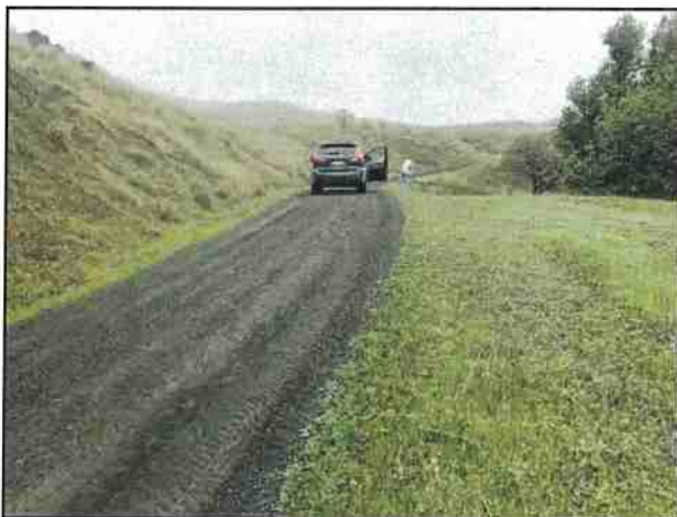
Photo #59 Private Access Rd Looking @ Curve w/ Pullout Looking NE
