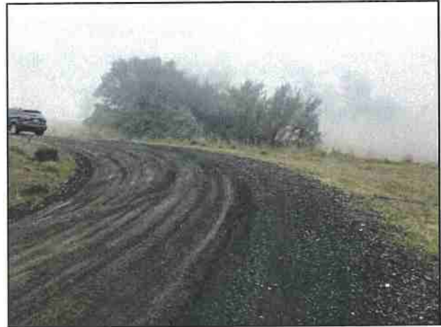
Photo #88 Private Access Rd @ Curve w/ Pullout Looking NE
