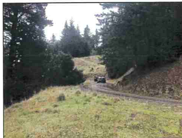
Photo #5 Private Access Rd @ Curve w/ Pullout Looking NE
