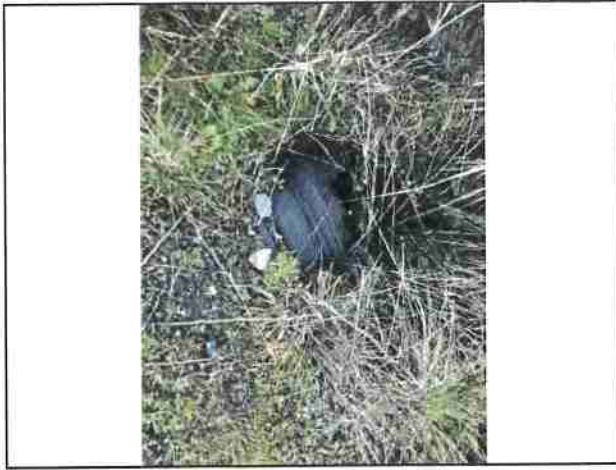
Photo #25 Private Access Rd Looking @ 18" Culvert In
