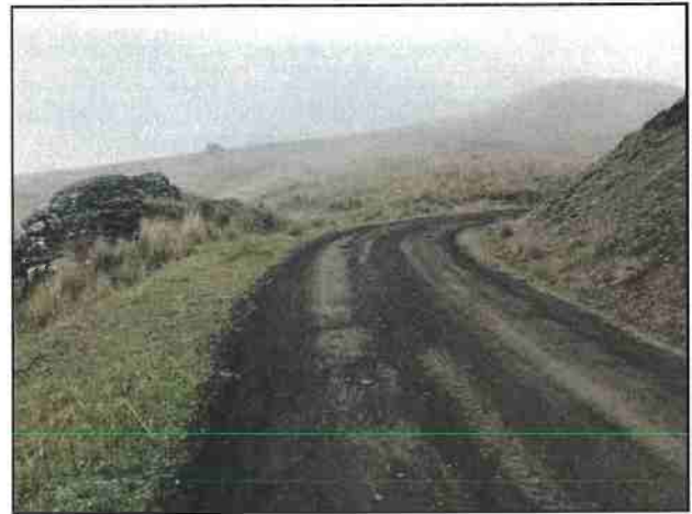
Photo #76 Private Access Rd @ Curve w/ Pullout Looking NW
