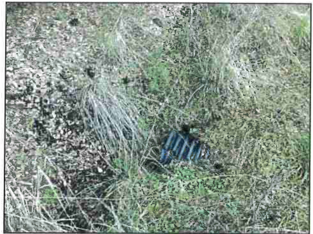
Photo #8 Private Access Rd Looking @ 18" Culvert In
