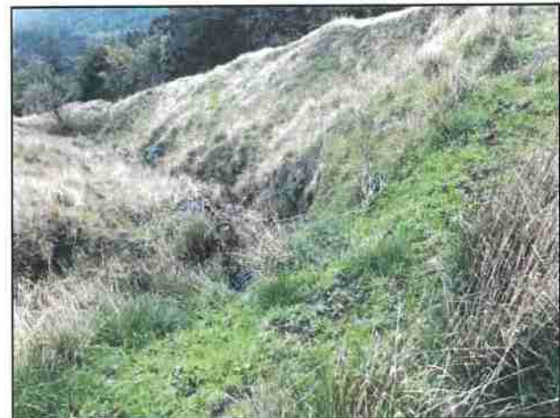
Photo #66 Private Access Rd Looking @ 18" Culvert Out
