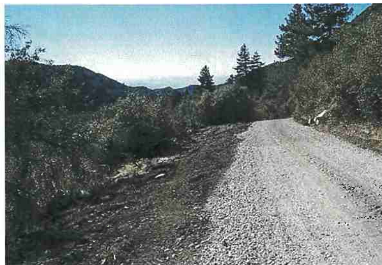
Figure 1. Low-volume road that has been newly graded and out-sloped, San Bernardino County. Photo: Richard Harris.
