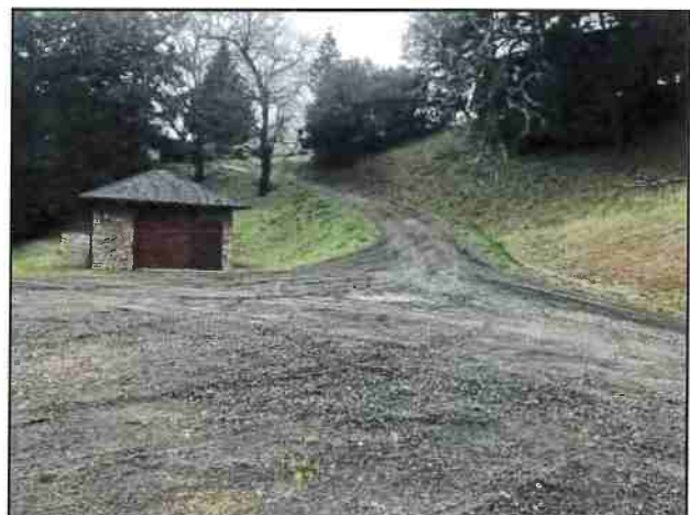
Photo #120 Private Access Rd @ Turnaround Looking NE
