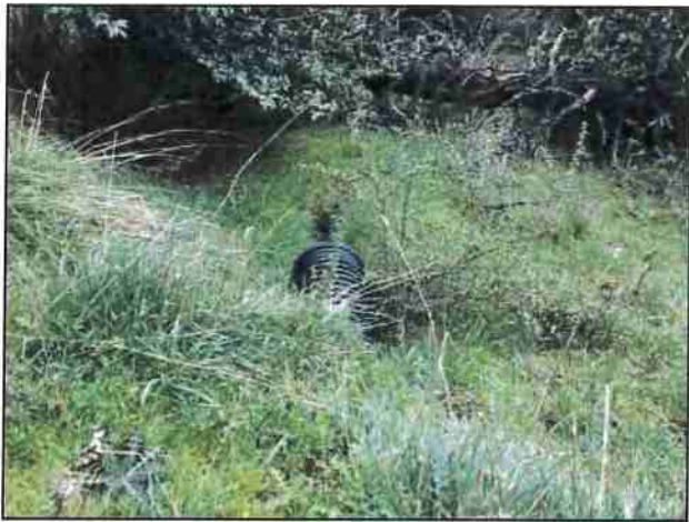
Photo #9 Private Access Rd Looking @ 18" Culvert Out
