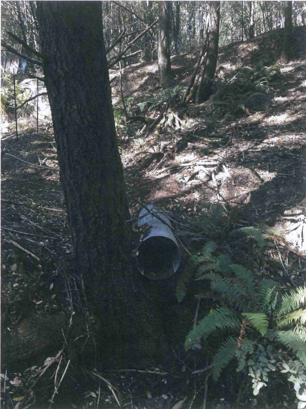
Picture 11: Outlet of Crossing #3. Photo date 8-13-2019
