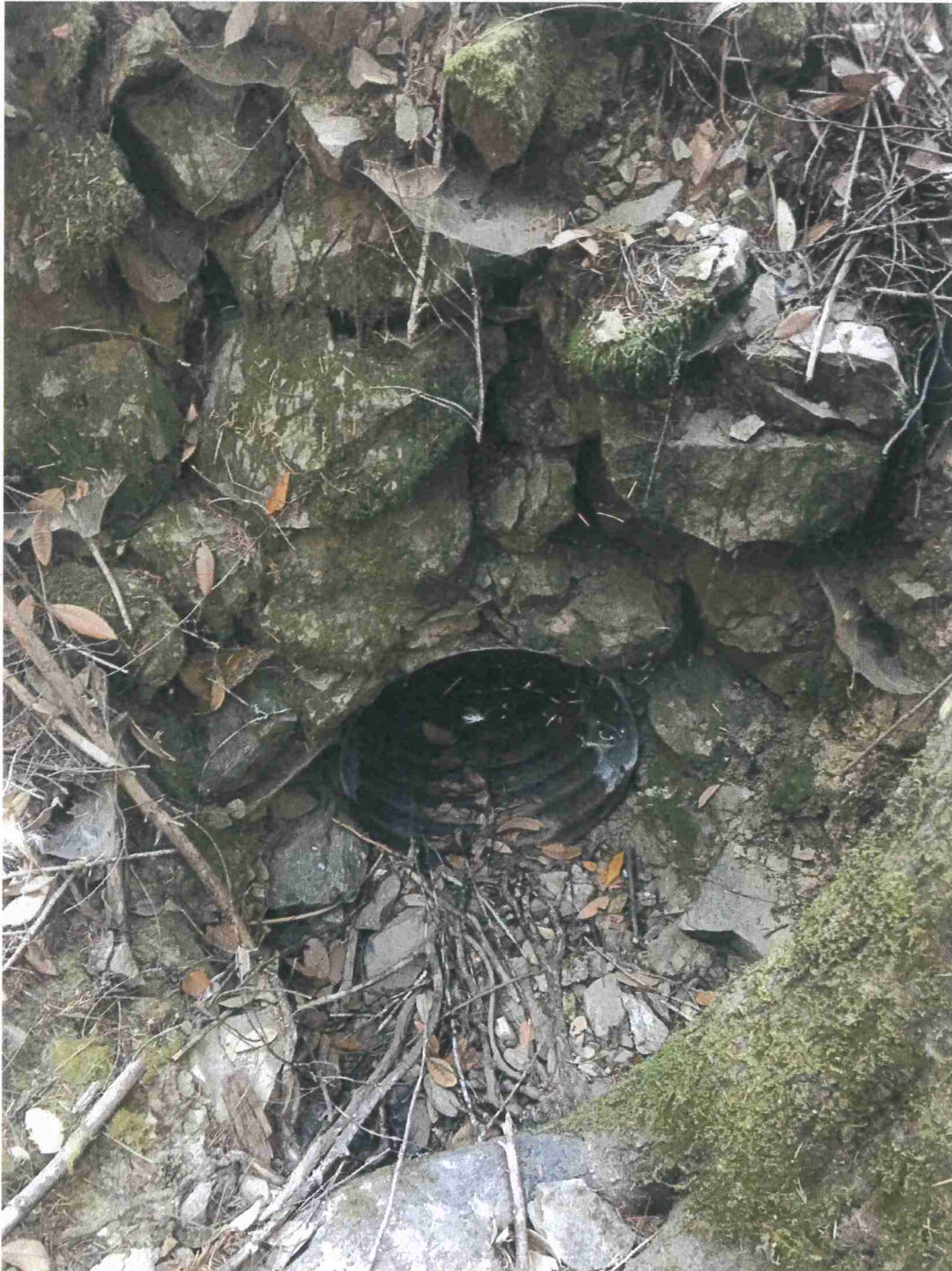
Picture 10: Inlet of Crossing #3. Photo date 8-13-2019
