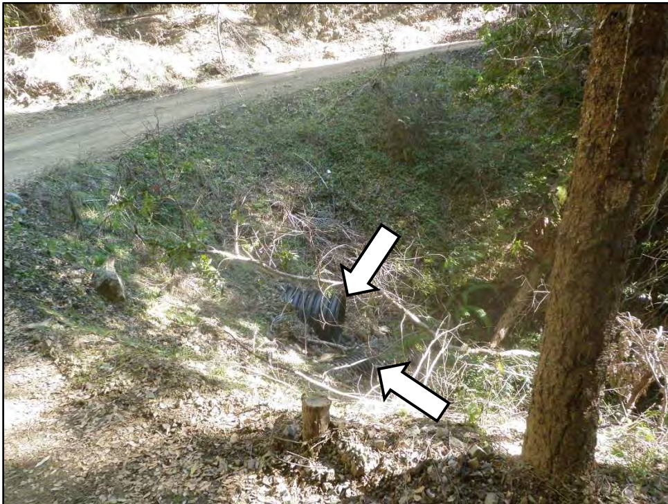
Photo 12 – Project #6, View from right road looking at SC #5 (lower arrow) culvert outlet, set at the base of fill. Note the upper arrow shows disclosure point SC #4 culvert outlet, also set at the base of fill.
