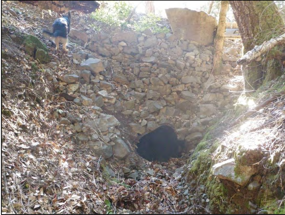
Photo 17 – Project #9, View looking downstream at SC #9 culvert inlet.
