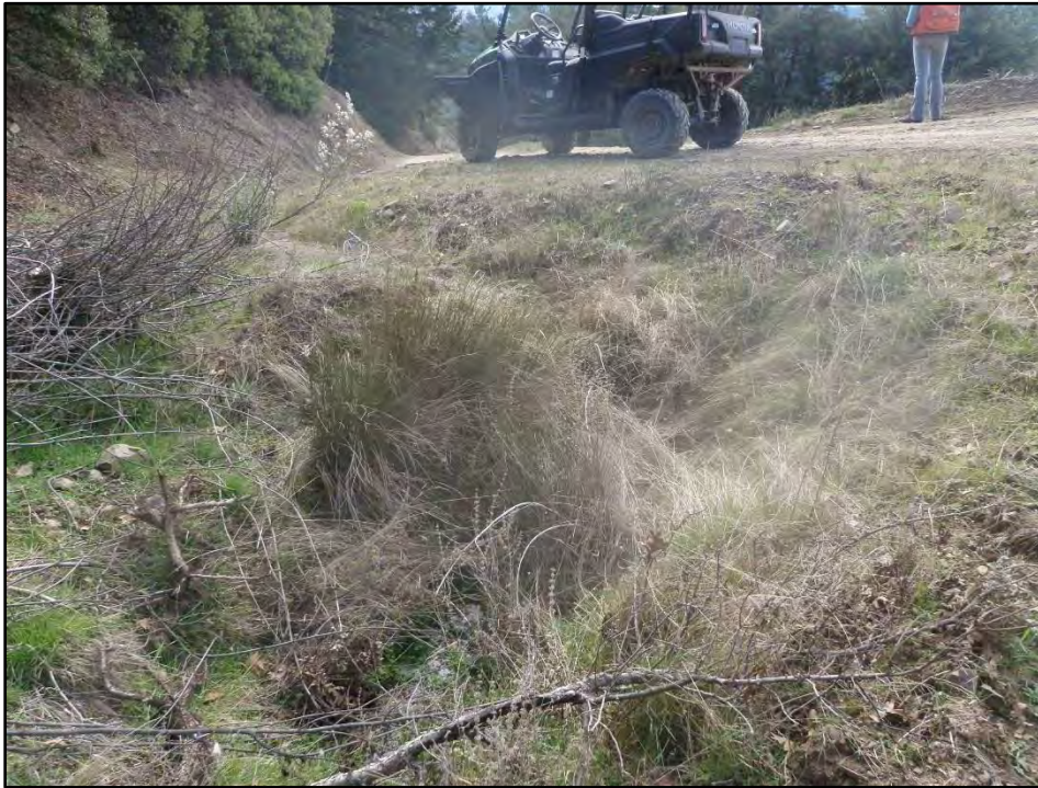
Photo 4 – Project #2, View of Stream Crossing (SC) #1 looking downstream towards the culvert inlet.
