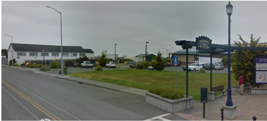
Figure 2: Street view from Waterfront Drive and C Street looking northwest
