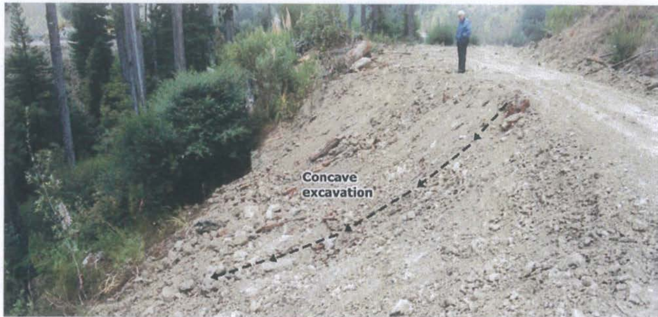
FIGURE 230. The most cost-effective treatment for unstable fills along the outside of a forest, ranch or rural road is simply the direct excavation of the unstable material. If road width is too narrow, additional width can often be derived from cutting into the bank. The excavation should encompass the unstable fill materials, beginning at the inside crack or scarp, and extending out and down the fill slope as far as possible. For proper surface drainage, and to retrieve most of the unstable fill, the excavation should have a concave profile when completed. Typically, the bulk of the fill is within 20 to 25 feet of the outside edge of the road and is easily reached by a mid-sized excavator. Any remaining fill is likely to be small enough that it will not fail or travel far enough to reach the stream.
