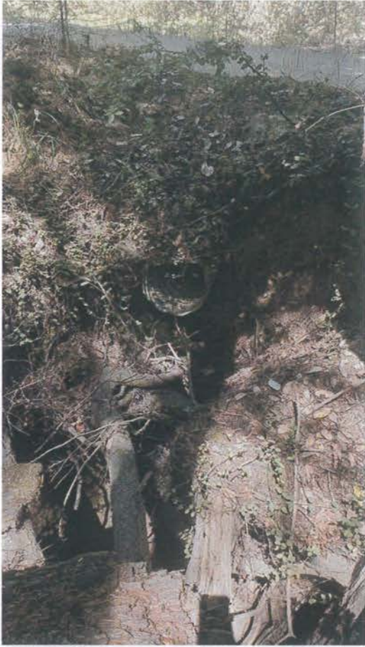
Site 24. Outlet of the watercourse crossing.
