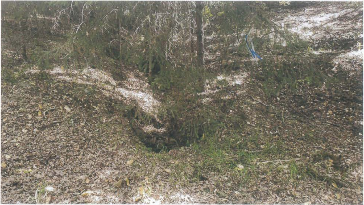
Inlet of the watercourse crossing at Site 17.
