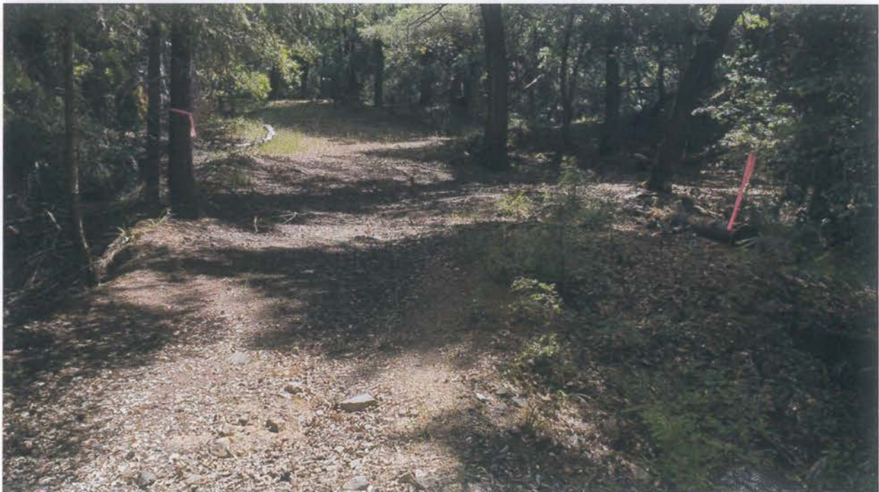
Site 19. Approximate location of watercourse re-alignment. A waterbar (Site 18) will be installed further up grade from the re-aligned watercourse.
