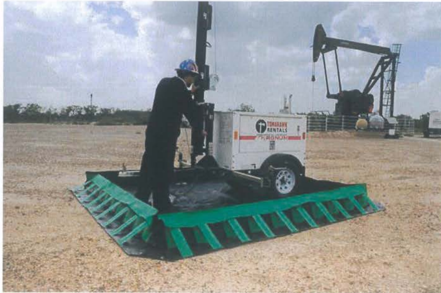
Example of a small, portable, and compact containment berm.
