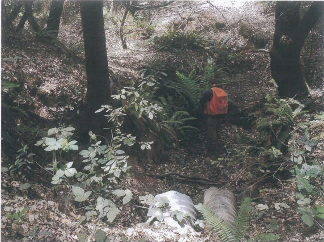
Site 23. Looking down channel from the outlet. The upgraded culvert will outlet approximately where the blue flag is being hung.
