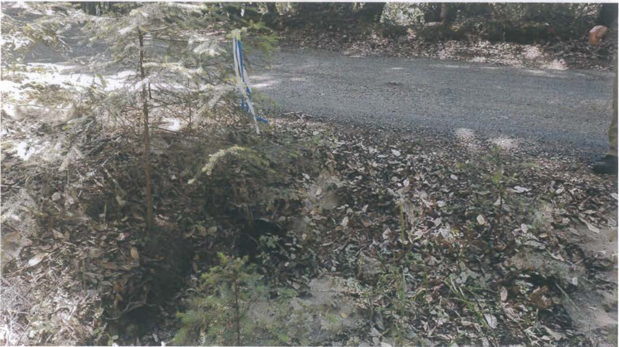
Site 24. Inlet of the watercourse crossing.
