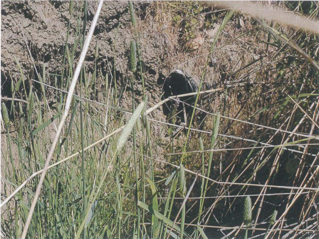
Site 04. Looking at the outlet.
