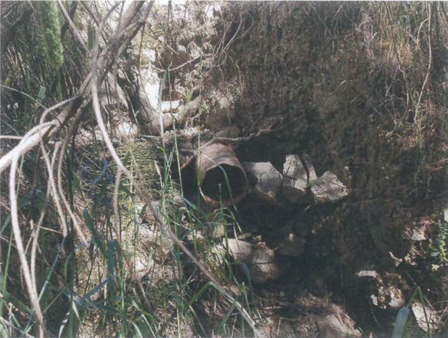
Site 07. Looking at the outlet.
