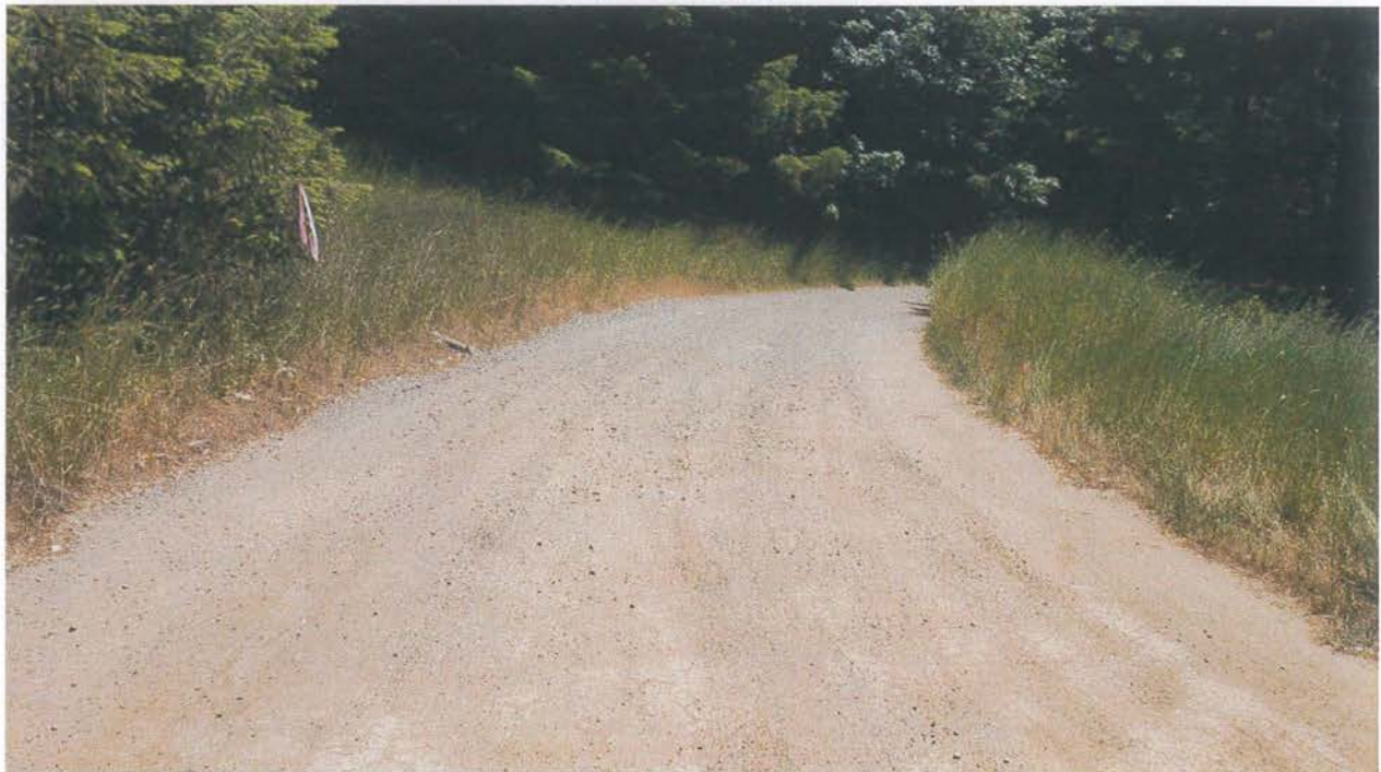
Site 12. Hydrologic disconnect for Sites 13, 14, and 23.
