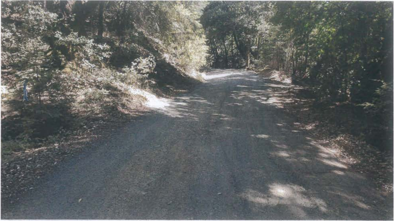
Site 24. Looking down grade.
