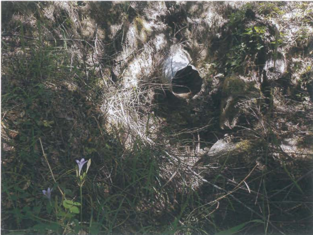
Site 05. Looking at the outlet.
