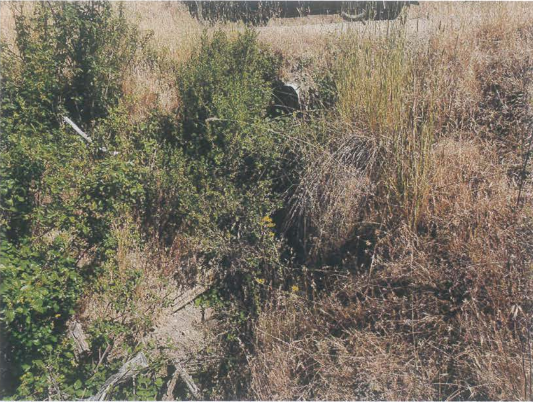
Site 03. Looking at the outlet.
