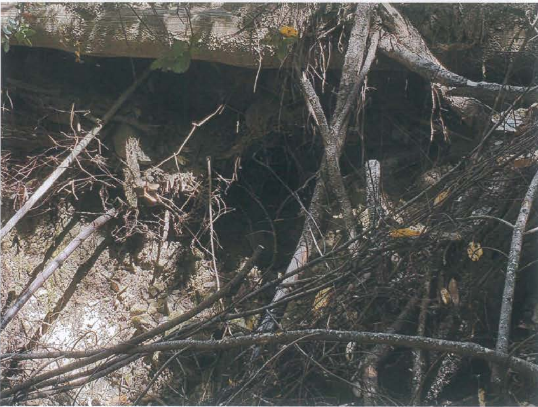
Site 06. Looking at the outlet.
