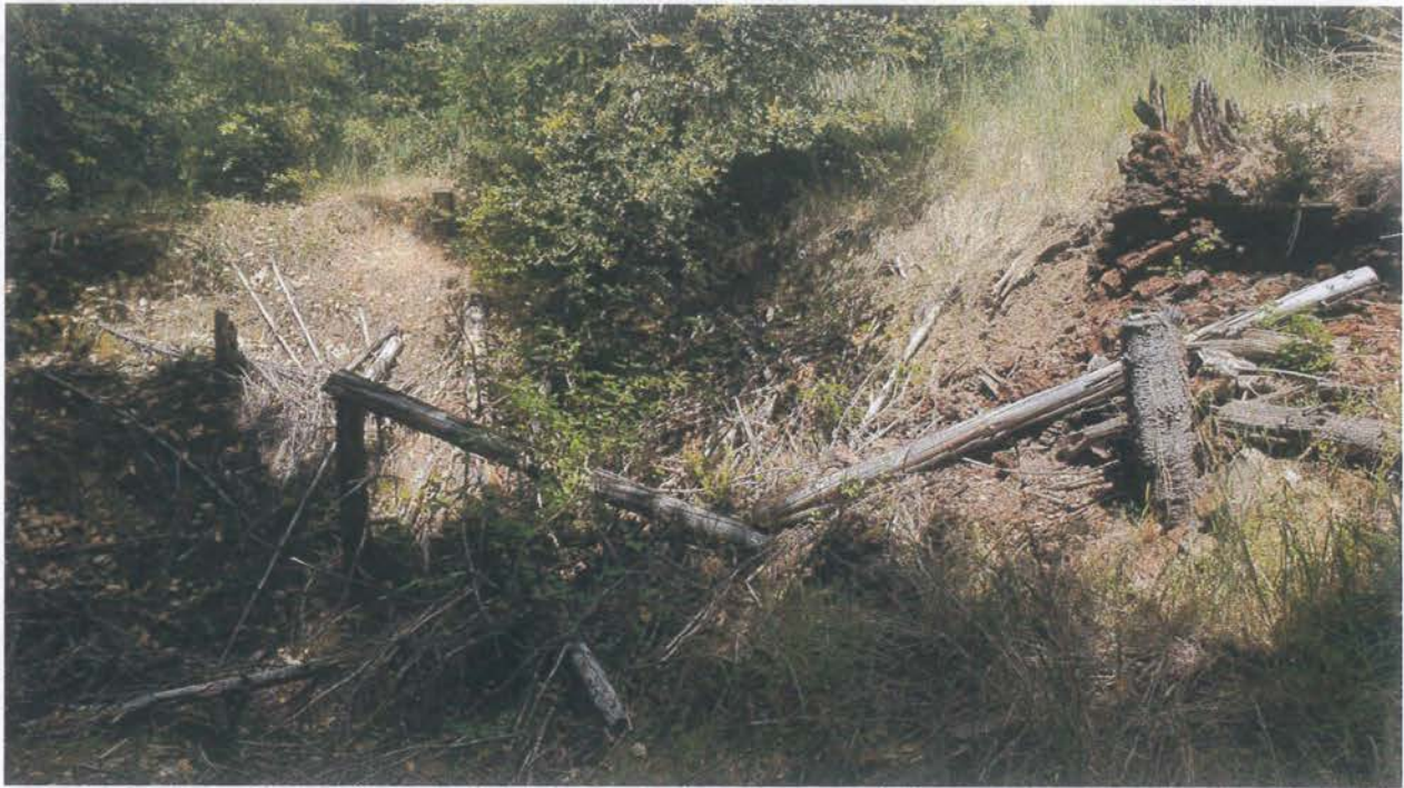
Site 19. Photo of the southeastern embankment of G5/G6/G, immediately downstream of the outlet of the watercourse crossing at Site 19. Note vegetation and rotted trees in the upper right. Indicative that this location has been in this condition for many years and was not recently created.
