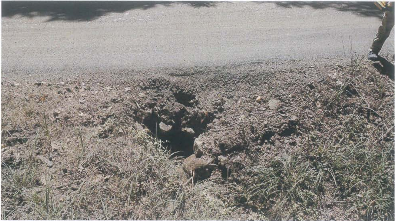
Site 26. Inlet of the watercourse crossing.
