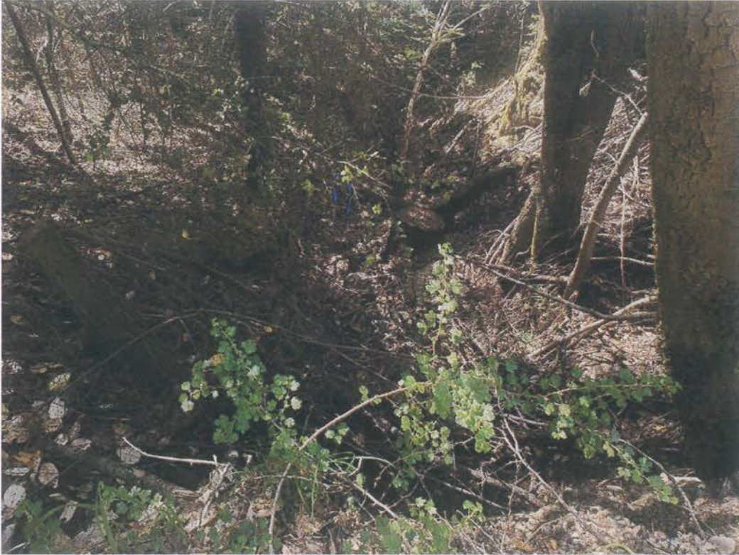
Site 06. Looking down-channel from the outlet. The upgraded culvert will outlet approximately where the blue flagging is hanging.
