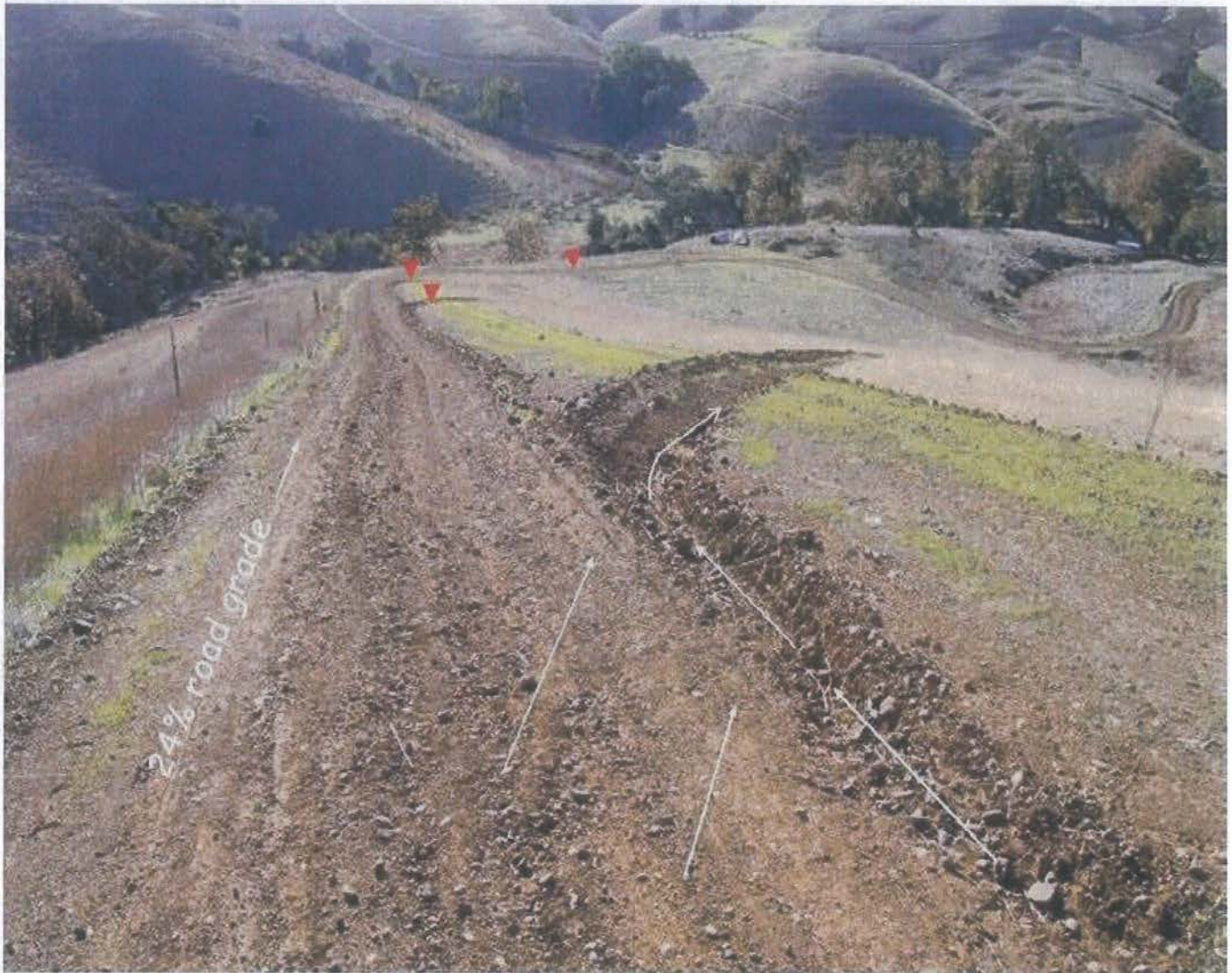
FIGURE 55. Steep roads that go straight up or down a hillside are very difficult to drain. This steep, fall line road developed a through cut cross section that was drained using lead out ditches to direct runoff off the road and onto the adjacent, vegetated hillside. The road was "outsloped" to drain runoff to the right side, and the lead out ditch was built slightly steeper than the road grade, to be self-cleaning. Four lead out ditches have been constructed at 100-foot intervals to the bottom of the hillside.
