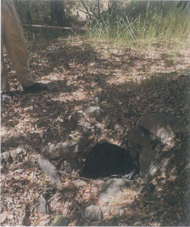
Inlet of Site 19
