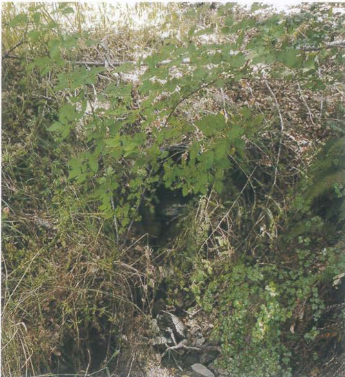
Site 19. Looking at the outlet.
