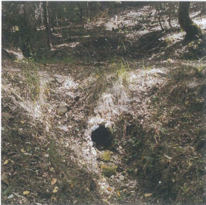
Outlet of the watercourse crossing at Site 17
