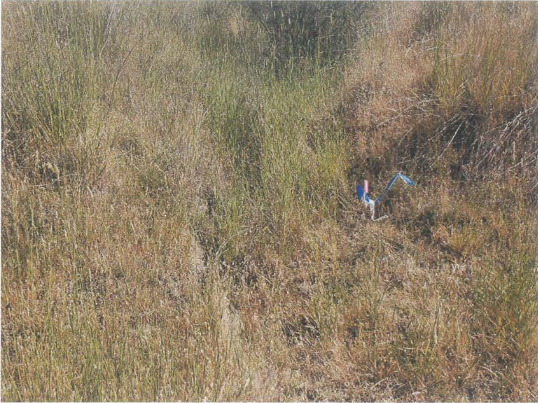
Site 08. Looking up-channel from the inlet of the culvert.
