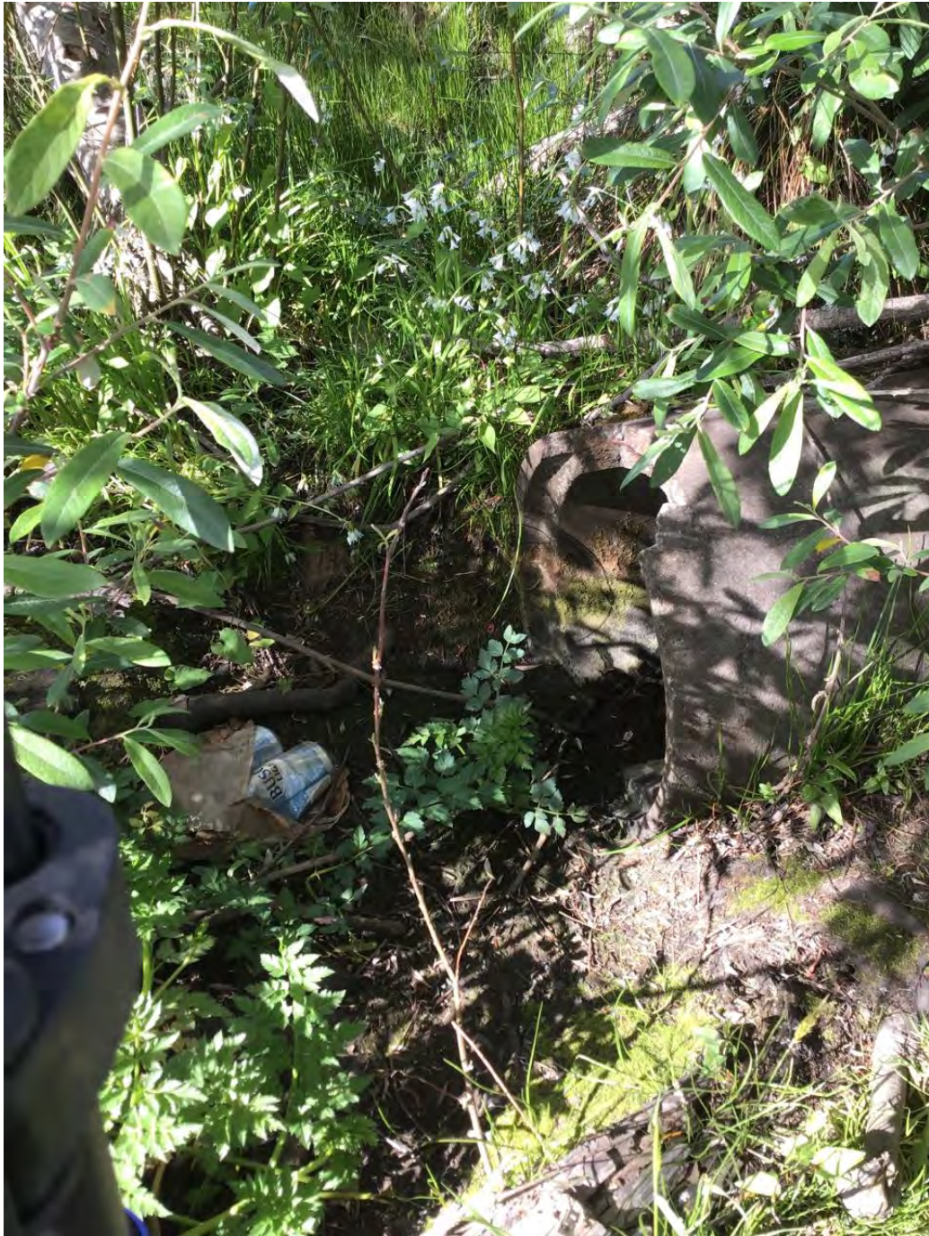
Photo 4. Downstream culvert within Wetland 4 (5/11/2021).
