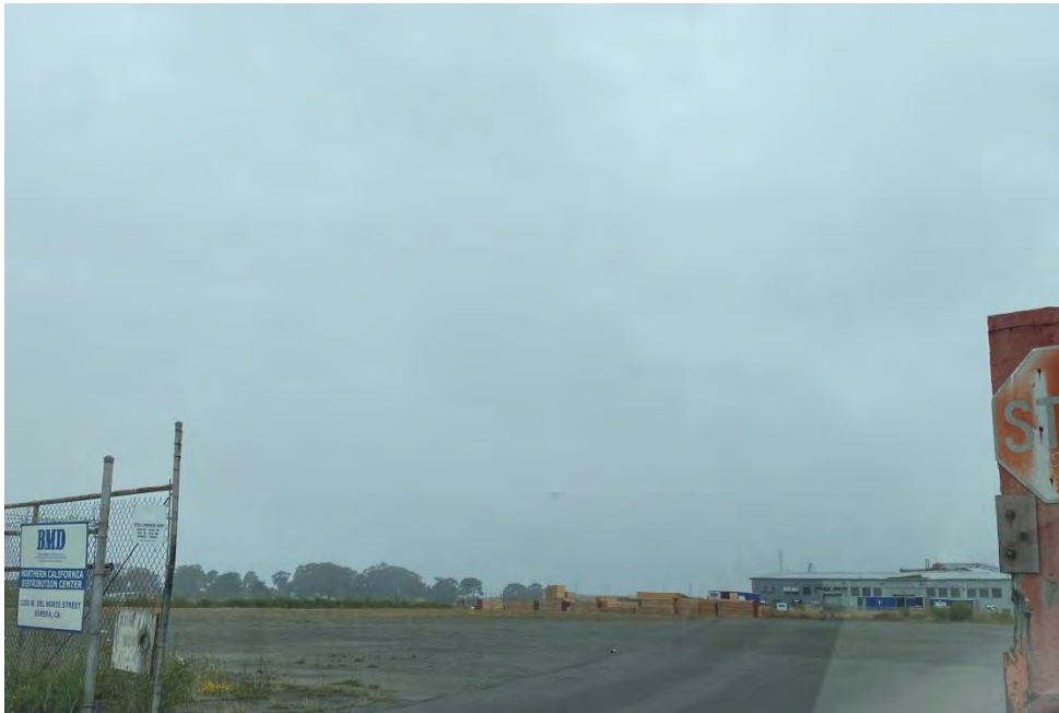
Photo 9 - View facing north, Project's staging area north of the Del Norte Street Pier in Eureka.
