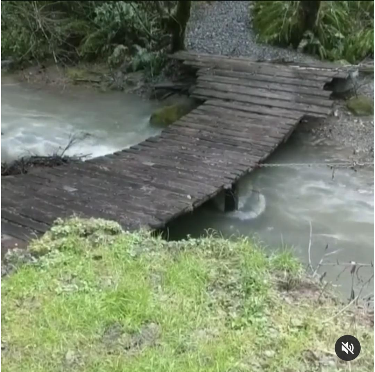
Figure 3. Bridge we are requesting to repair in it's current state, pictured here with the creek at it's highest flow. Fish and game has said that it's current height is not enough to allow down wood to pass through at high tides
