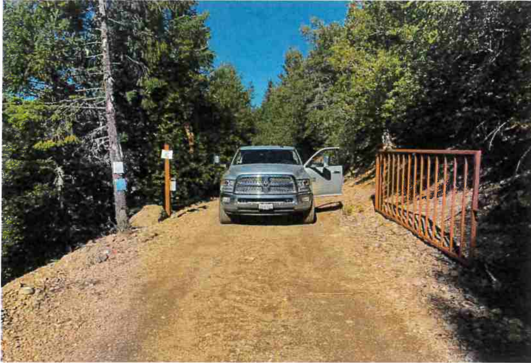
Figure 1: RP 1 on Supply Creek Rd. (Section scheduled for repair & maintenance - To start by 6/1/2020)
