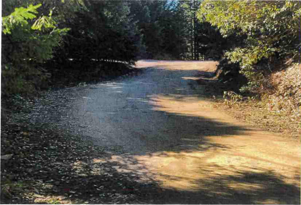
Figure 32: RP 19 on Old 3 Creeks Rd.
