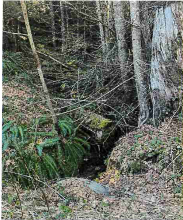
Figure 5: RP 4 on Supply Creek Rd.
