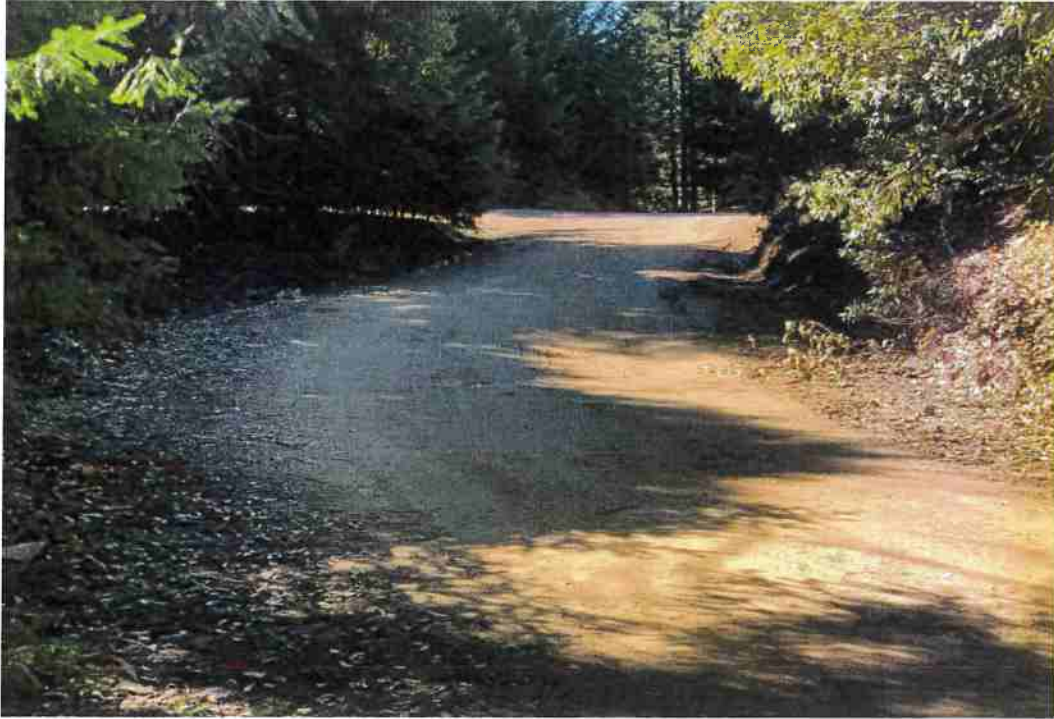
Figure 32: RP 23 on Old 3 Creeks Rd.
