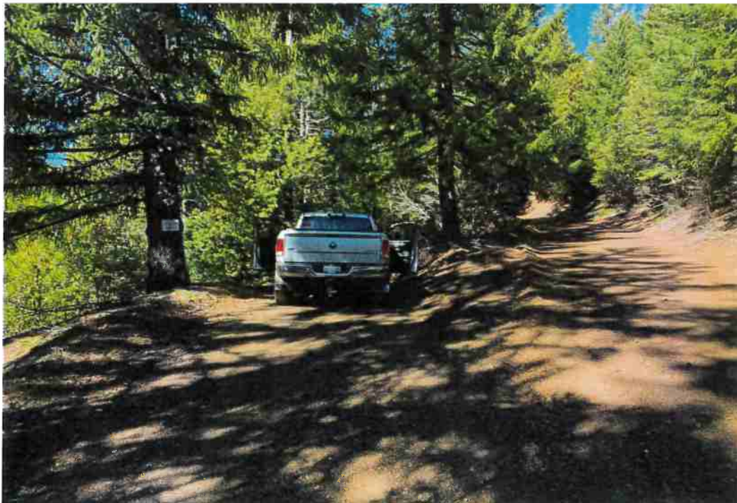
Figure 2: RP 2 on Supply Creek Rd. (Section scheduled for repair & maintenance - To start by 6/1/2020)
