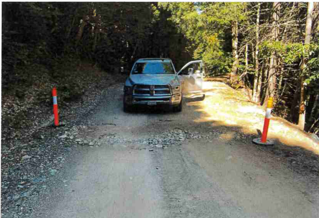
Figure 25: RP 22 on Old 3 Creeks Rd.
