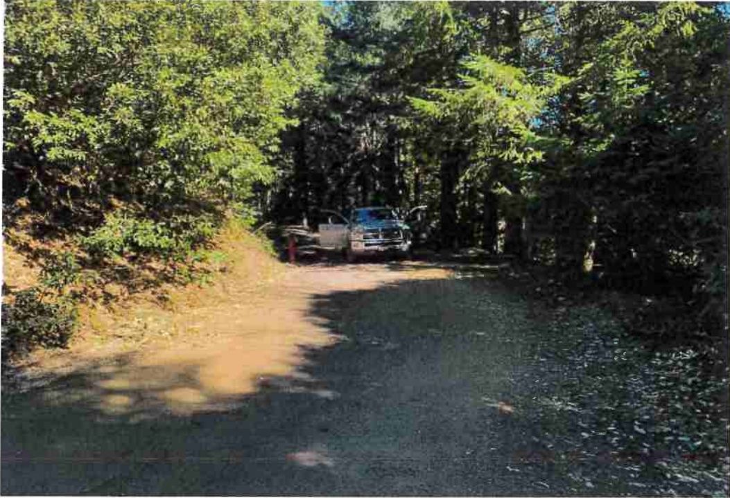
Figure 30: RP 19 on Old 3 Creeks Rd.
