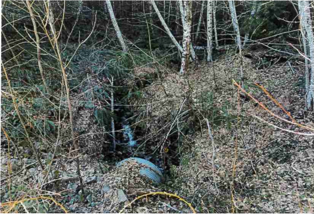
Figure 9: RP 6 on Supply Creek Rd.
