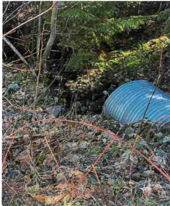
Figure 4: RP 4 on Supply Creek Rd.
