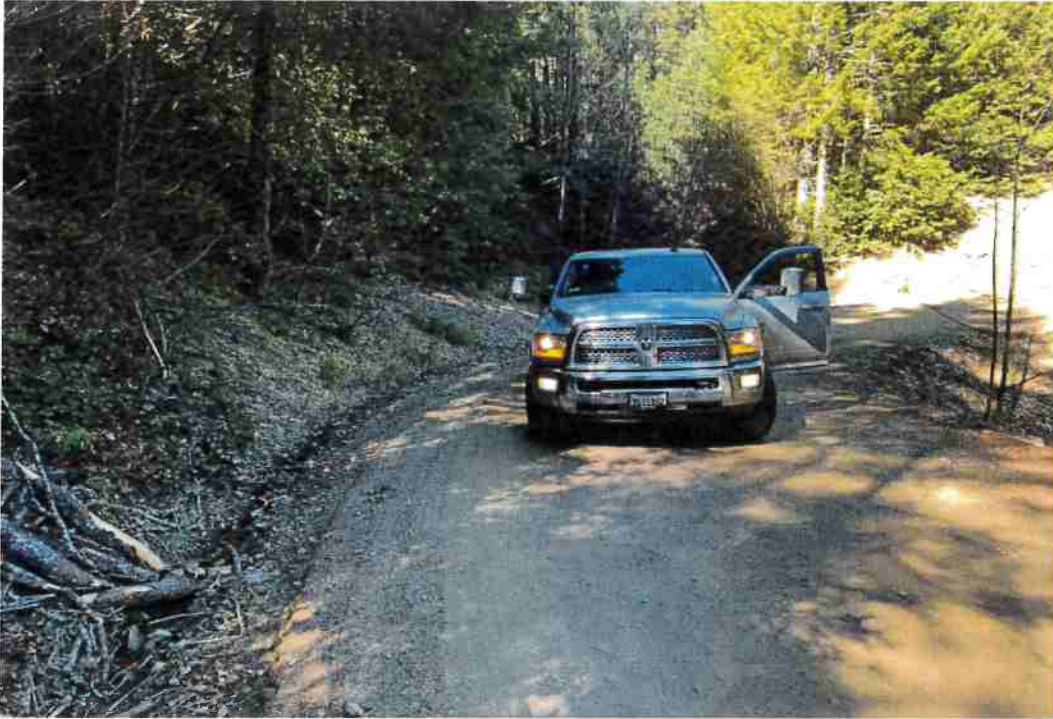
Figure 22: RP 19 on Old 3 Creeks Rd.
