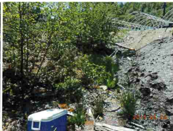
Fig. 2. Fillslope and soil encroaching on riparian vegetation
