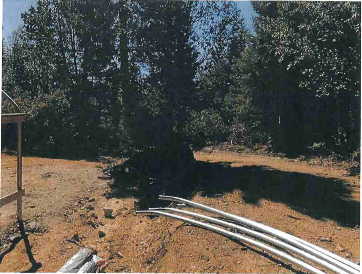
Photo #1 : This is an image of the southern extent of Cultivation Area #6 (CA 6), where surface runoff is hydrologically connected to surface waters. The Discharger shall install a pipe at this location that channels the runoff beneath the road at the top right of the image, where it can disperse and infiltrate in the vegetation. Photo Date: 06/06/2017.
