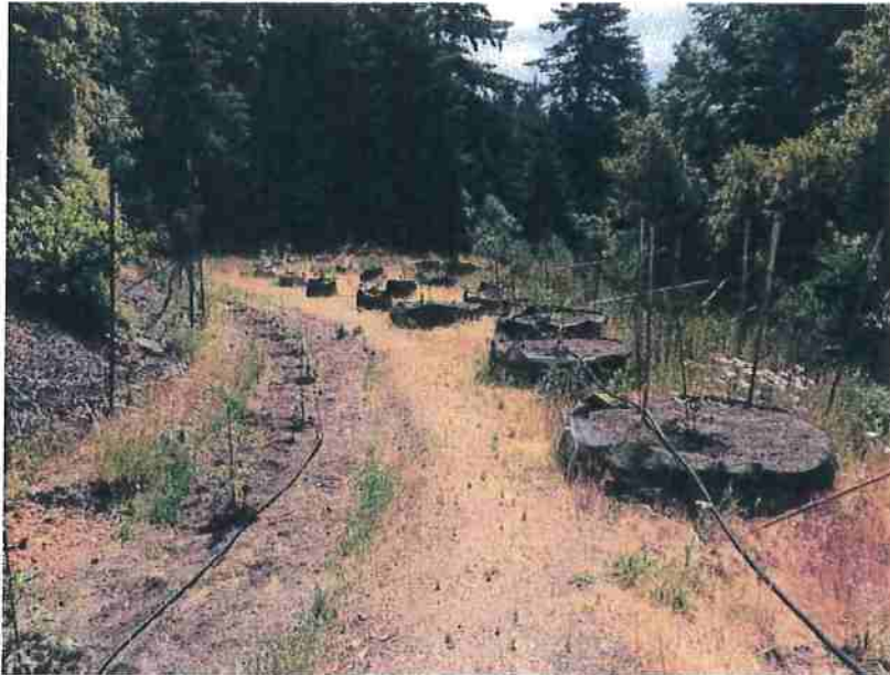
Photo 3-5A: Spent potting soil and cultivation-related materials located at Cultivation Area #5 (CA #5). View is from the right road approach looking southeast toward the outboard fillslope landslide. (Photo taken June 13, 2016)
