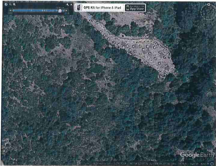
Photo 5-1C: 2014 Google Earth aerial imagery pre-outboard landing fillslope failure.
