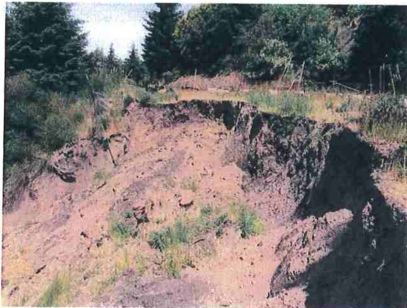
Photo 1-5B: Outboard landing fillslope failure looking northwest from the left edge of head scarp. (Photo taken June 13, 2016).
