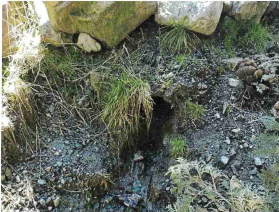
6" culvert currently functional
