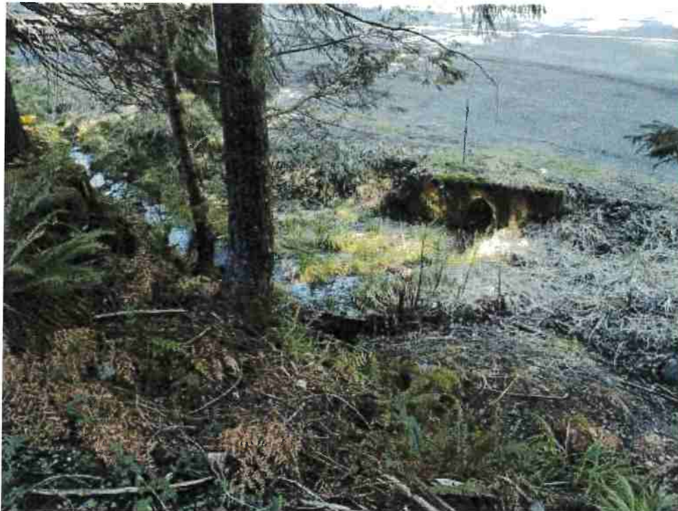
Highway 299 culvert below MP21 where flow should be directed
