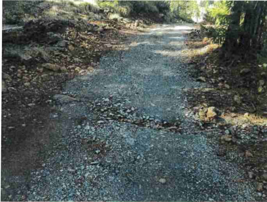
Existing ford, still functional
