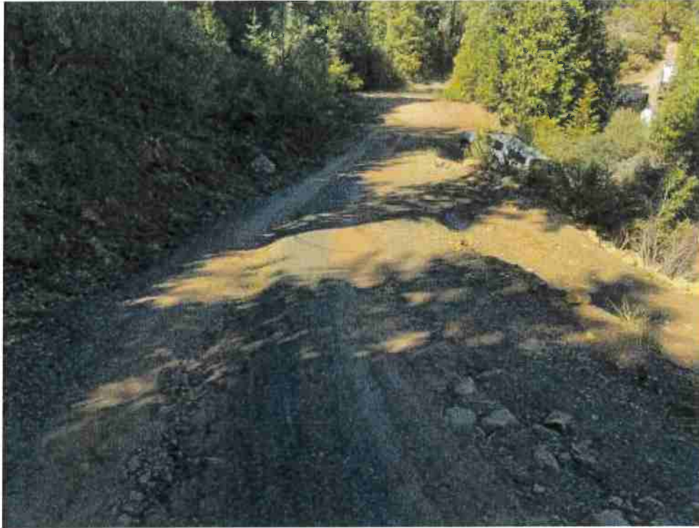
Water diverted to inboard ditch to rolling dip below. Minimal erosion
