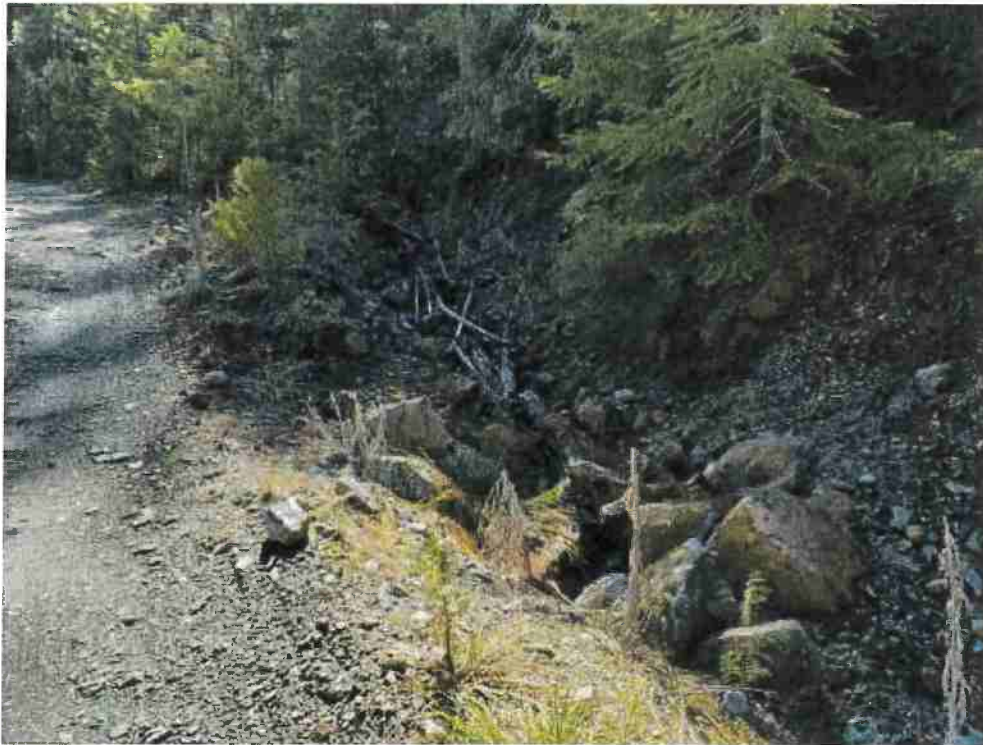
Stream diverted to inboard ditch leading to MP7
