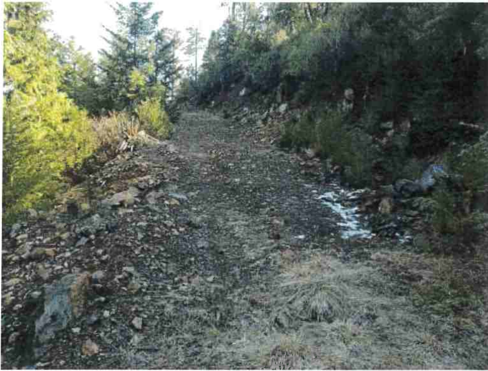
No signs of overtopping above culvert
